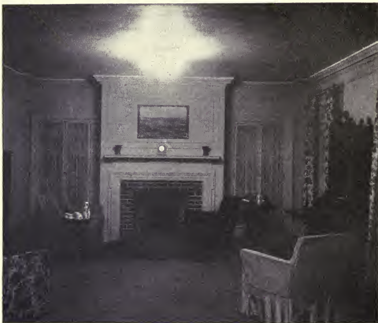
FIG. 49.—Early lighting installation with its glaring ceiling fixture. Compare with modern lighting methods shown in Fig. 50
