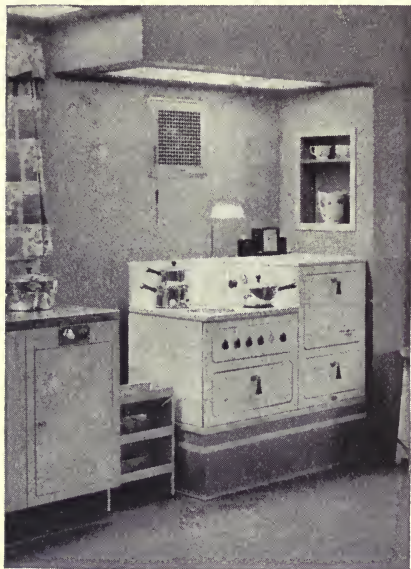
FIG. 62.—Architectural lighting applied to the kitchen. (Installed in ceiling over range)
