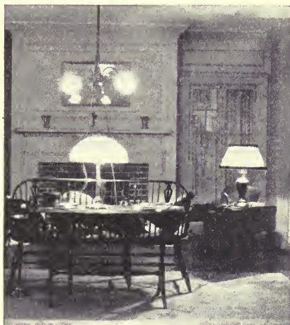
FIG. 84.—Extension cords from ceiling fixture to table lamps are unnecessary when proper wall outlets are used
