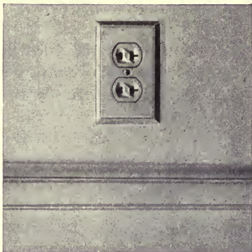
FIG. 15.—The duplex outlet for additional service
