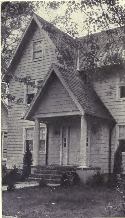
FIG. 52.—Side brackets used for entrance lighting
