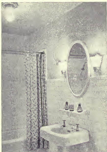
FIG. 66.—Bathroom lighting with both ceiling and side fixtures
