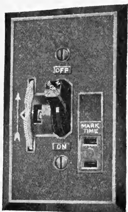
FIG. 182.—Combination time switch for permanent installation
