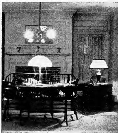
FIG. 84.—Extension cords from ceiling fixture to table lamps are unnecessary when proper wall outlets are used
