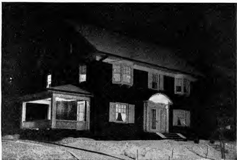
FIG. 53.—Entrance lighting using overhead fixtures
