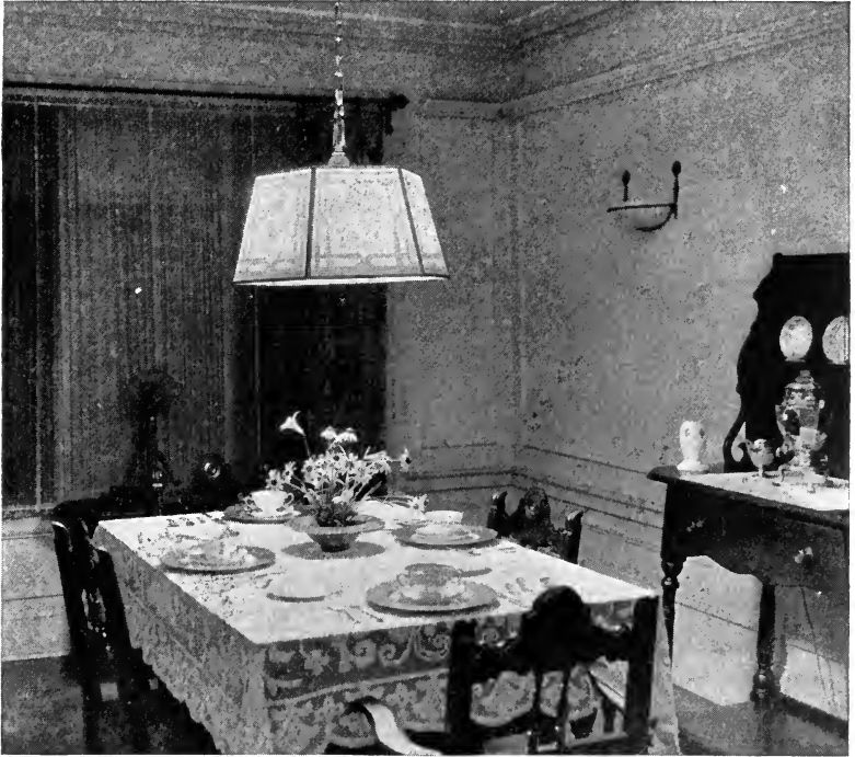
FIG. 58.—Modern dome light for lighting the dining room
