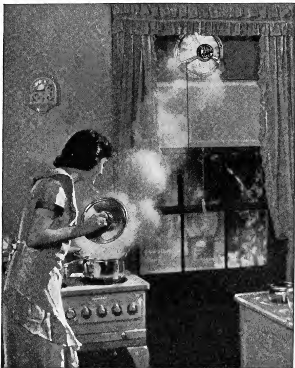
FIG. 20.—A ventilating fan in the kitchen removes cooking odors
