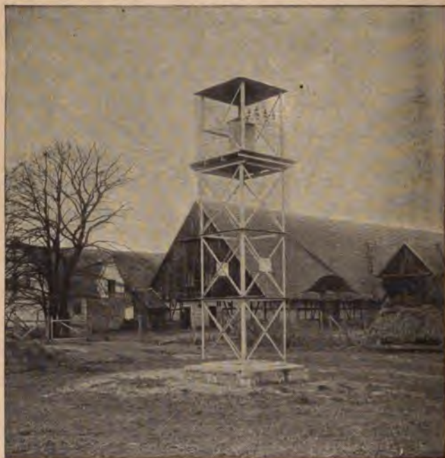
Fig. 2. Electric transformers in the farmyard.
