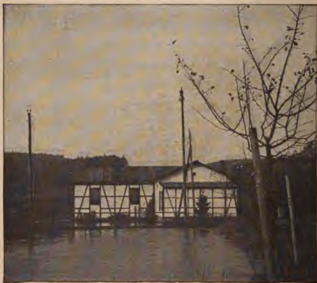
Fig. 4. Hydroelectric generating plant on a large farm.
