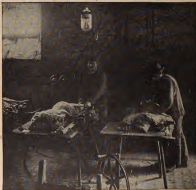
Fig. 38. Shearing sheep by electric power.
