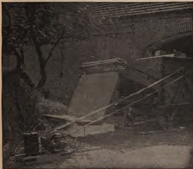
Fig. 16. Portable motor and controller operating thresher.
