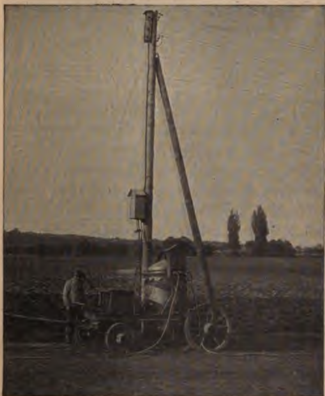
Fig. 8. Portable transformer and field telephone connection.
