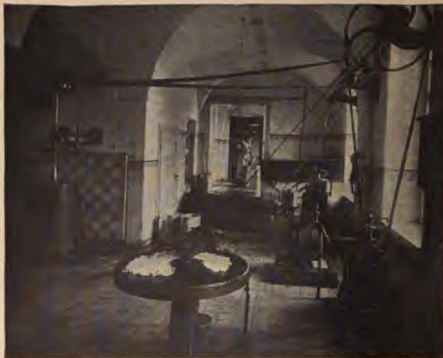
Fig. 12. An electrically operated dairy. Churn, butter machine and separator, operated from a common motor by means of counter, shaft and belts.
