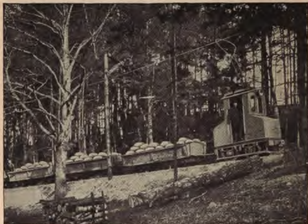
Fig. 30. Electric railway for handling farm products on a farm in Germany.
