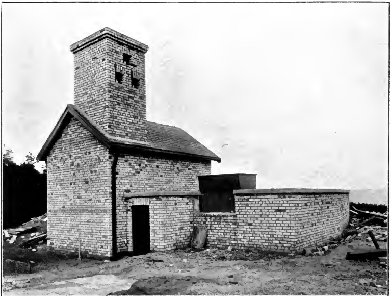
PLATE 30C.—Fan House at one of the Lambton Collieries, with one of the Fans driven by a Three Phase Motor. The Wires conveying the Current are shown entering the Tower of the Fan-house. By Messrs. Bruce, Peebles & Co.
