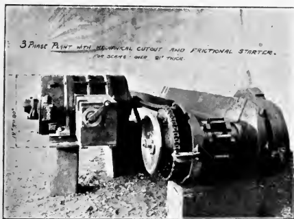
PLATE 31C.—Blackett's Underground Coal Conveyor with Three Phase Motor. The Trough shown on the Right is the Conveyor.
