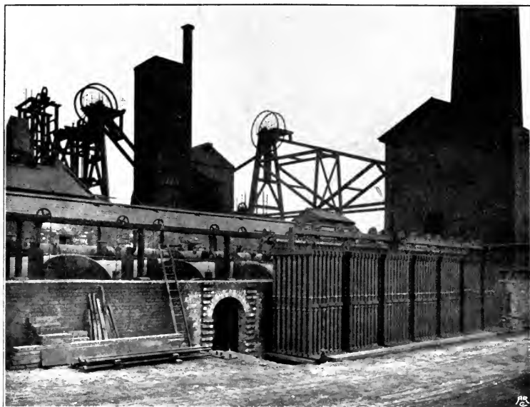
PLATE 3A.—A Battery of Green's Economizer Tubes in Process of being Fixed at Pendlebury Collieries. The Tubes will be built in, the Flue shown being connected to the Chamber.
