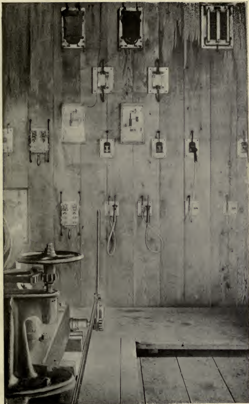
Plate VII. Motor Switch-Board.
