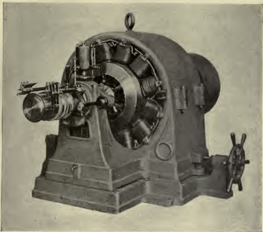
Plate VIII. Machine used as Generator and Motor at Telluride, Colorado.
