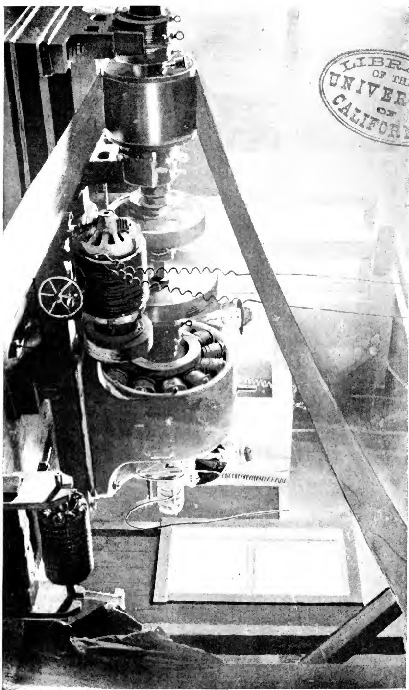
Plate VI. Motor in operation. Standard Con's Mill.
