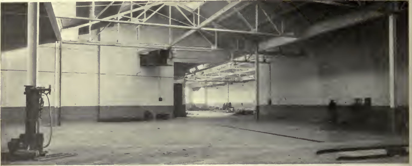
View of the bus garage looking toward the storage end. At the left of the doorway may be seen the ventilation hood and above the hood, the steel roof truss construction. Buses are serviced and repaired in the rear section of the garage
