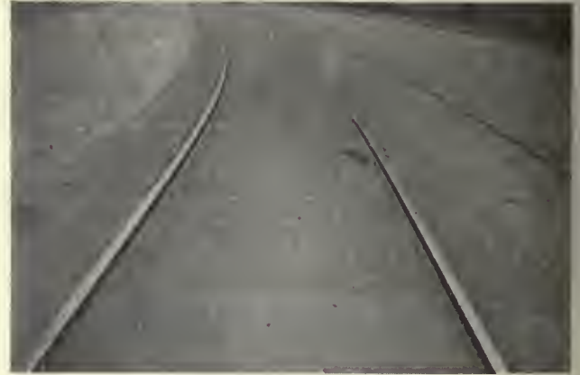
Fig. 12—Finished curve track construction
