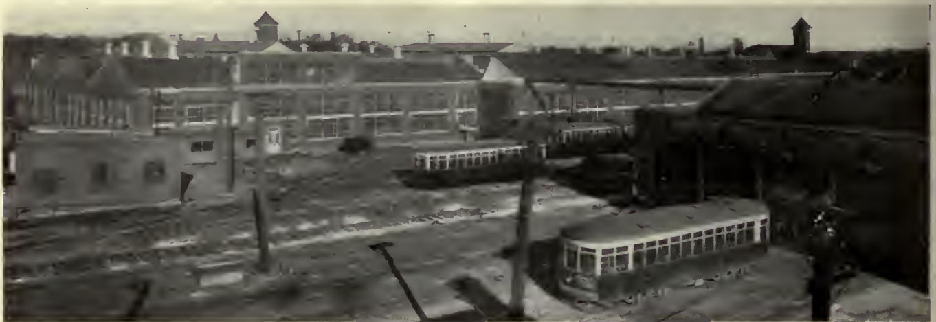
The size of the new building can be seen in this view, which also shows the old inspection barn and a section of the storage yard. Note the many windows in the walls of the new building
