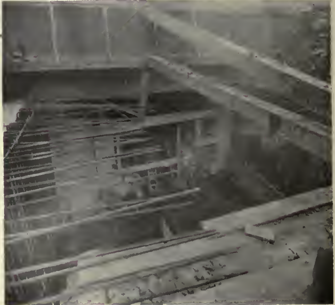
Building a culvert for Pittsburgh railways
