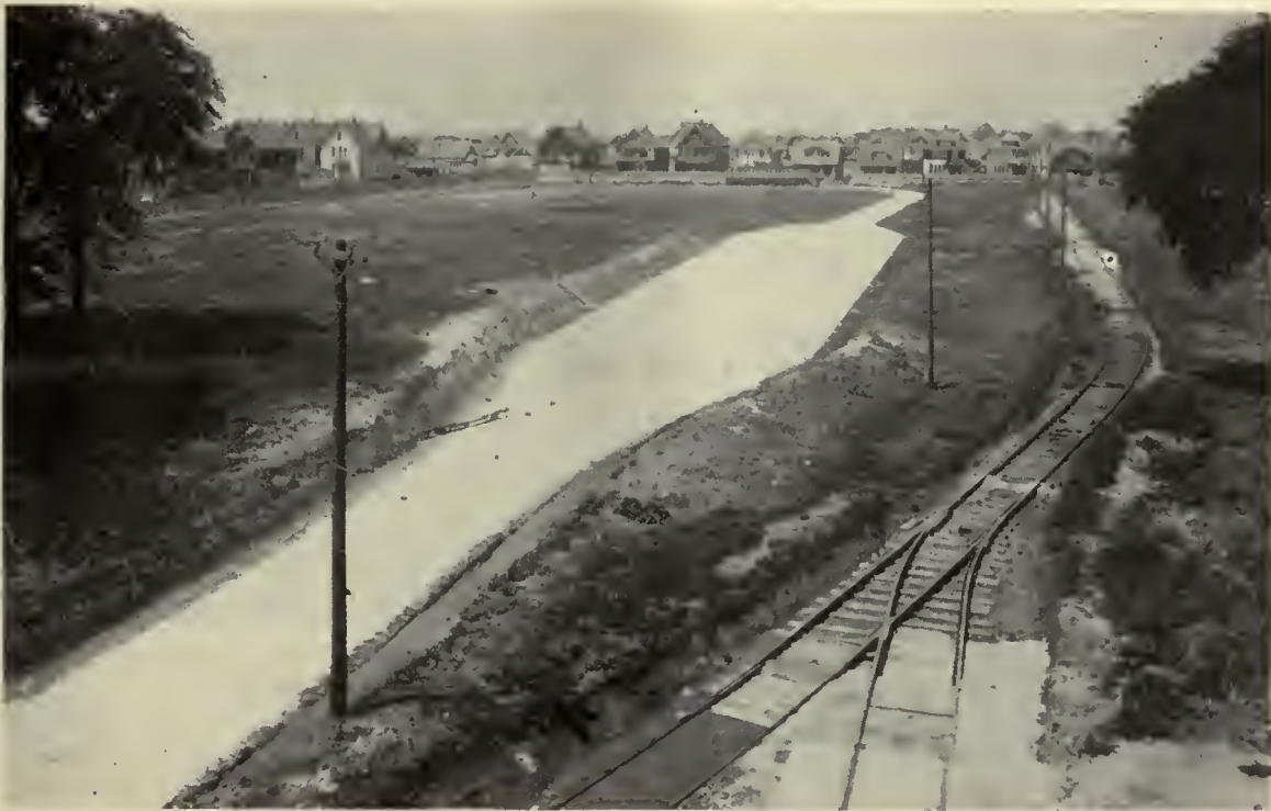
An oval practice track with stops, signals, switches and grades is used. Bus drivers practice on the macadam road shown in the center
