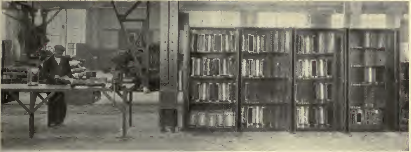
Motor suspension axle bearings are kept in cabinets and are marked with exact dimensions so that they can be fitted readily as needed. Accurate gaging is done on a bench
