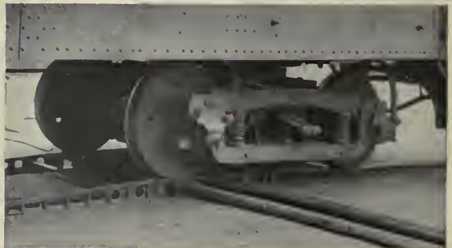
Easy grade of hose bridge prevents wheels scraping on car underframe
