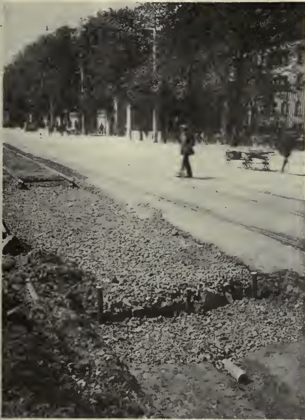
Fig. 16—Track under construction according to the design shown in Fig. 15
