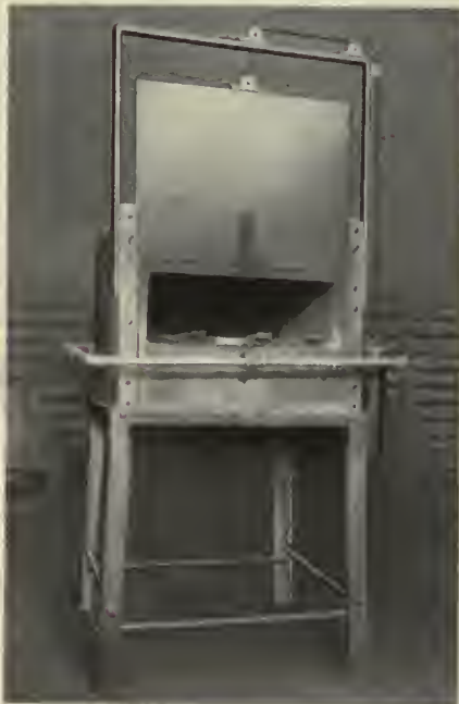
Shop constructed gas furnace
