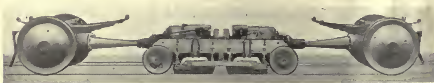
Early Zurich radial axle truck for Cardan drive
