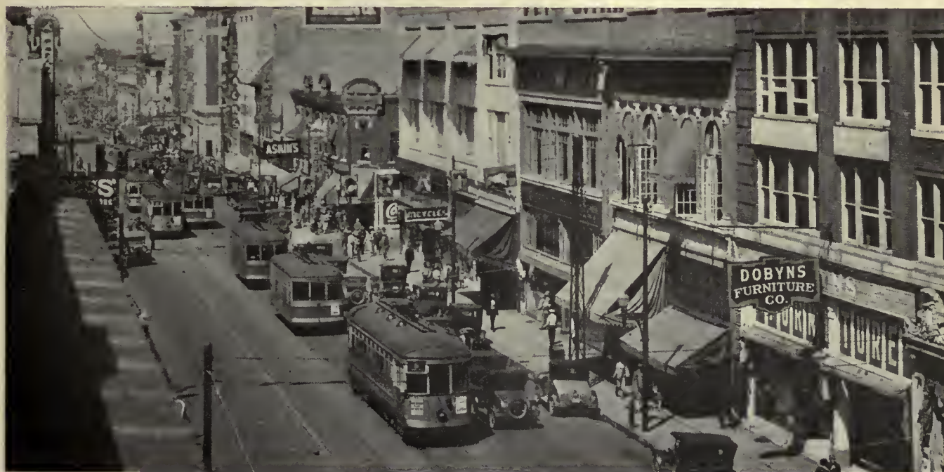
Both single and double-truck cars are used to give efficient modernized service in Little Rock, Ark. One-man operation has permitted frequent headways with resulting increased revenue and reduced expense
