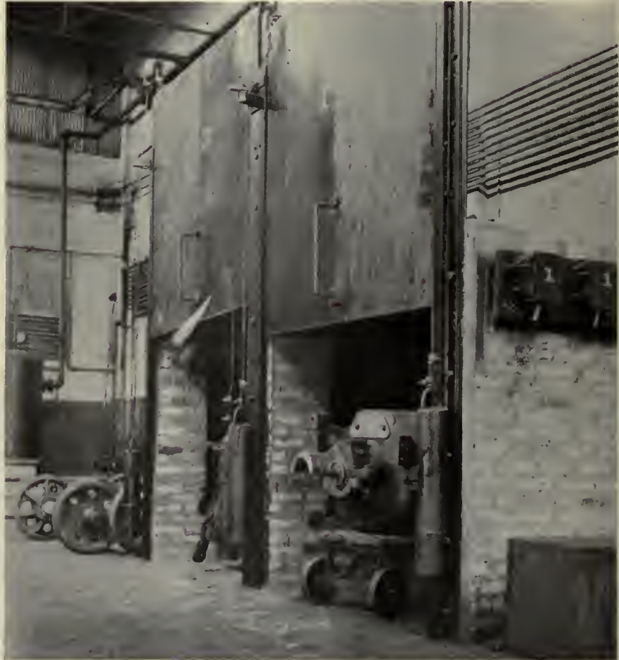
Bake ovens showing sliding doors, counterweights and motors being entered for preheating. The heater control switches can be seen on the brick wall
