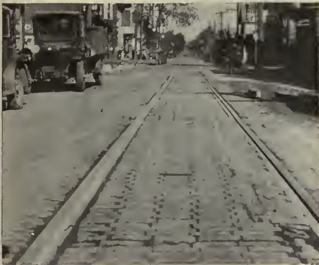
Track on West 18th Street before reconstruction was started
