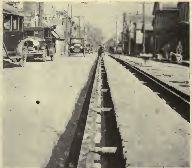
Replaced rail laid and lined
