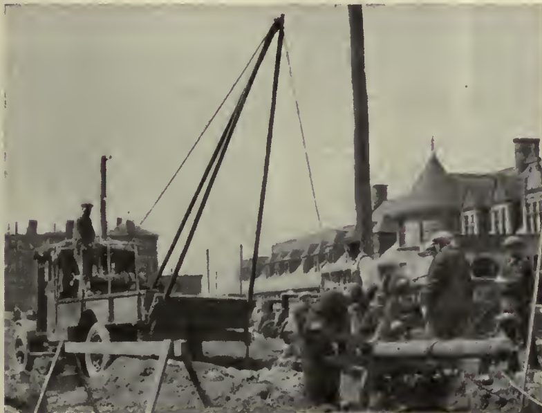
Convenient type of line truck with winch and tripod developed in Portland, Me.
