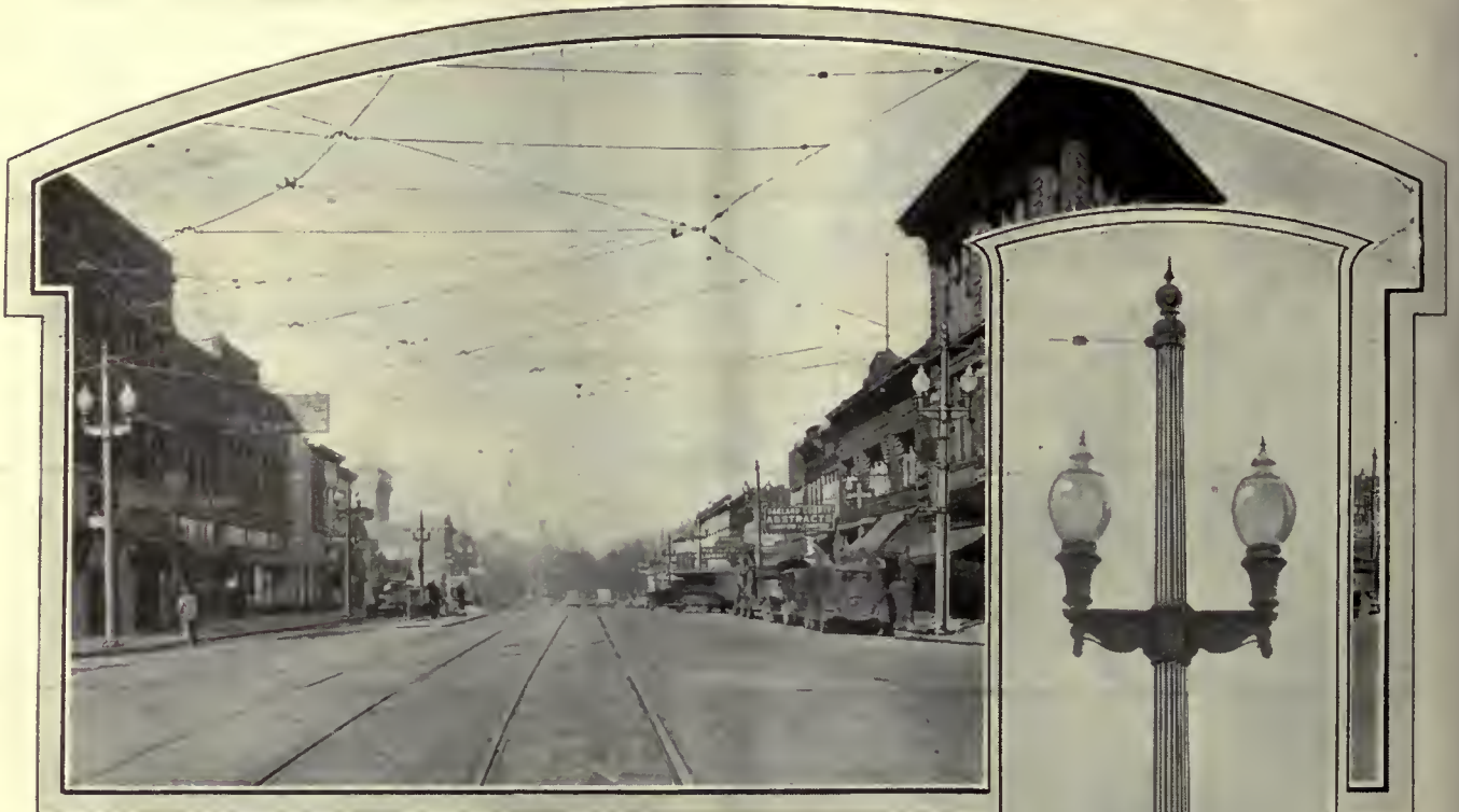
Saginaw Street, Pontiac, Michigan. Note the heavy overhead corner loading which the Union Metal Poles ably support.
