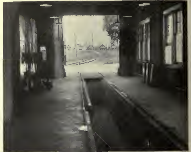
This 60-ft. track pit is so constructed that either a street car or a bus can be run over it
