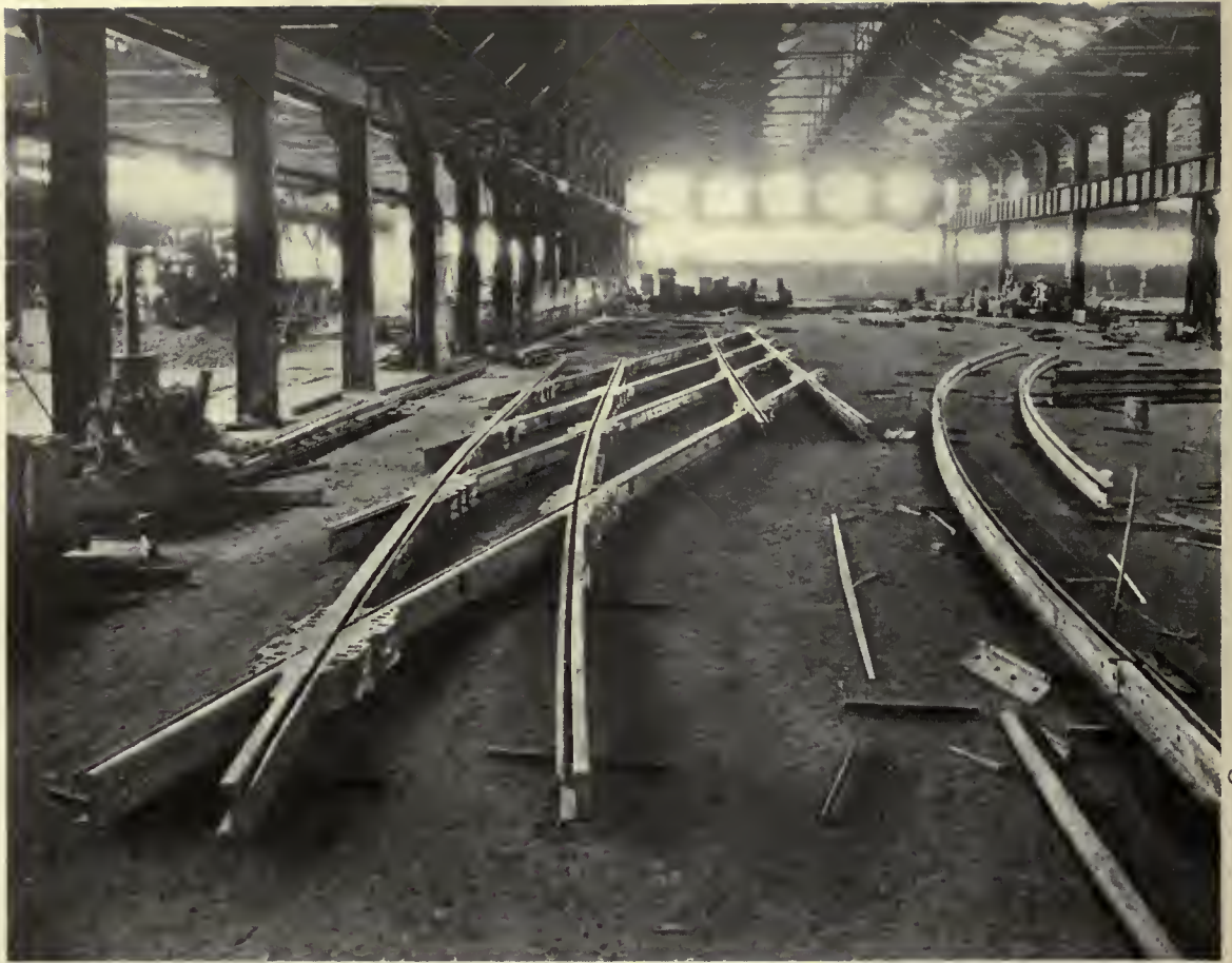
Part of the layout floor in the Bethlehem Frog and Switch Plant at Steelton, Pa.
