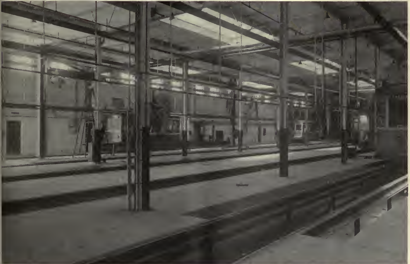
General interior view of Grove Street carhouse inspection bay. Note drop side inspection pit, Columbia car hoist and jib crane
