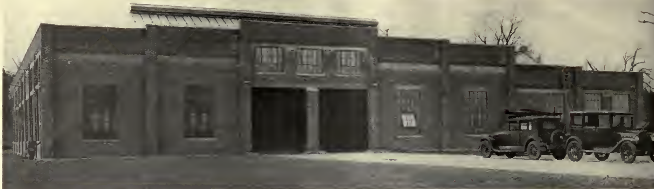
The new Grove Street garage. Space is available to extend the present unit in two directions
