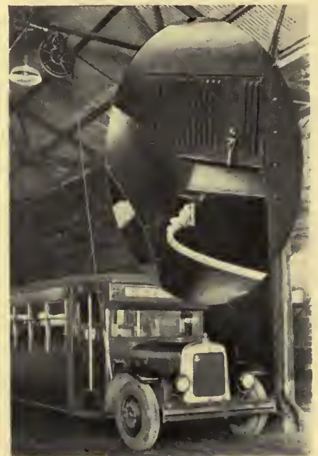
Spring return hose reel attached to roof truss with length of hose sufficient to reach several buses. Insert shows hose connection at bus
