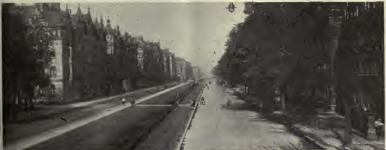
Fig. 17—High-speed railway on a reservation between Nuremberg and Fürth, 4 miles apart. Part of this line has three tracks and part has four tracks. It gives an express and local service
