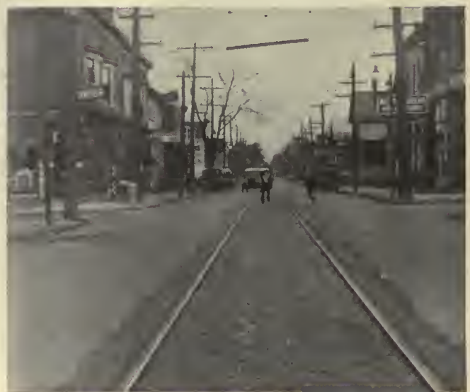
Completed track taken at the same point as the first picture
