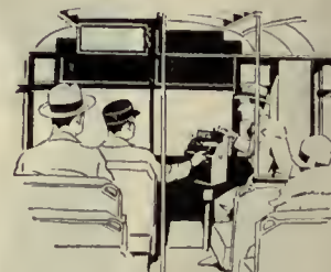
The indication of the National Fare Register is visible to passengers in the car.
