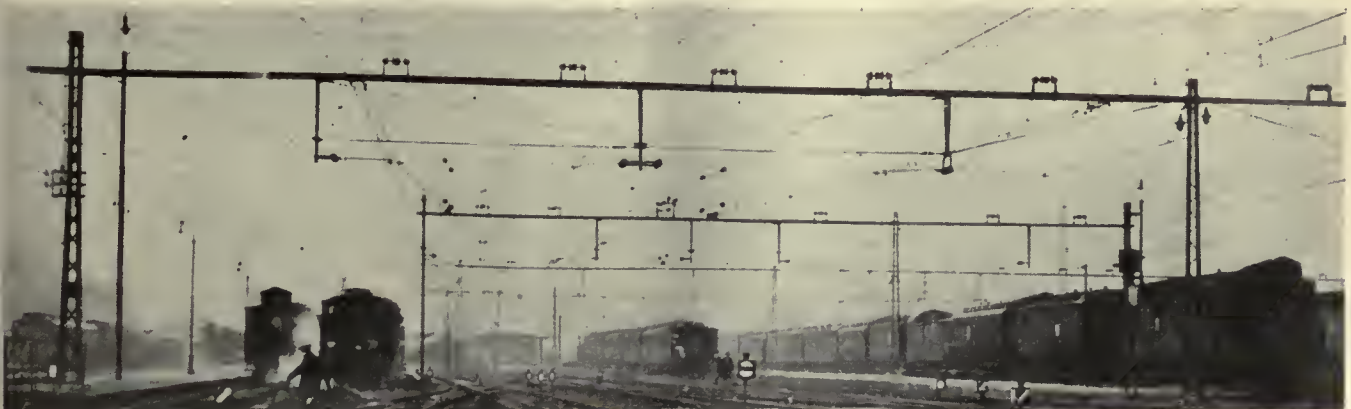
Old type yard construction with crossbeams in Silesia. Note absence of deflectors and use of intermediate wire
