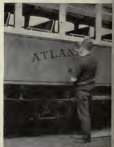
At left—After three coats of flat color have been applied and lettering and striping done, the car is given three coats of varnish. At right—Lettering and striping are done by hand
