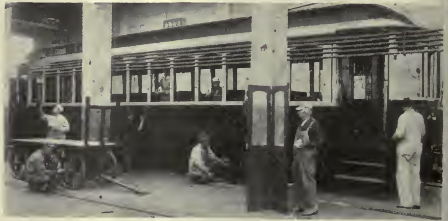
Car of the Atlantic City & Shore Railroad in process of being repainted "burning bush orange" with cream window posts
