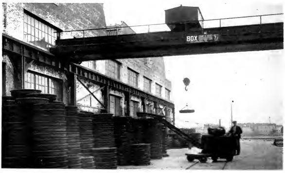
A convenient departmental storage for wheels and axles speeds up production. Material can be brought in on a car and unloaded by the overhead 7½-ton traveling crane. Wheels are loaded on small trucks and taken to the wheel and axle department by electric crane trucks
