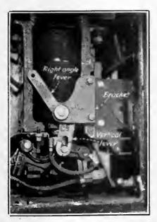
Device mounted on sectionalizing switch by which it is possible mechanically to close the contactor
