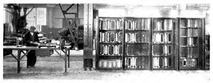
Motor suspension axle bearings are kept in cabinets and are marked with exact dimensions so that they can be fitted readily as needed.
