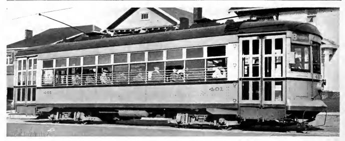
Twenty double-truck cars of this type were completely renovated and equipped for one-man operation. Automatic rear-exit treadles have since been installed on twelve of them
