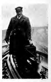
At left—The brush is made of flat steel bristles set in a hard wood block. Holes in the stem are for adjustment. In center—Two snow brushes are provided for each of the four third-rail shoe-beams of the cars. At right—When the snow brushes fail to remove sleet from the third rail, hydro-carbon oil burners are used
