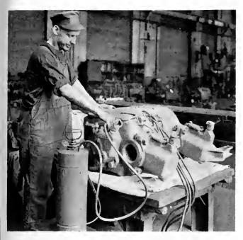
Filling the commutator end housing of a 35-hp. motor fitted with oil sealed housings and axle caps
