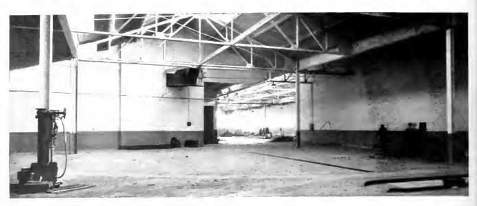
View of the bus garage looking toward the storage end. At the left of the doorway may be seen the ventilation hood and above the hood, the steel roof truss construction. Buses are serviced and repaired in the rear section of the garage
