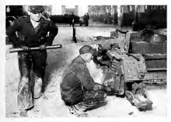
Bolts are installed under journal boxes quickly by means of a dever attachment that compresses the spring between the truck frame and the top of the journal box
