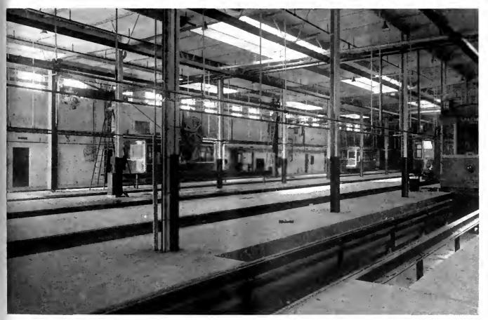
General interior view of Grove Street carhouse inspection bay. Note drop side inspection pit, Columbia car hoist and jib crane
