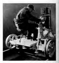
The operator's position has been chosen carefully to give a good view of the action of the tamping arms
