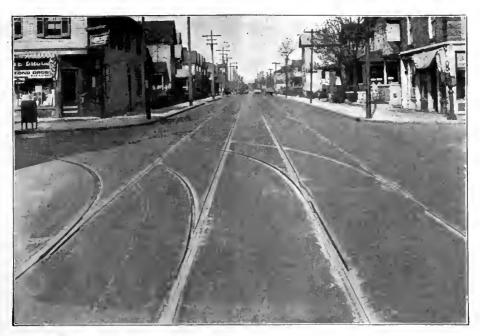
Looking west on Washington Street at the intersection of Cincinnati Street. Note the excellent condition of the tangentials and the smooth surface of the track area. Carey Elastite Track Insulation was used throughout.
