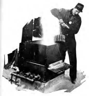
Removing a pinion from the hot water tank for installation on armature shaft
