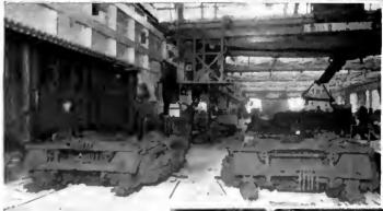
The entire operation of dropping out a truck is controlled from a station alongside the droppit table
