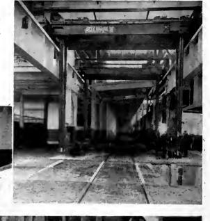
The drop-pit transfer table has a platform that raises and lowers. Longitudinal motion is provided by moving the entire table on rails at the bottom of the pit
