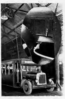
Spring return hose reel attached to roof truss with length of hose sufficient to reach several buses. Insert shows hose
