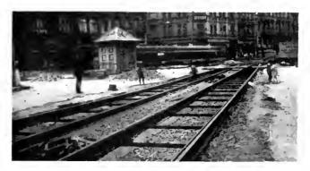
Fig. 10—Tangent track on concrete base with resilient filler and tie rods, before the installation of paving
