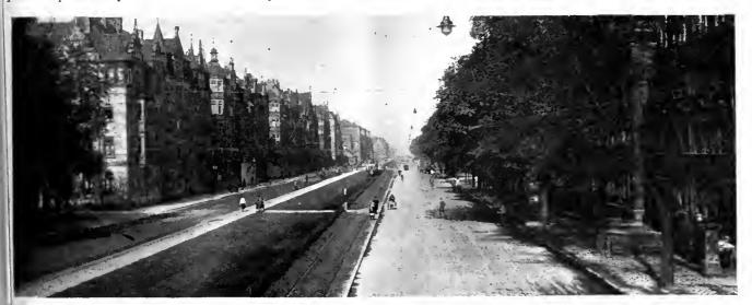
rig. 17—High-speed railway on a reservation between Nuremburg and Fürth, 4 miles apart. Part of this line has three tracks and part has four tracks. It gives an express and local service
