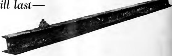
The unretouched photograph above shows a Carnegie Tie, just as it was taken from the road-bed, after eighteen years of service. The chief engineer, in charge of the reconstruction work, stated the ties were in excellent state of preservation after this long time, and both ties and clips were in fit condition for rail renewal.
