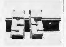
At left-80-lb. A.S.C.E. tee rail set up with 134-lb. girder groove rail. In center-Finished thermit weld. At right-A pair of mold boxes cut out and ready for applying to the joints
