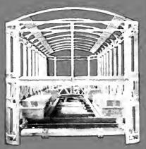
Rear view of Versare frame showing engine mounting and heavy channels affording protection at corners. When engine is installed this chanelling extends clear across the hack behind the bumper. Here you have bridge type truss construction, the same as used for strength in cantilever bridges and dirigibles. There is nothing like it in highway transportation vehicles. The girders, angles, castings and side posts are of Duralumin, an alloy selected where tremendous tensile strength is required.
