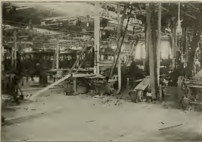
North Jersey Shops—General View in Carpenter and Erecting Shop.
