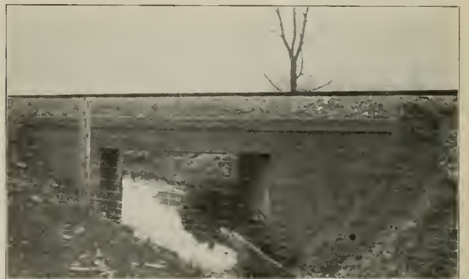
Marion Bluffton & Eastern Traction Company—Culvert Between Warren and Van Buren, Ind., with Square Top.
