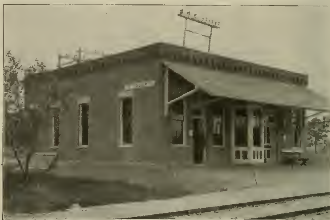
Lafayette & Logansport Traction Company—Standard Waiting and Substation.
