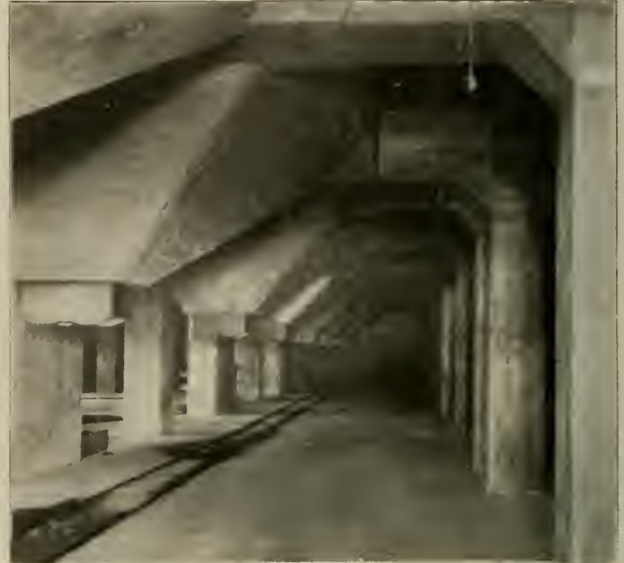
Seattle Electric Power Station—Ash Hoppers Under Boiler Room.
