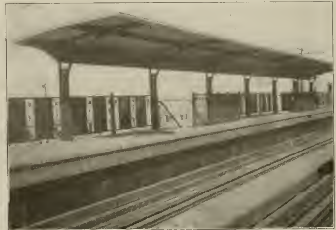
Ravenswood Extension of the Northwestern Elevated—View of Station Platform.
