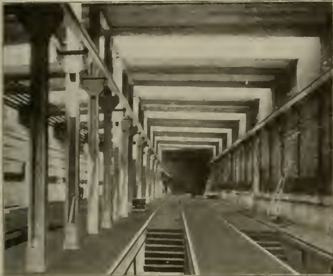
Brooklyn Rapid Transit Company—Interior of Repair Shops — Showing Inspection Pits.
