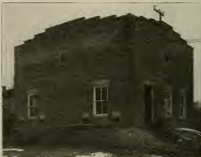
Pittsburg & Butler Street Railway—View of Rotary Substation.
