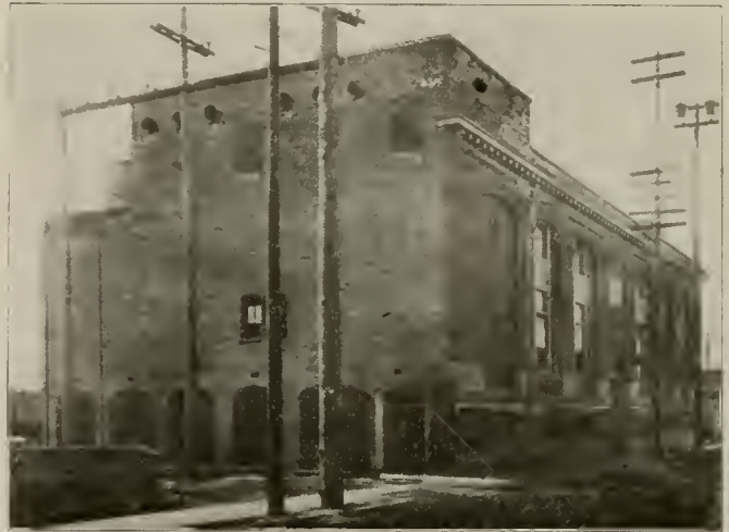
Portland Railway—Substation. Showing Outside Entrance to Transformer Compartment.
