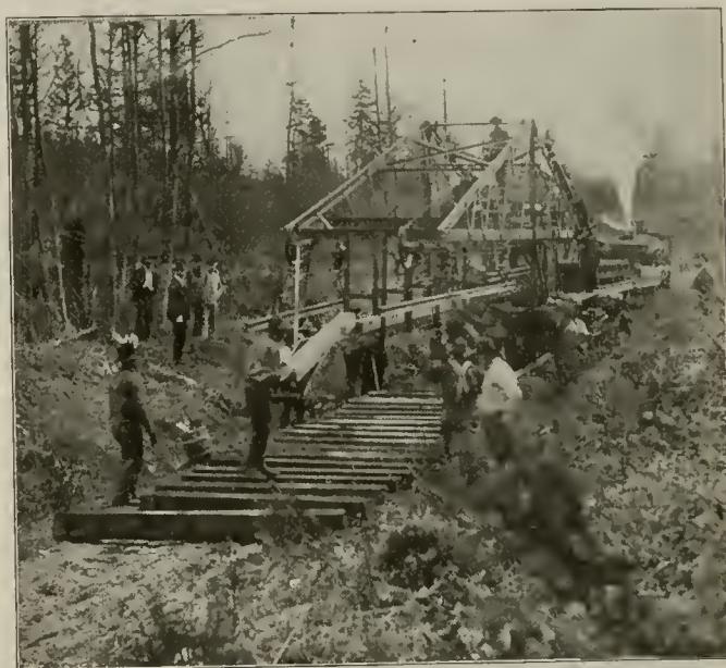
Wescott Track-Layer in Operation.
