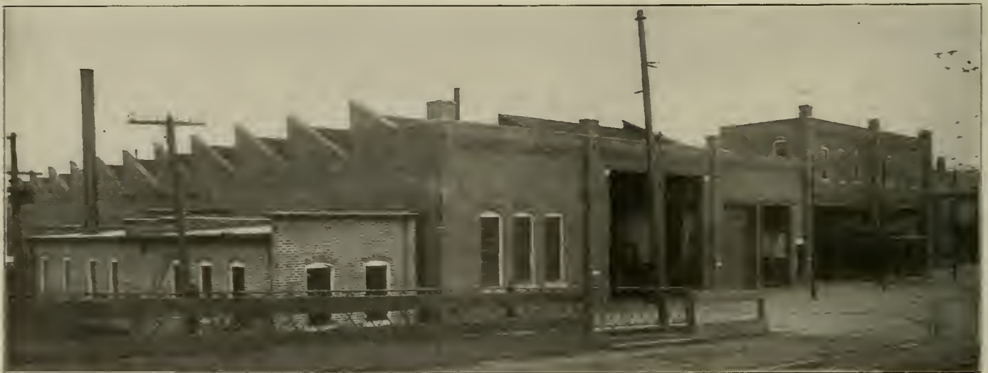
Car House and Shops at Knoxville—Exterior View, Showing Saw-tooth Roof.
