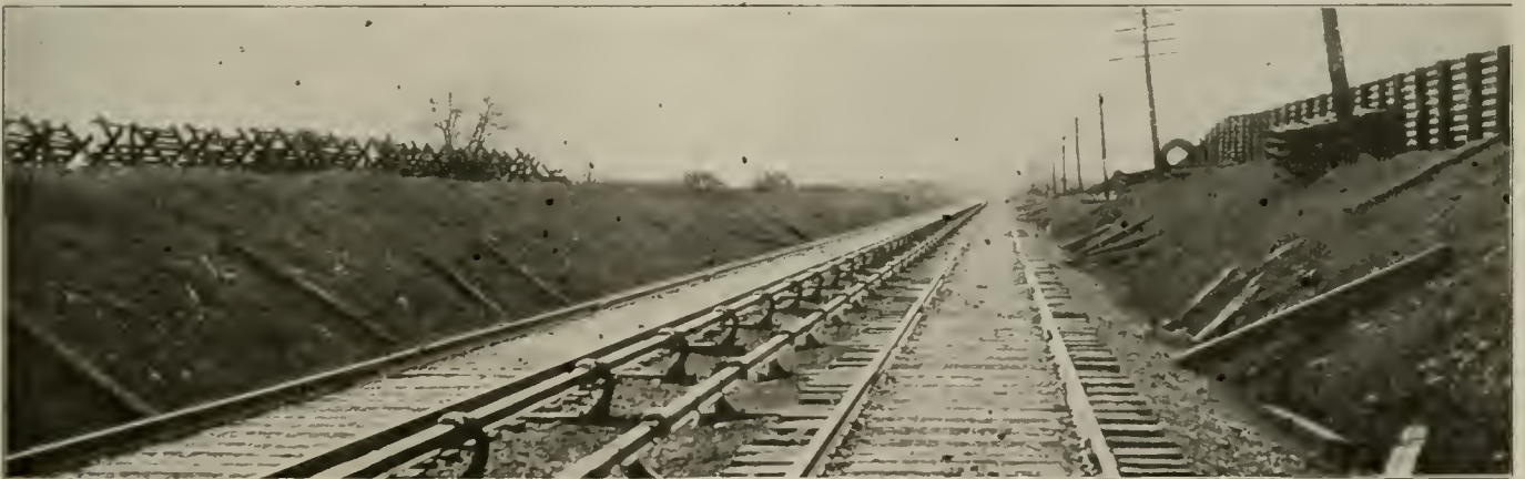
West Shore Electrification—Under-Contact Third Rail as Installed.
