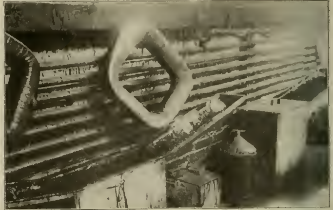
Shop Practice at Memphis—Arrangement of Dripping Vats and Drying Coils.
