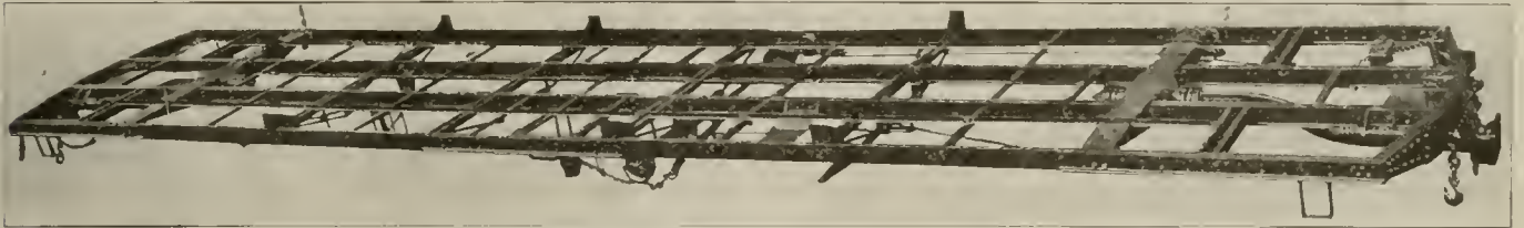
Hudson Companies Cars—Underframe, Showing Sills, Connections and Reinforcement.
