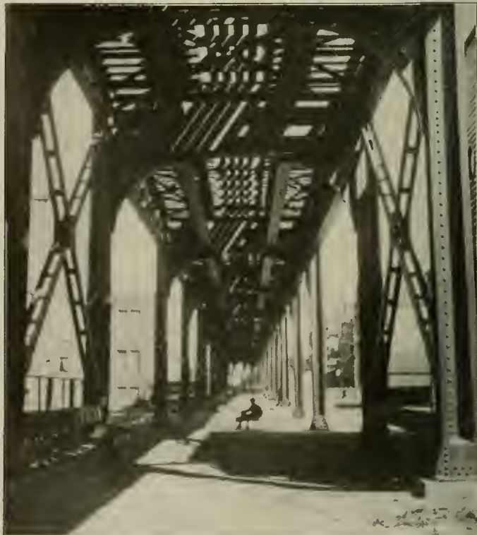
Ravenswood Extension of the Northwestern Elevated—View Under Structure, Showing Slight Obstruction to Light and Air.
