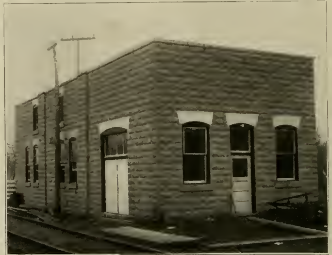
Marion Bluffton & Eastern Traction Company—Liberty Center Substation.
