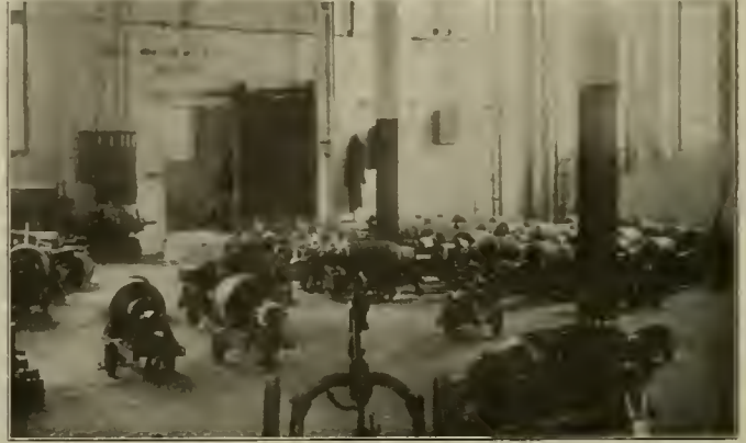
North Jersey Shops—Entrance to Bake-Oven Room, Showing Armatures on Buggies.
