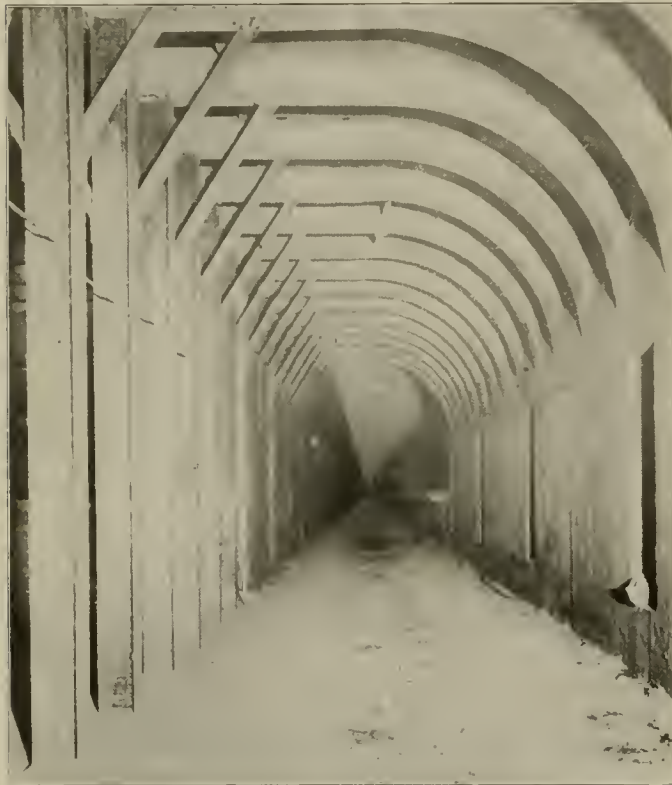
Rapid Transit in Boston—Concreted Steel Columns in Washington Street Tunnel.
