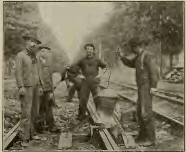
Thermit Rail Welding—Tapping a Cupola.
