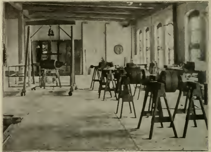
New Shops and Car Storage at Nashville—Winding Room.
