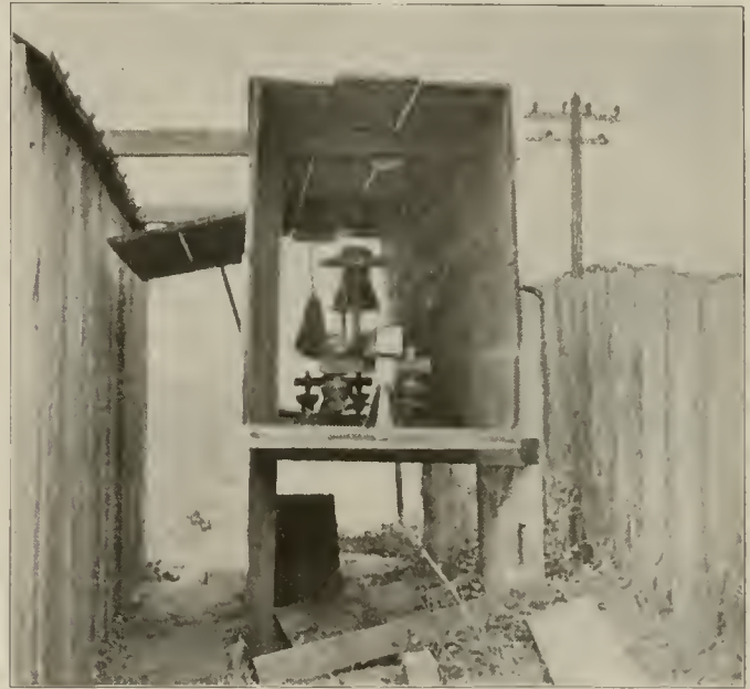
Insulators for Exceptional Service—Near View of Testing Box, Showing Insulator and Dust Bag.
