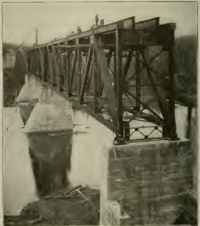
Ft. Dodge Des Moines & Southern Railway—Steel Deck Bridge.
