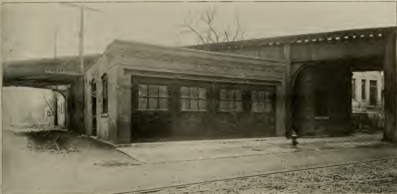
Metropolitan Elevated Railway—Exterior Robey Street Substation Showing Elevated Structure Above.
