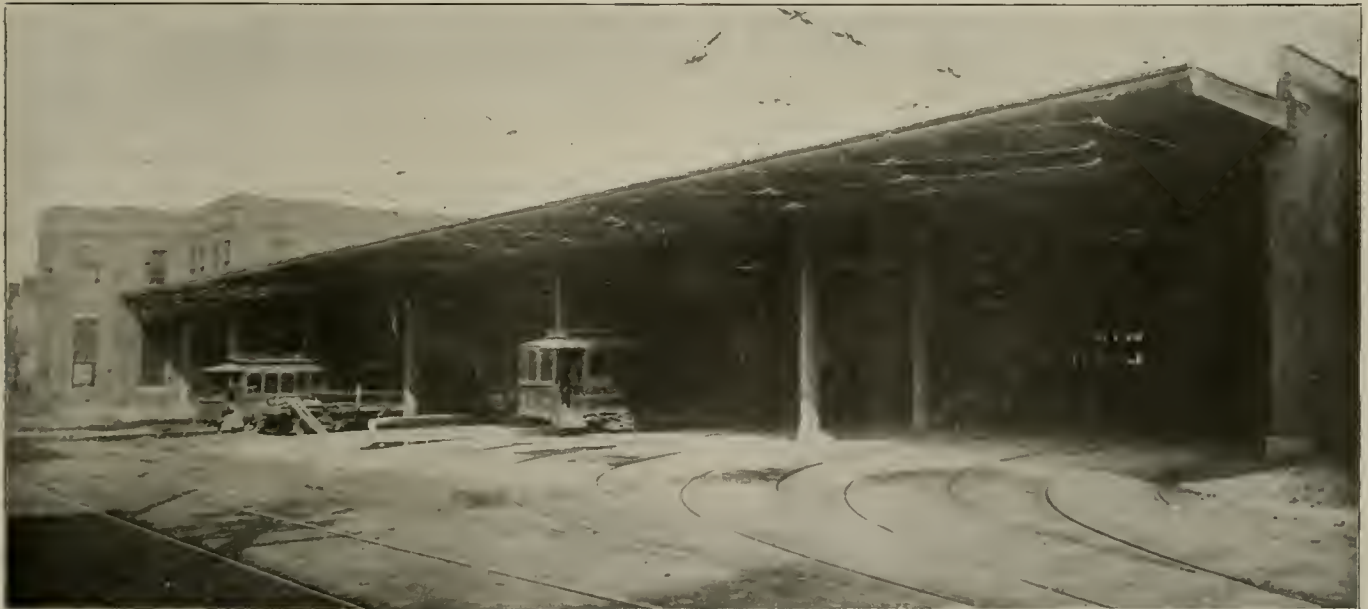
New Shops and Car Storage at Nashville—Fourth Avenue Structure with Projecting Roof and Doors.
