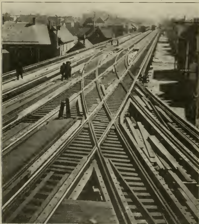
Ravenswood Extension of the Northwestern Elevated—View of Clark Street Junction.
