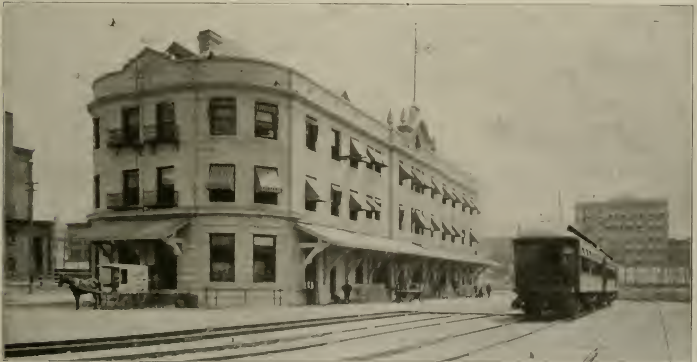
Spokane Electric Terminal—Exterior of Building.
