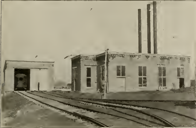
Ft. Wayne & Springfield Railway—Car Barn and Power House.
