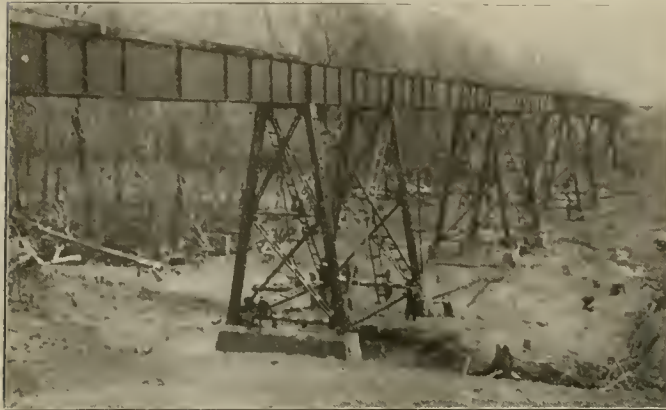
Lafayette & Logansport Traction Company—Rock Creek Viaduct, 394 Feet Long.
