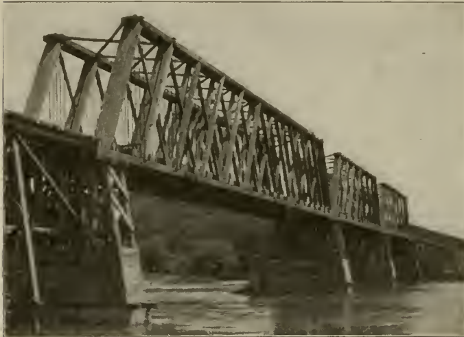
Ft. Dodge Des Moines & Southern Railway—Timber Truss Bridge Across Des Moines River.
