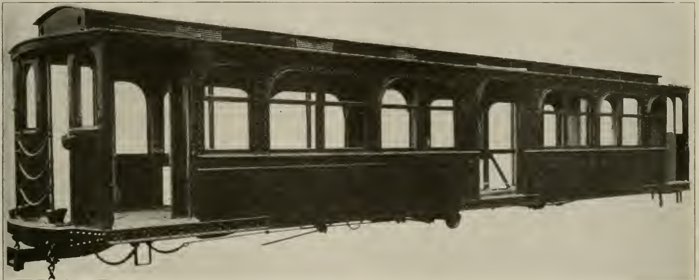
Hudson Companies Cars—Body with Sheathing in Place.
