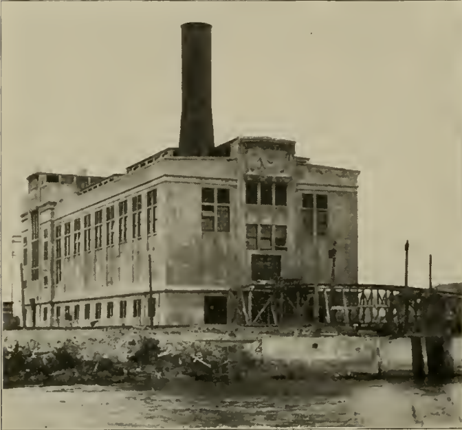
Seattle Electric Power Station—Exterior of Power Station.
