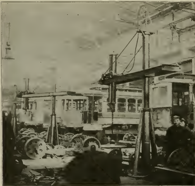
North Jersey Shops—Self-Supporting Jib Cranes with Air Hoists.
