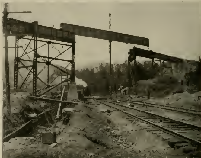
Pittsburg & Butler Street Railway—Showing Bridge at Bryant Under Construction.
