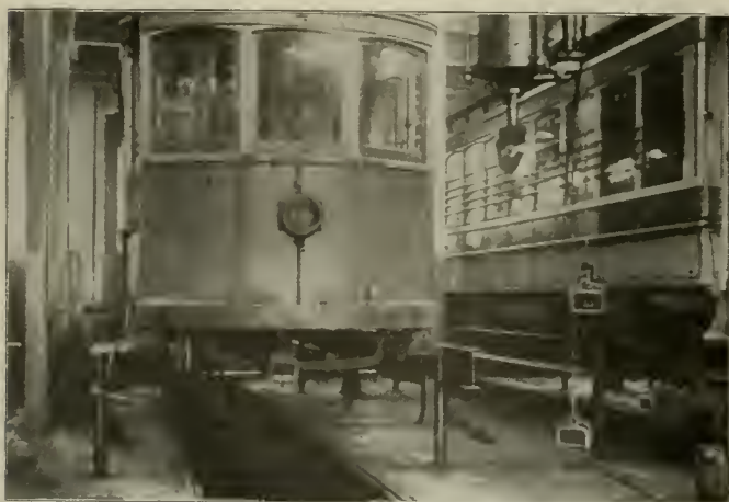
North Jersey Shops—Car Repair Pit with Body Hoist.
