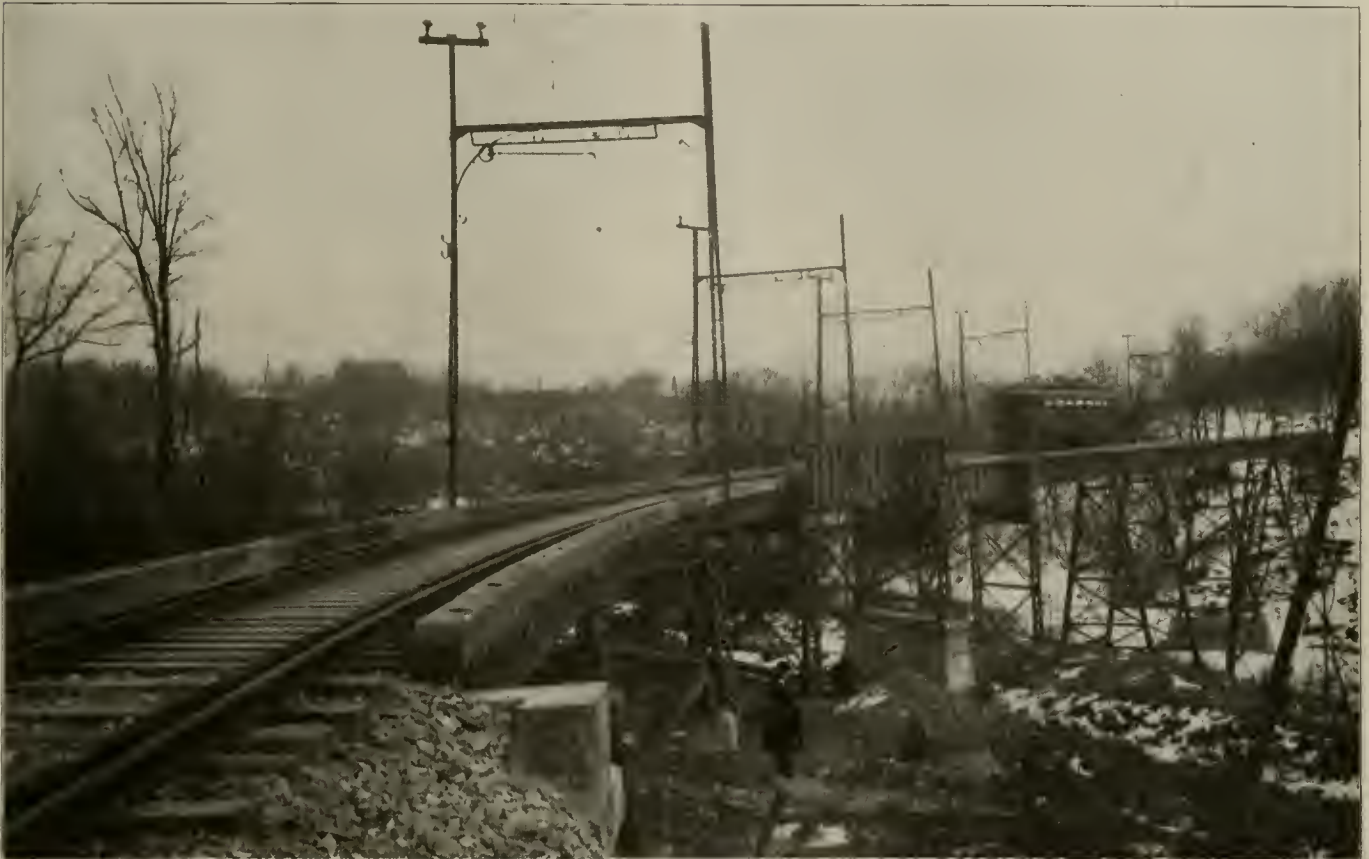
Pittsburg & Butler Street Railway—Bridge over Thorn Creek.
