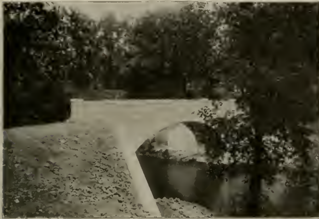
Dellwood Park—Single-Span Concrete Bridge.
