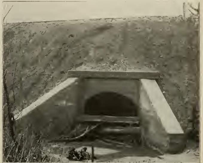
Marion Bluffton & Eastern Traction Company—Culvert in Fill Near Marion, Ind.
