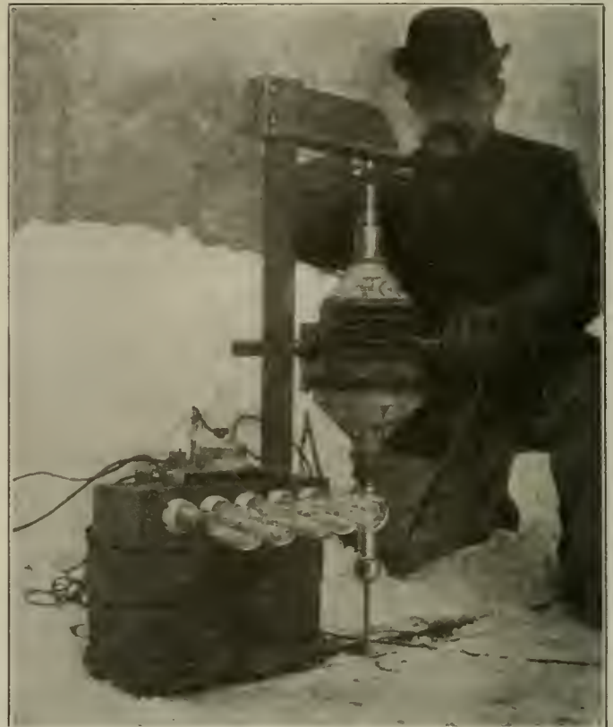
Brown Plastic Rail Bond—View Showing Clamp and Lamps for Night Work.
