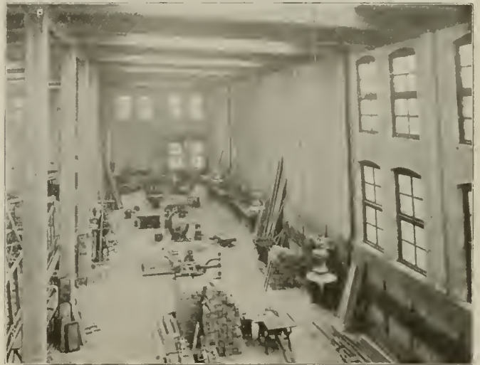
New Shops and Car Storage at Nashville—Interior of Carpenter Shop.
