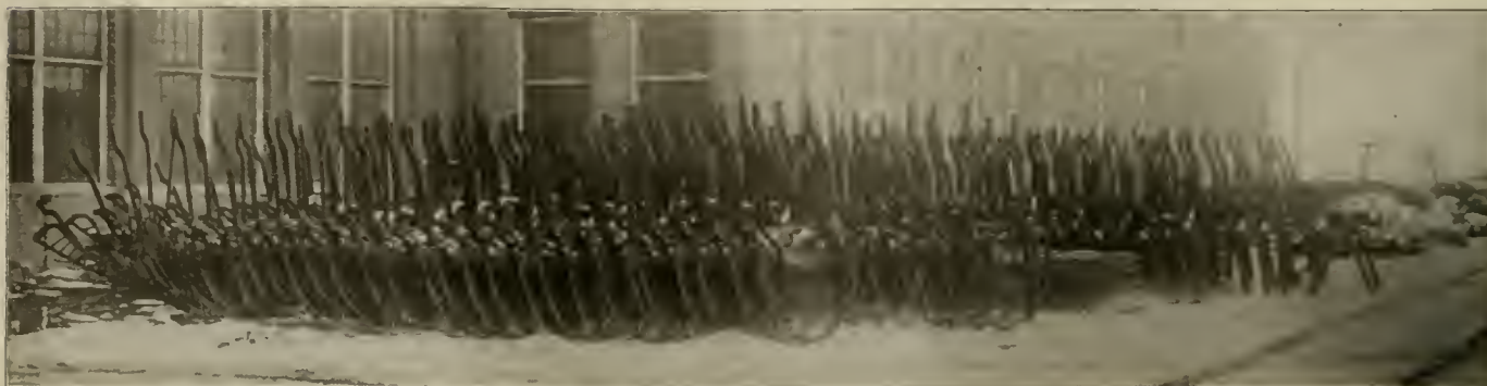
North Jersey Shops—Fenders Piled Adjacent to Blacksmith Shop.
