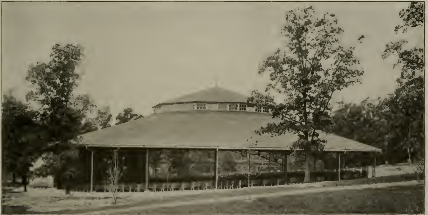
Dellwood Park—Steel Auditorium in Chautauqua Grounds.
