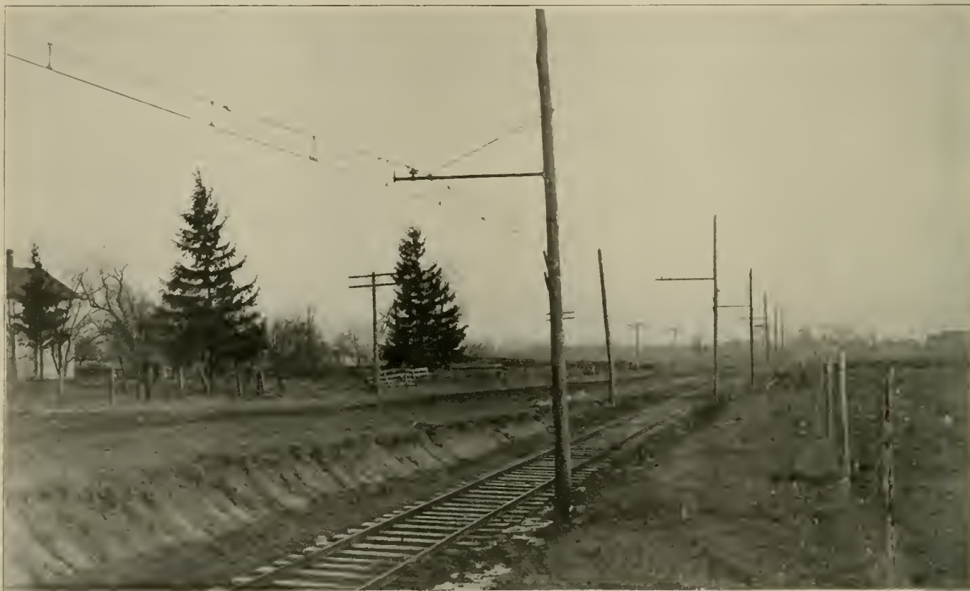
Ft. Wayne & Springfield Railway—Catenary Construction on Tangent.
