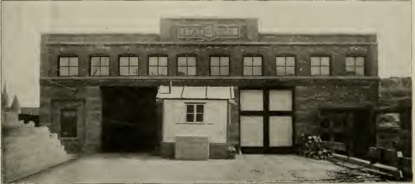
Ash-Handling by the Brooklyn Rapid Transit Company—General View of Receiving Station.
