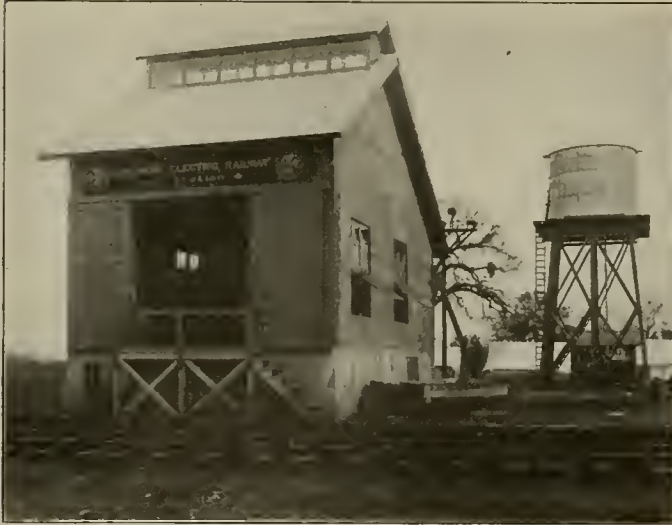
Northern Electric Railway—Typical Substation Structure.
