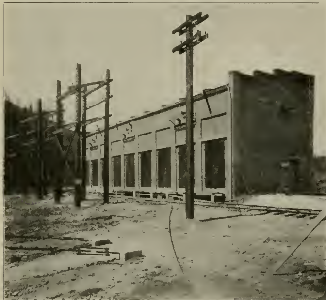
Cazadero Station of the Portland Railway—Step-up Transformer Station.
