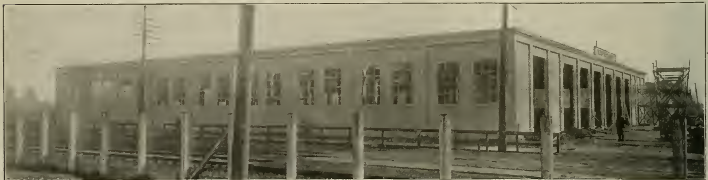
New Shops at Seattle—Exterior of Machine Shop Showing General Type of Buildings.
