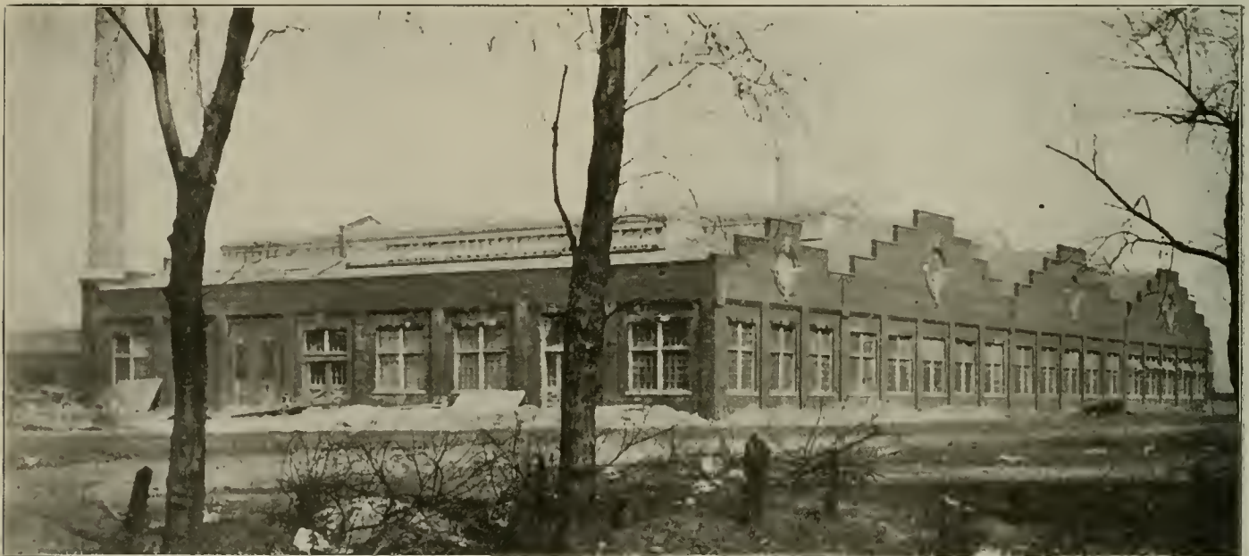
Camden Shops, Public Service Corporation—General View of Buildings.
