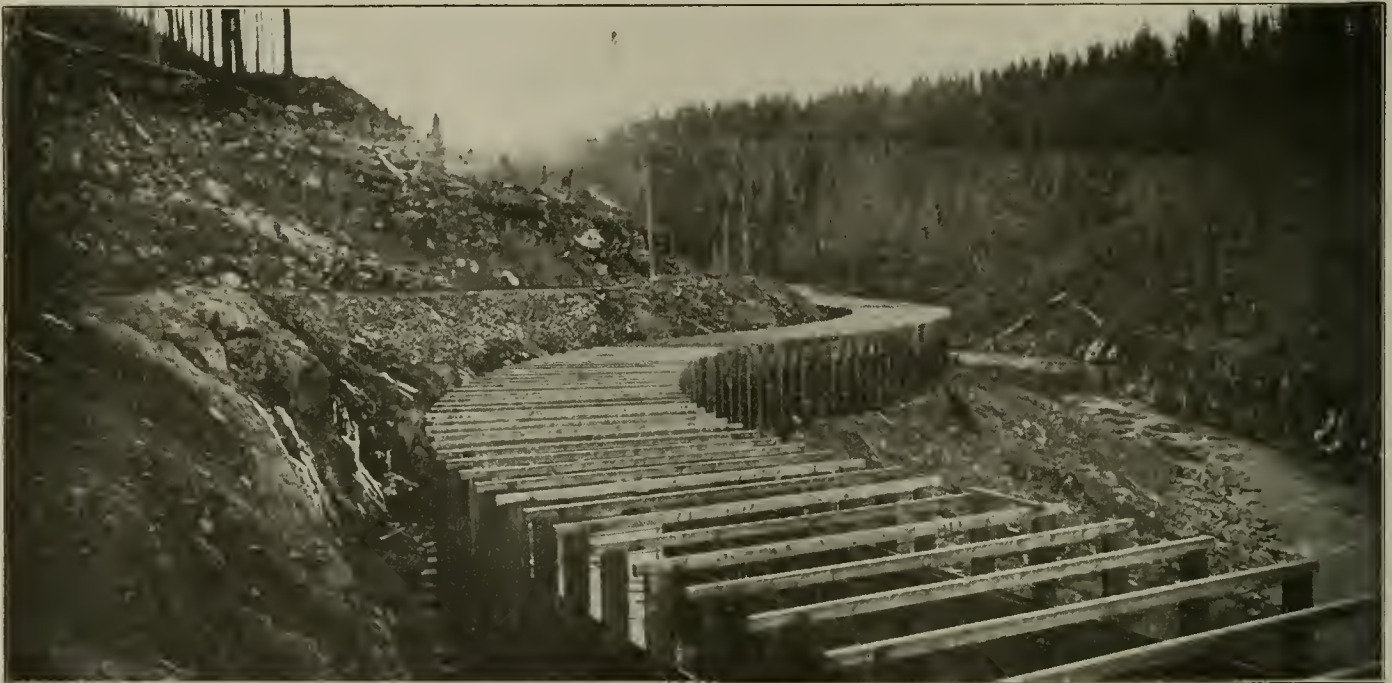
Cazadero Station of the Portland Railway—Open Flume Along River Bank.
