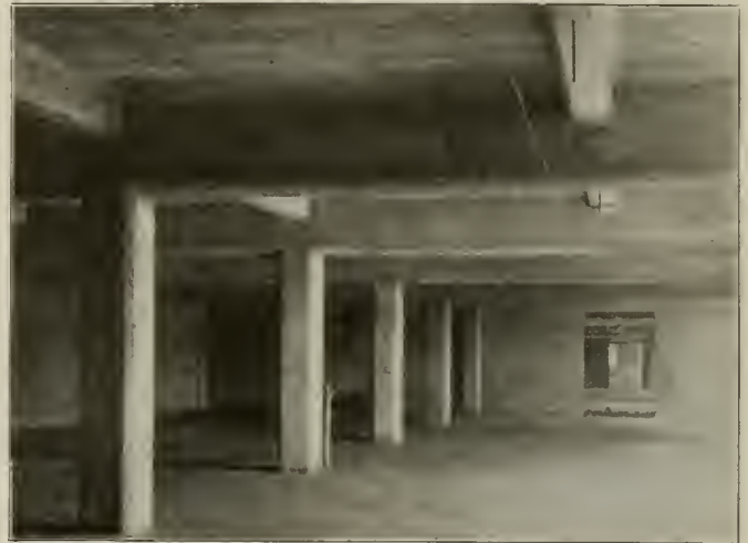
New Shops at Seattle—Interior of First Floor of Store Room, Showing Massive Concrete Construction.
