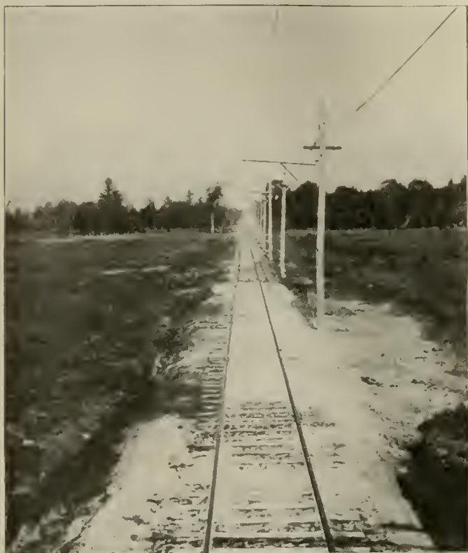
Manchester-Nashua Street Railway—Standard Track and Overhead Construction.
