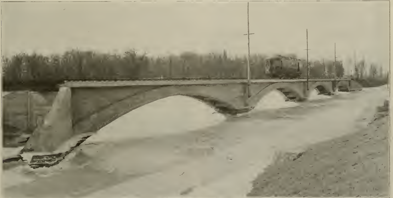
Elgin & Belvidere Electric Company—Kishwaukee Bridge.
