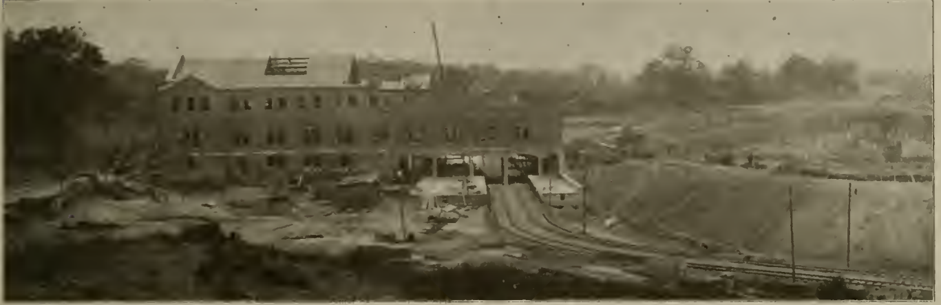
Market Street Terminal, Philadelphia—General View Showing Construction Work in Progress.
