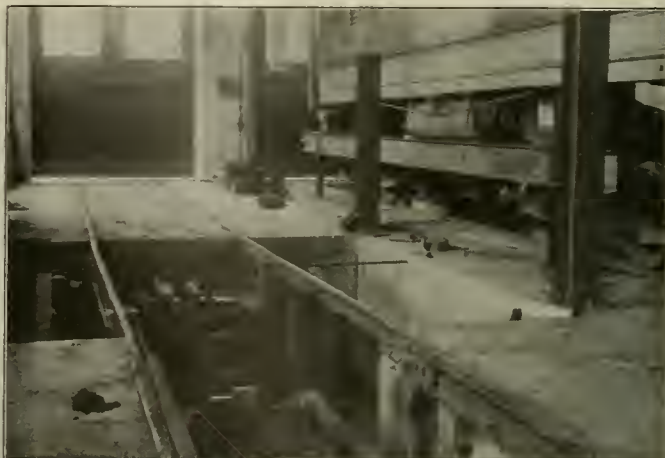
North Jersey Shops—Drop Pit with Wheel Grinding Apparatus.
