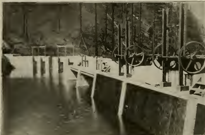
Cazadero Station of the Portland Railway—Gates Leading to Penstocks and Spillway.
