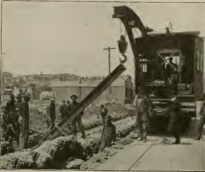
San Francisco Track—Lifting Cable Yokes and Concrete with Derrick Car.
