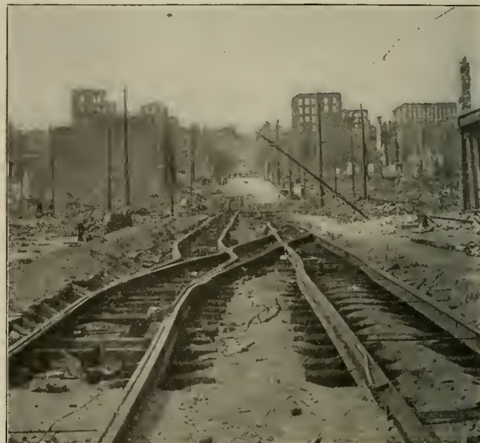
San Francisco Track—Condition of New Unpaved Track in Street After Earthquake and Fire.
