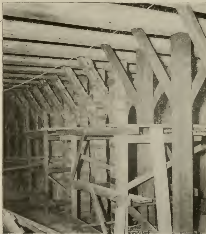
Rapid Transit in Boston—Washington Street Tunnel Under Construction.
