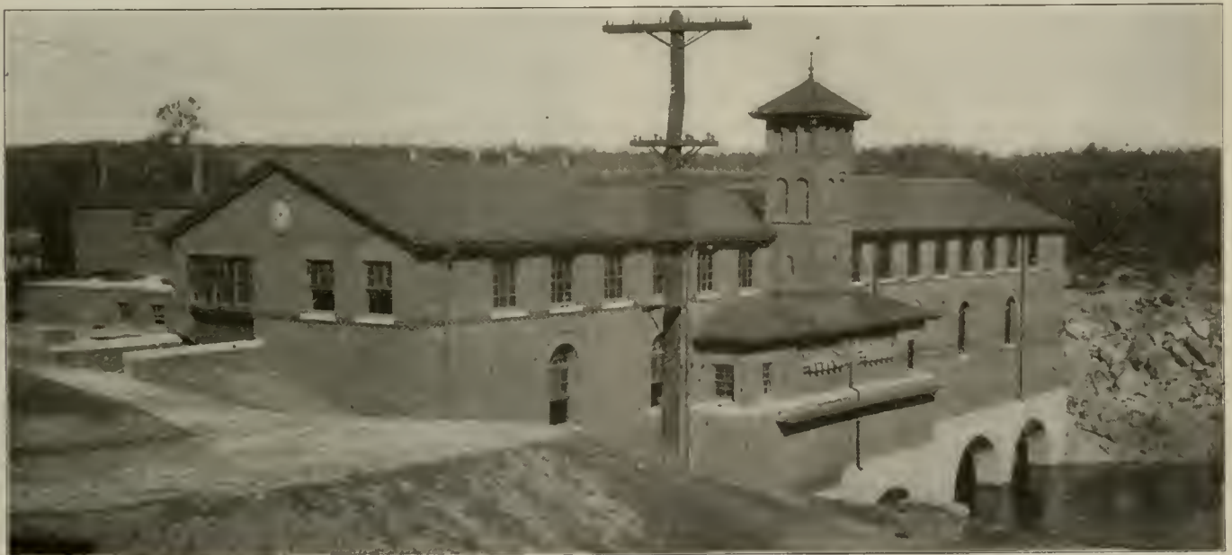
Manchester-Nashua Street Railway—Garvins Falls Hydro-Electric Plant.
