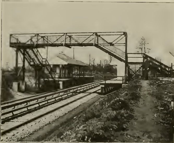
Philadelphia & Western—Typical Station with Overhead Footbridge.
