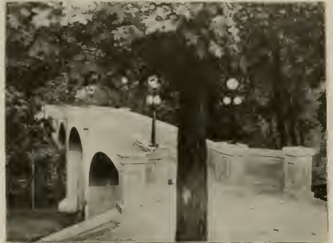
Dellwood Park—Three-Span Concrete Bridge.
