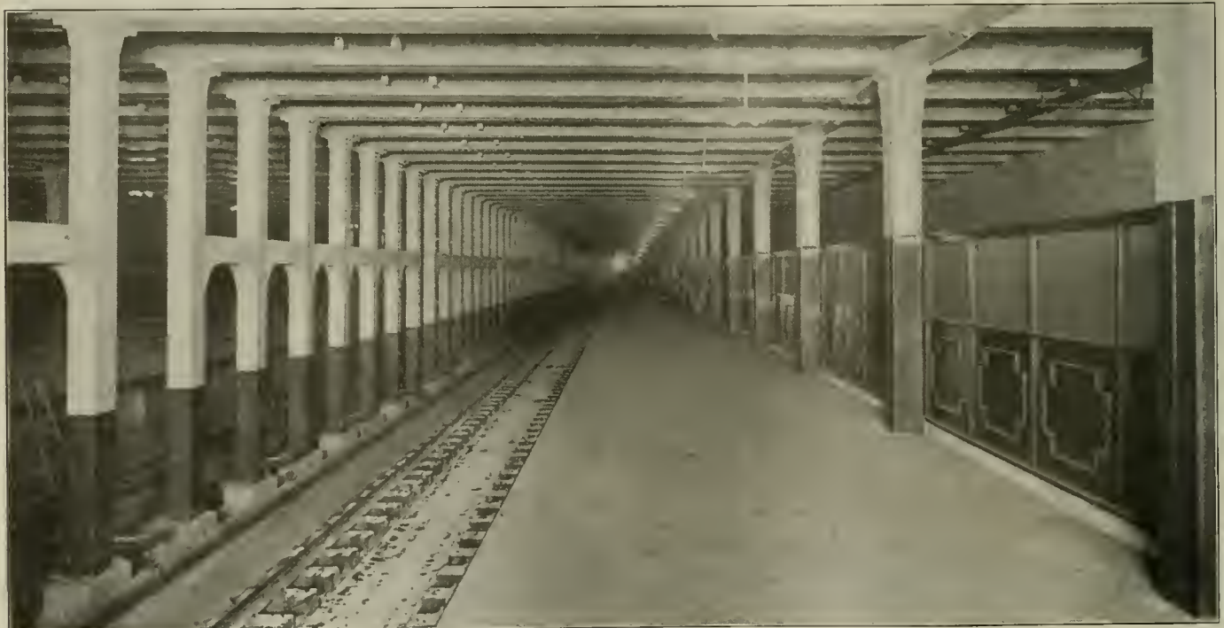
Market Street Elevated, Philadelphia—Interior View of Subway Station at Fifteenth and Market Streets.
