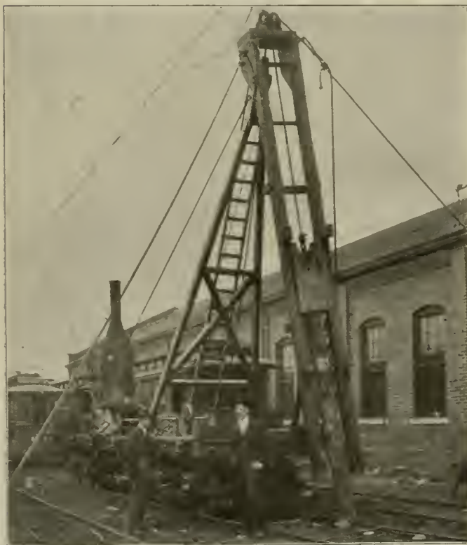
Shop Practice at Memphis—Pendulum Pile-Driver.
