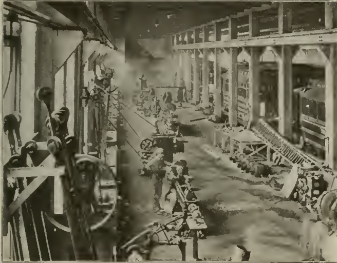
New Shops and Car Storage at Nashville—Interior of Machine Shop.
