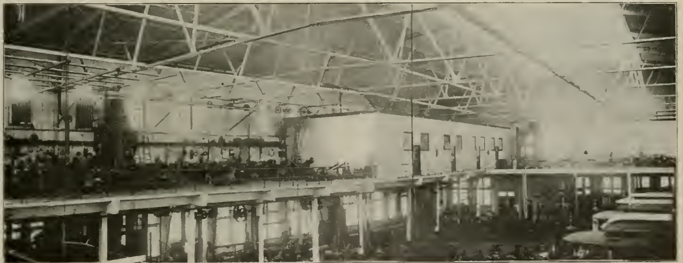
North Jersey Shops—General View Interior of Machine Shop.
