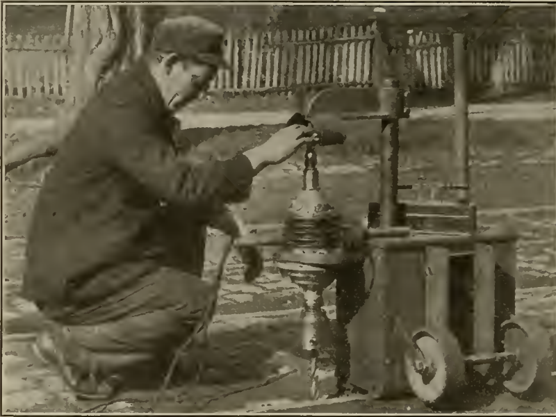
Brown Plastic Rail Bond—View Showing Method of Drilling Holes.
