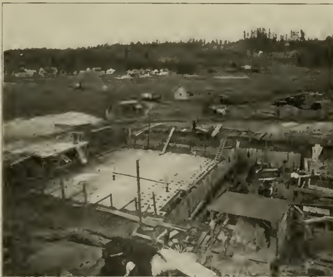
Seattle Electric Power Station—View of Engine Foundation During Construction.
