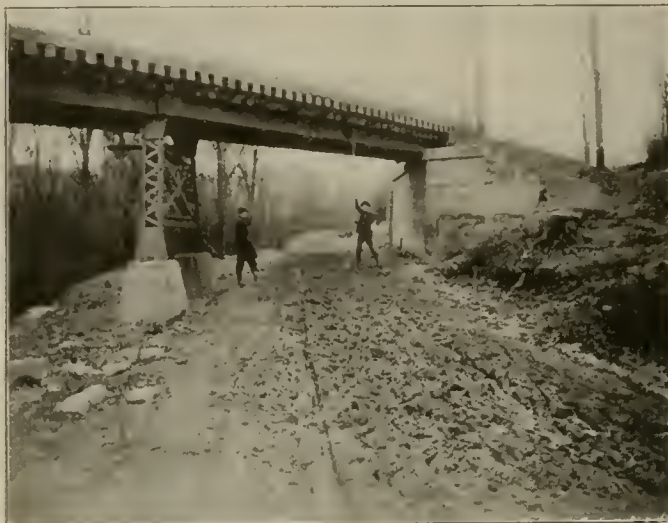
Pittsburg & Butler Street Railway—Showing Concrete Abutment of Thorn Creek Bridge.
