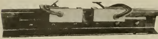
Copper-Welded Rail Bonds—Clay Molds in Position for Cast Welding.
