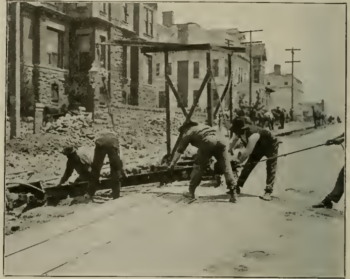
San Francisco Track—Breaking Brick Cable Conduit with Battering Ram.
