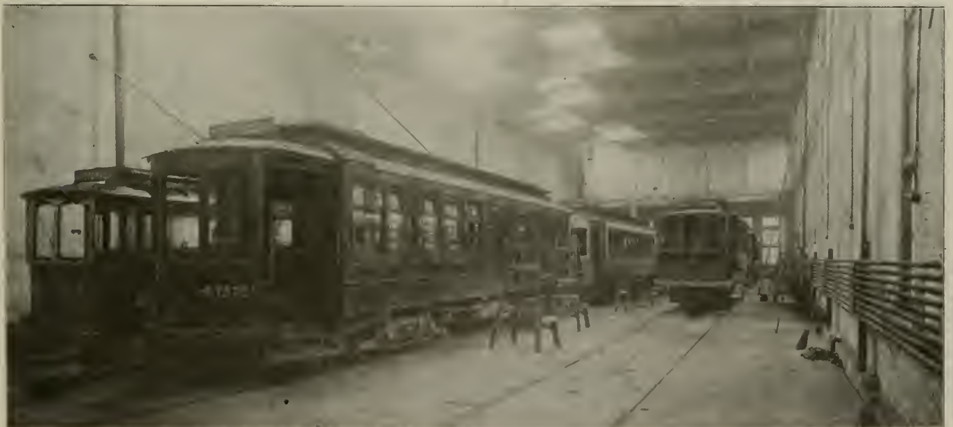
New Shops and Car Storage at Nashville—Interior of Paint Shop.
