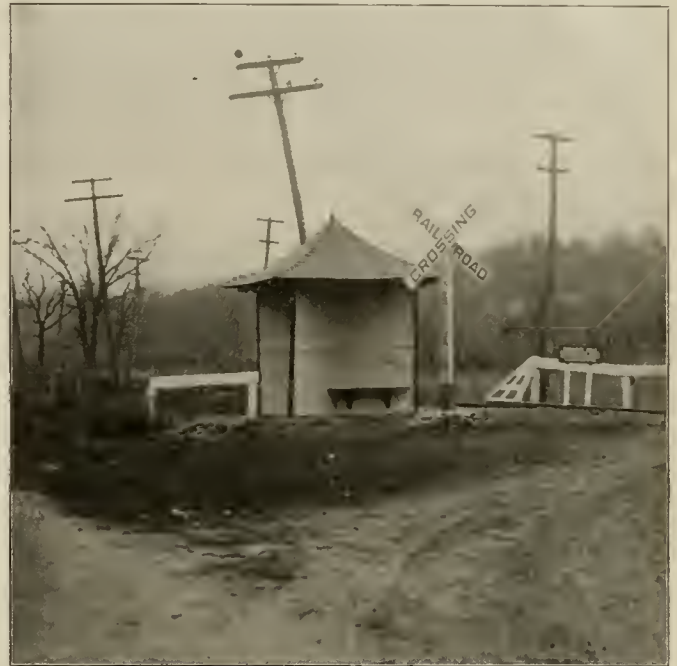
Illinois Valley Shelter Shed—General View.
