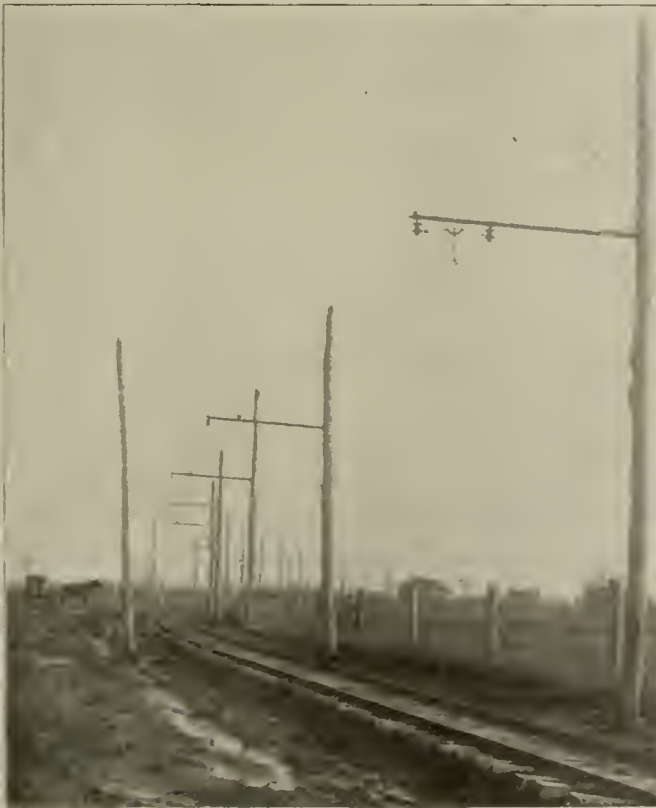
Ft. Wayne & Springfield Railway—Catenary Construction on Curves.
