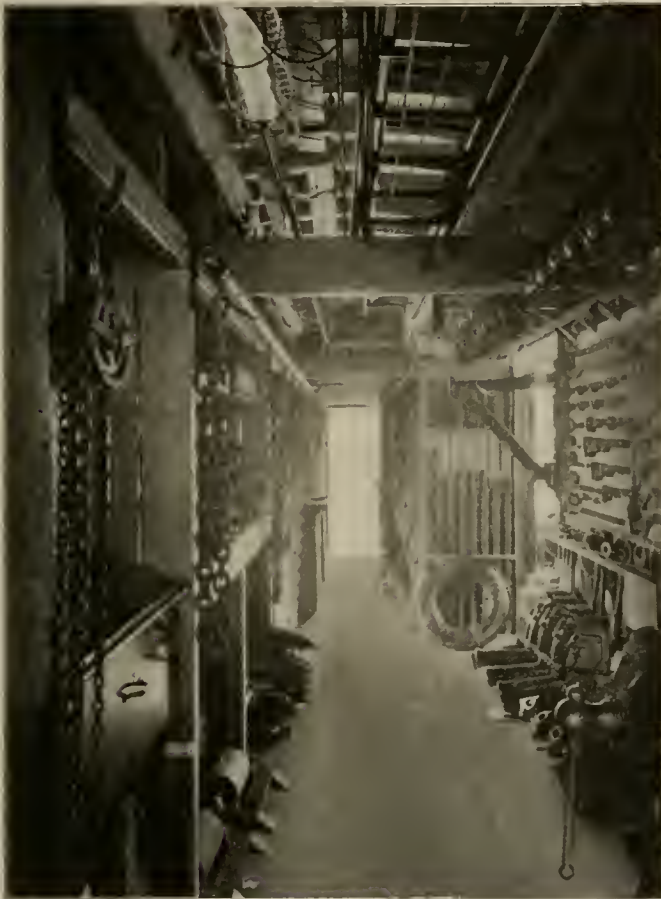
Oakland Wrecking Car—Interior, Showing Very Complete Equipment of Tools.
