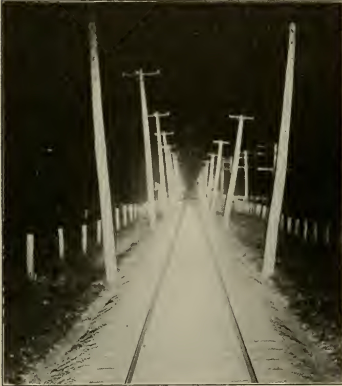
Night View Showing Comparative Headlight Illumination.
