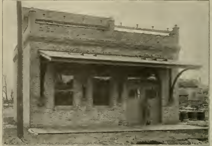
Elgin & Belvidere Electric Company—Substation at Union, Ill.
