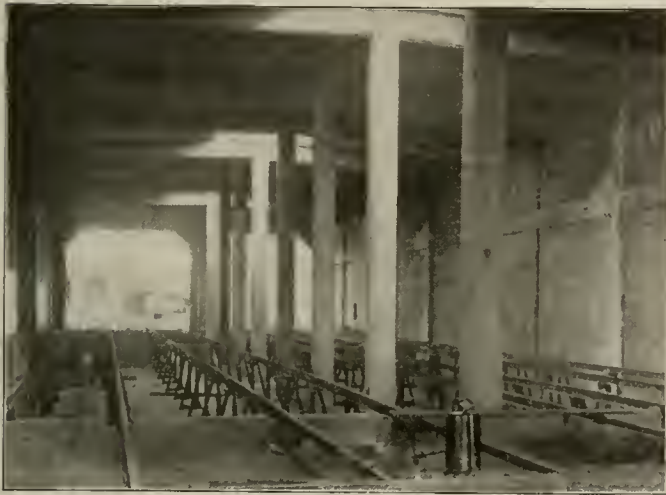
New Shops at Seattle—Interior of Inspection Shop, Showing Open Pit with Rails Supported on Cast-Iron Yokes.
