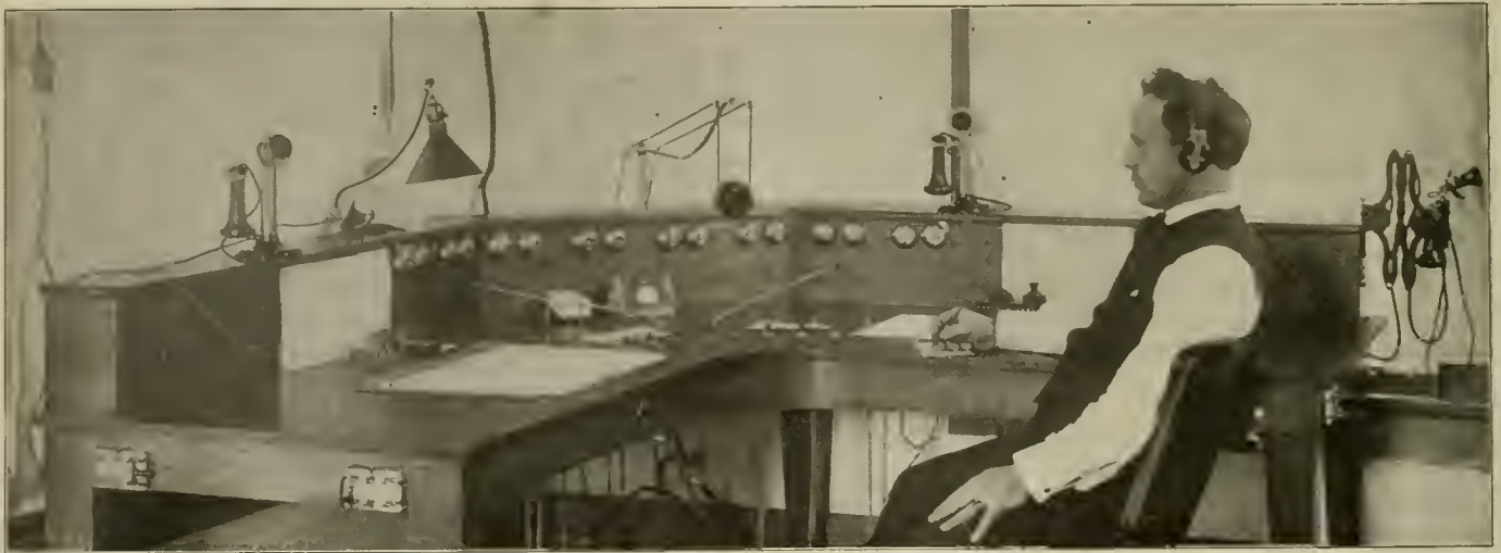
Lima & Toledo Traction Company—Dispatcher's Table and Switch-board in Office at Lima, O.
