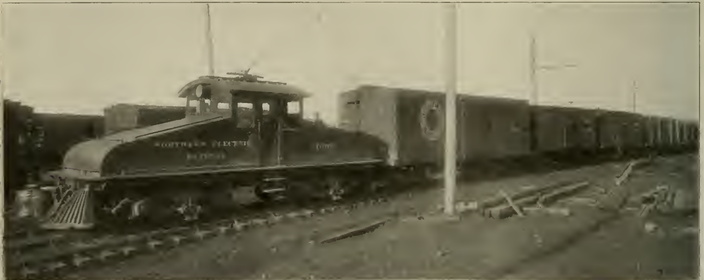
Northern Electric Railway—Locomotive with Freight Train.
