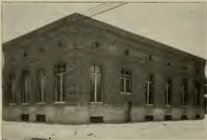
Seneca Street Substation, Buffalo—Exterior View.
