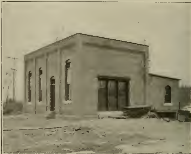
Manchester-Nashua Street Railway—Exterior Litchfield Substation.
