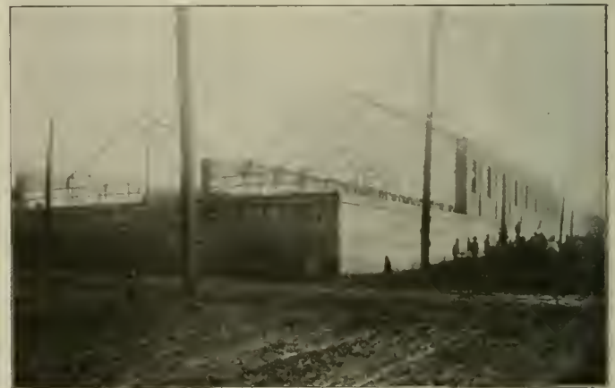
Shop Practice at Memphis—New Car Storage House with Retaining Walls.
