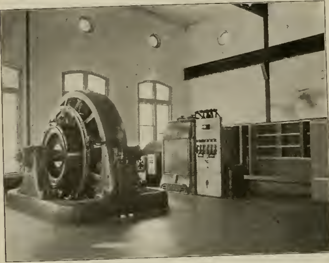
Seneca Street Substation, Buffalo—Interior View Showing 1,000-Kw. Rotary and Busbar Compartments with Doors Removed.
