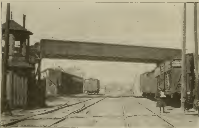
Ravenswood Extension of the Northwestern Elevated—Plate Girder Through Span over Chicago Milwaukee & St. Paul Railway.
