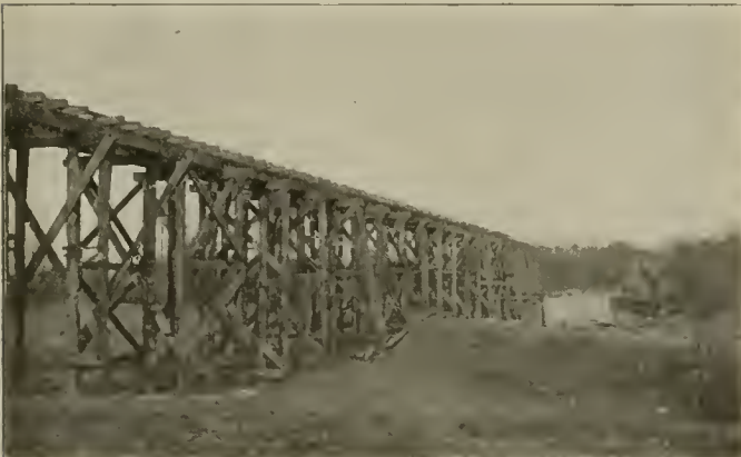
Lafayette & Logansport Traction Company—Trestle Approach to Wild Cat Bridge.
