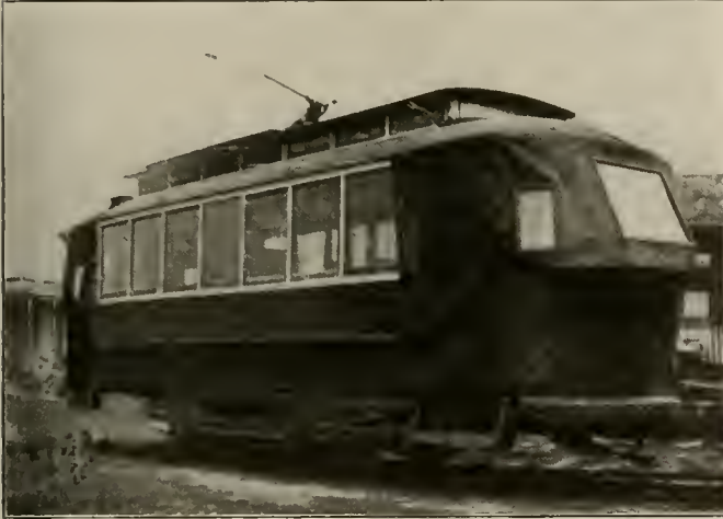
Car Equipped with Temporary Vestibule.
