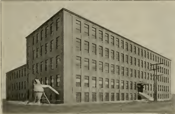
O. M. Edwards Company's Plant—Main Building.
