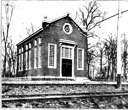
United Railways of St. Louis—Creve Coeur Substation.
