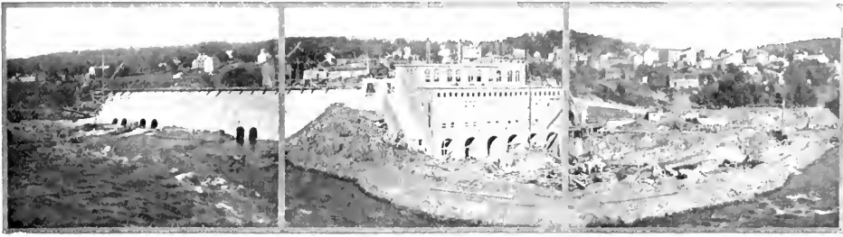
Taylor's Falls Power House and Dam.
