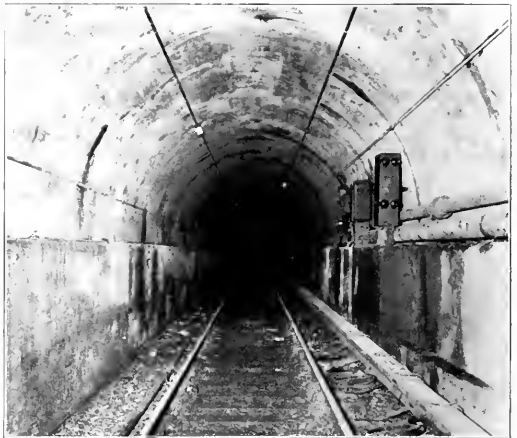
Hudson River Tunnel—First Signal Station.
