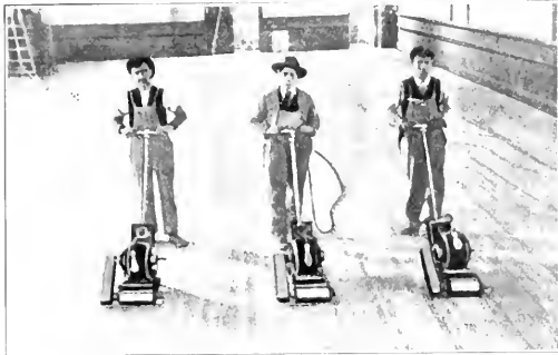
The Wattles Electric Floor Surfacers in Use.
