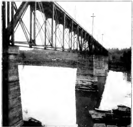
Oregon Electric Railway—Steel Deck Bridge over the Willamette River at Wilsonville.
