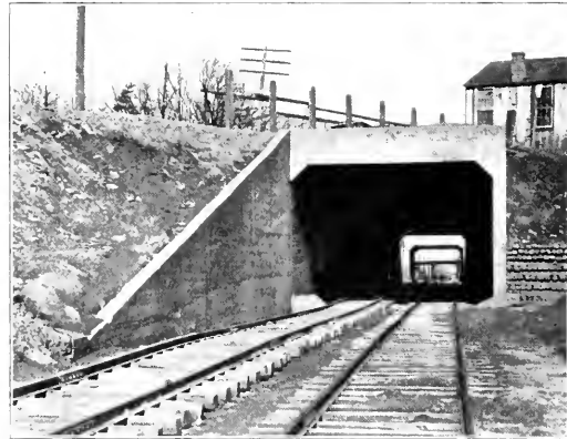
Washington Baltimore & Annapolis—Concrete Subway at Baltimore Entrance.
