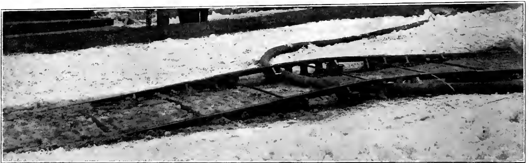
Philadelphia Rapid Transit Hose Bridge—View When in Service.
