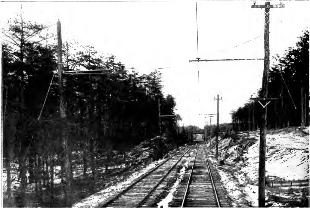
Washington Baltimore & Annapolis—Overhead Construction on Main Line.
