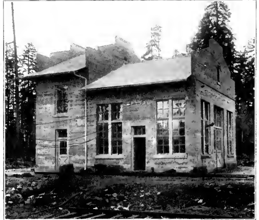
Oregon Electric Railway—Standard Concrete Substation.
