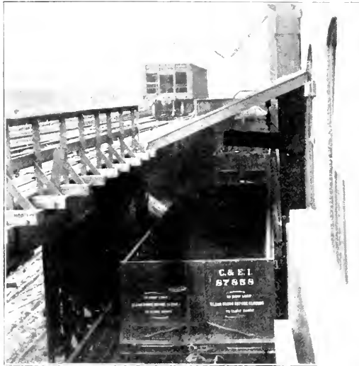
South Side Elevated Railroad—Coal Tracks in Rear of Power House.
