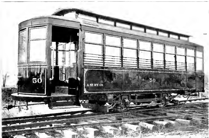
Semi-Steel Car—Amarillo Street Railway.
