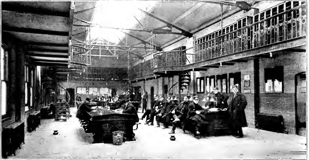
Broadway Car House, Buffalo—Trainmen's Quarters.
