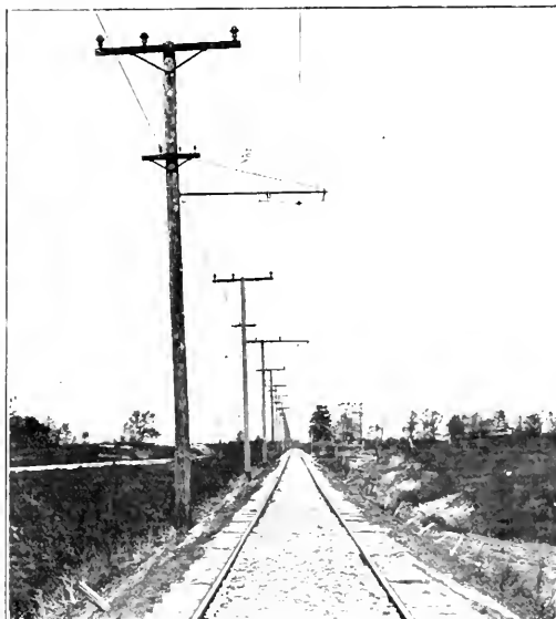
Ben-Hur Route—Track and Overhead.
