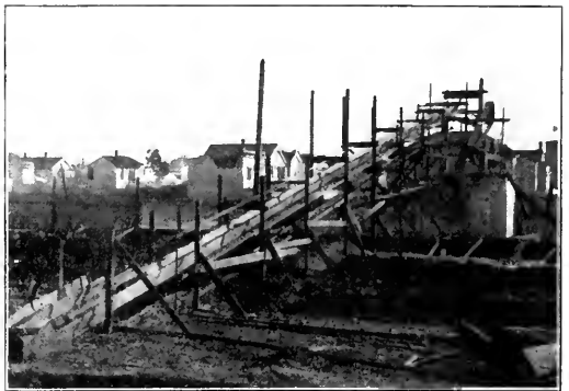
Key Route Power Station—A Simple Conveyor for Removing Dirt.
