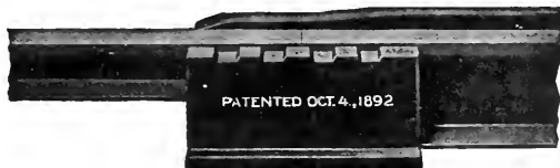
Cast Weld Compromise Rail
