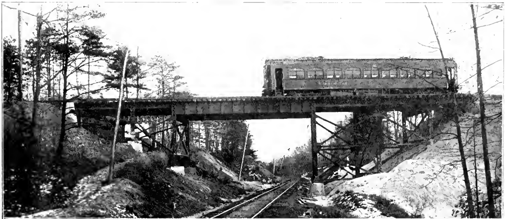
Washington Baltimore & Annapolis—Double-Track Steel Viaduct over Steam Road.
