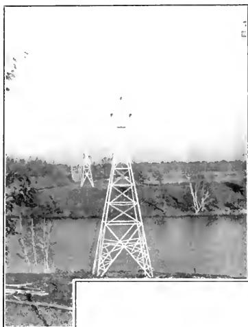
Steel Tower Construction for Long Spans
