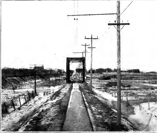
Chicago & Southern—Typical Roadway, Bridge and Overhead Construction.
