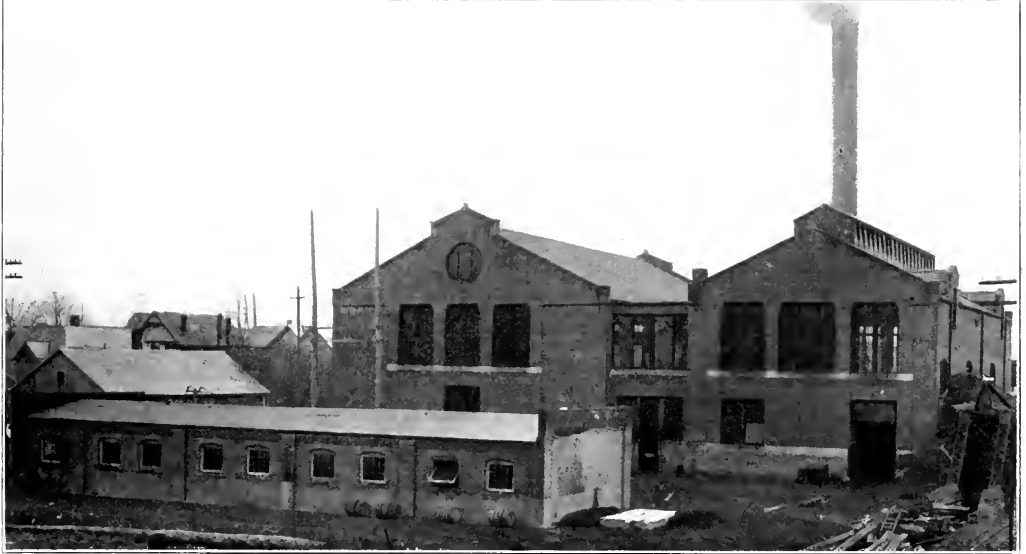
Kokomo Marion & Western—General View of Power Plant, with Storage Battery House in Foreground.
