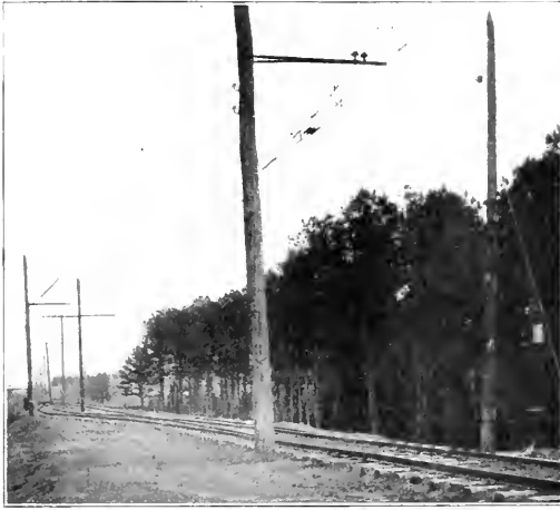
Richmond & Chesapeake Bay Railway—Catenary Construction at Turnout.
