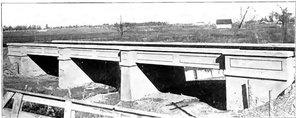
Ben-Hur Route—Flat Top Ballasted Floor Concrete Bridge.
