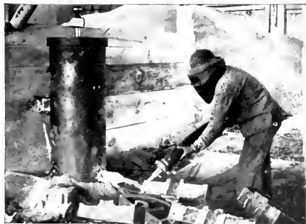
Sand-Blasting Gear Castings to remove all foreign materials from surface of steel castings.
