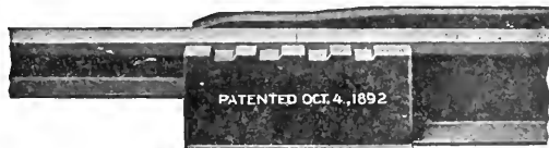
Cast-Weld Compromise Rail
