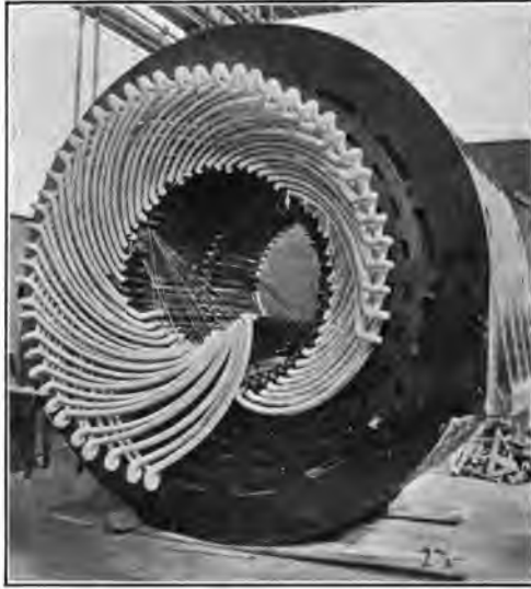
FIG. 107.—U. S. S. Tennessee : Method of Winding Generator Stator
