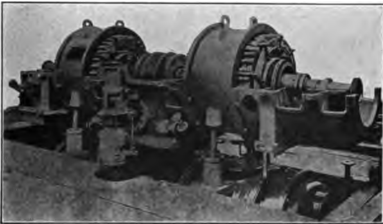
FIG. 134.— Wulsty Castle : A Ljungstrom Turbo Alternator in Course of Erection
