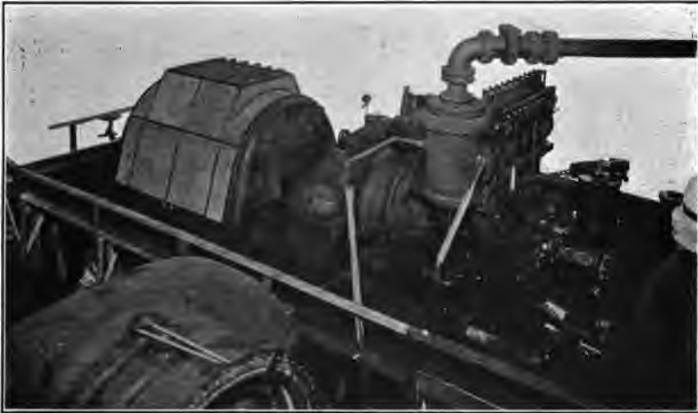
FIG. 79.—U. S. S. California : Propulsion Unit No. 2 Assembled for Test; 10-Stage Curtis Steam Turbine, 2,065 R. P. M., Direct Connected to 10,600 Kilowatt Alternating Current Generator
