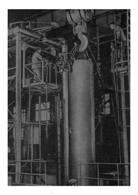
Fig. 227. Welding of two longitudinal seams.
