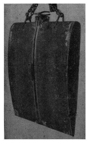
Fig. 12. Odd-shaped article welded by the electric slag process with a consumable electrode guide
