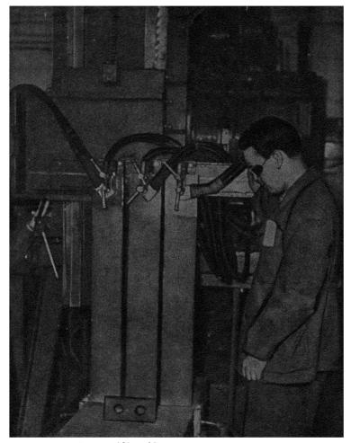
Fig. 144. Type A-480 welding apparatus using plate electrodes.
