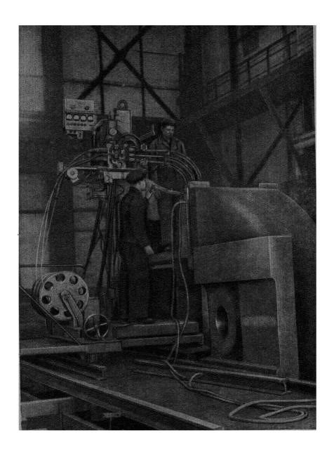
Fig. 245. Electric slag welding of the crosshead of a 6,300 ton power torging press.
