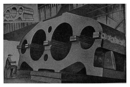
Fig. 244. Welded crown of a heavy hydraulic press.
