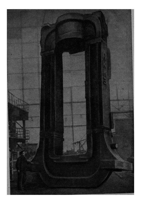
Fig. 242: Rolling mill stand welded with plate electrodes.
