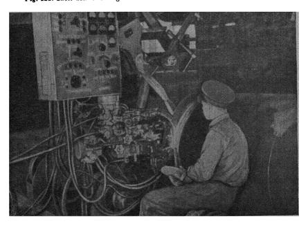
Fig. 229. Welding a girth seam.
