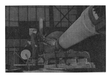
Fig. 253. Electric slag welding of a shaft for a hydraulic turbine.
