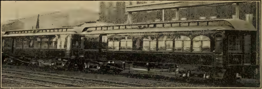
FIG. 64.—SPOKANE AND INLAND EMPIRE RAILROAD MOTOR-CAR TRAIN. The 6600-volt, 25-cycle system. Four 100-h.p. motors per 42-ton motor-car.
