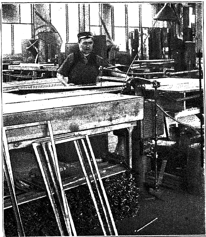
Fig. 250.—Convenient Setting of Machine for Sheet Metal Work.
