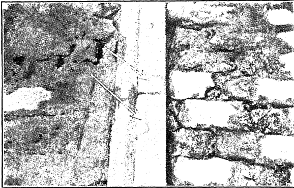
FIG. 124.—Built Up Cupped Rail Ends.
