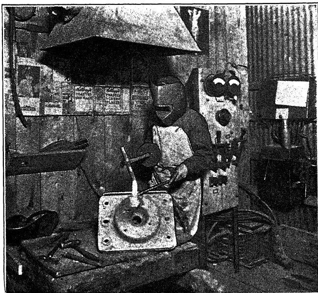
FIG. 13.—Carbon-Arc Welding, Using King Mask.
