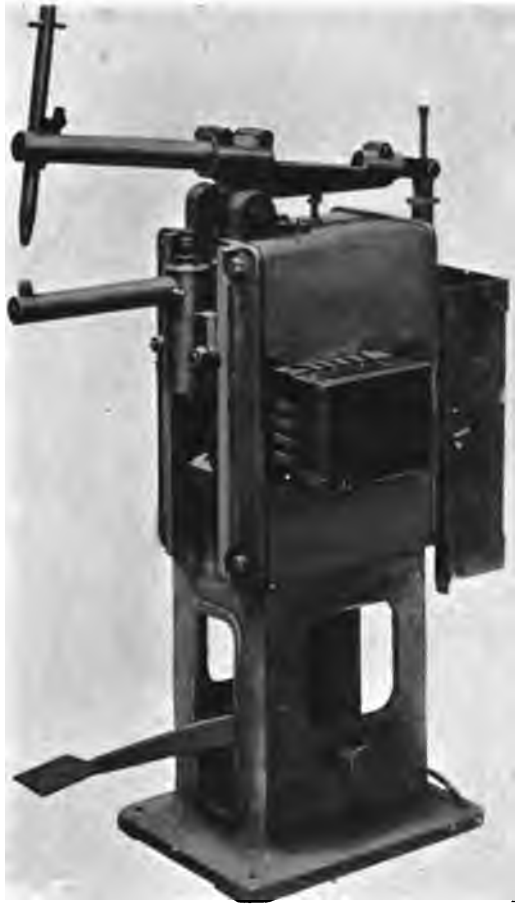
FIG. 19.—Typical Pontelec Spot Welder.
