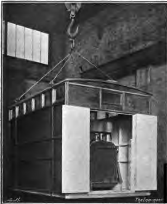
FIG. 36.—Premier Welding Set in Cabin.
