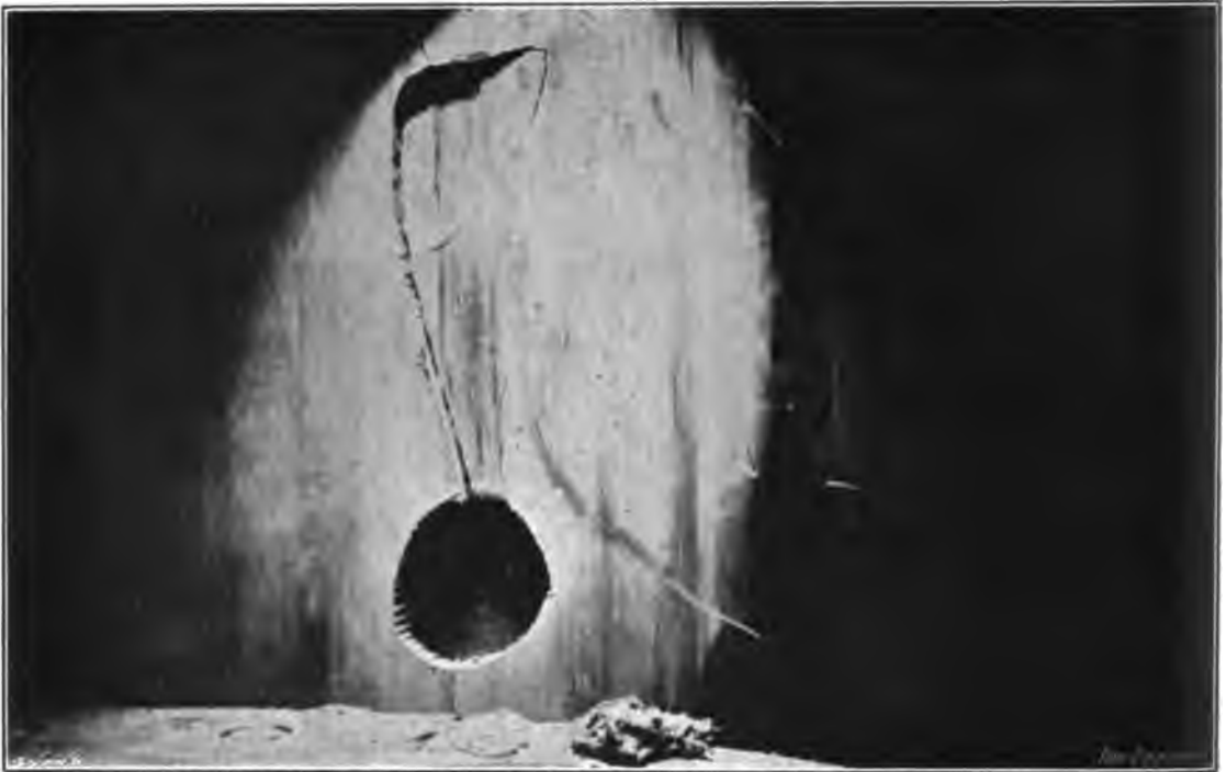
FIG. 75.—S.S. Kaiser Wilhelm II. —Fractured Low-Pressure Cylinder Liner.
