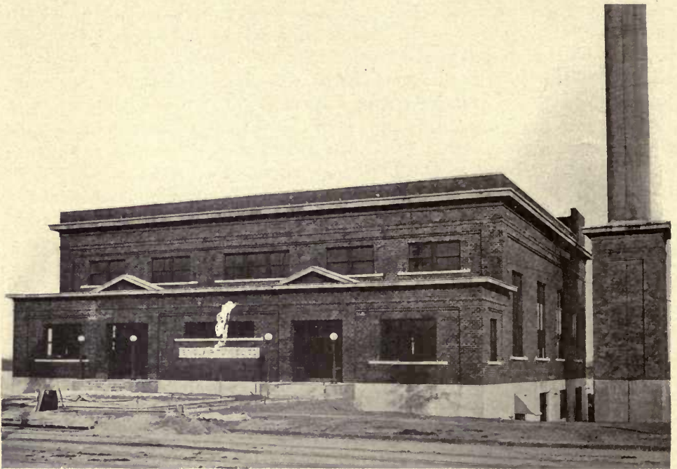
FRONT OF POWER HOUSE.
