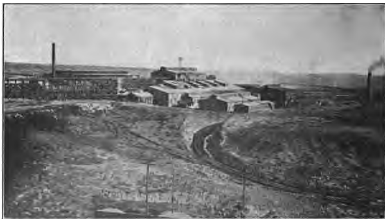
FIG. 39a.—Great Falls leaching plant
