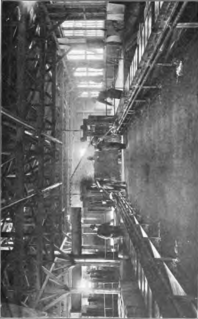
FIG. 38.—Melting and casting electrolytic zinc (Great Falls)
