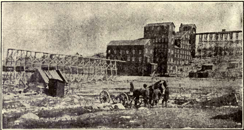
FIG. 54.—MILL AT LYON MOUNTAIN.
