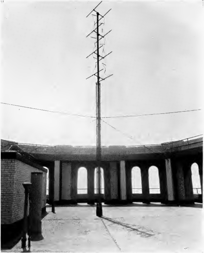
Fig. 80. Antenna Atop an Office Building in New York for Reception of Ultra-Short Waves, in the New York-Philadelphia Circuit of R.C.A.
