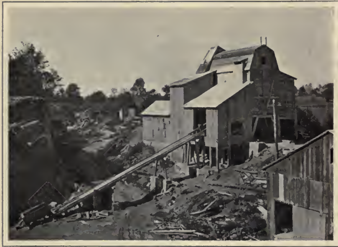
PREPARING STONE LIME.
