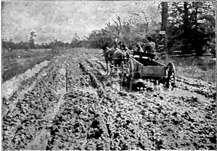
FIG. 104. Grading and draining are essential to good roads.
