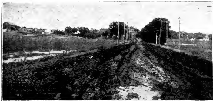
A. Typical country road after long rainy period.
