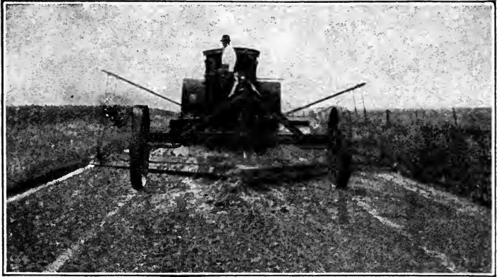
FIG. 105. Grading a country road.
