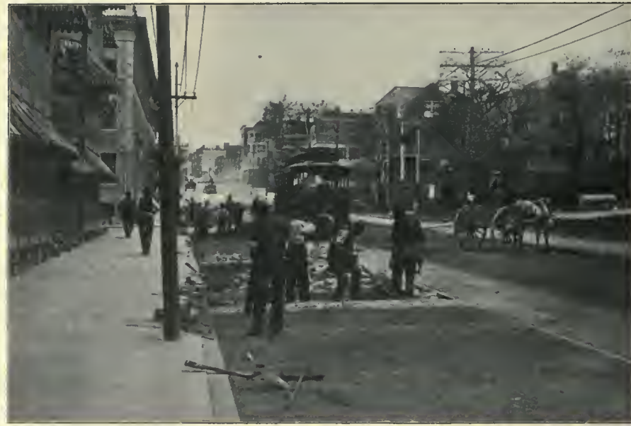
Repairing the Street
