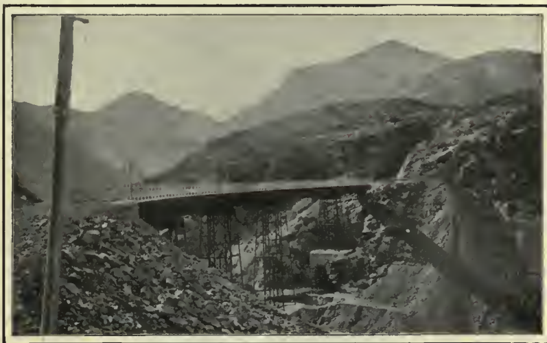
A Railroad Bridge on the Santiago Railroad in the Andes
