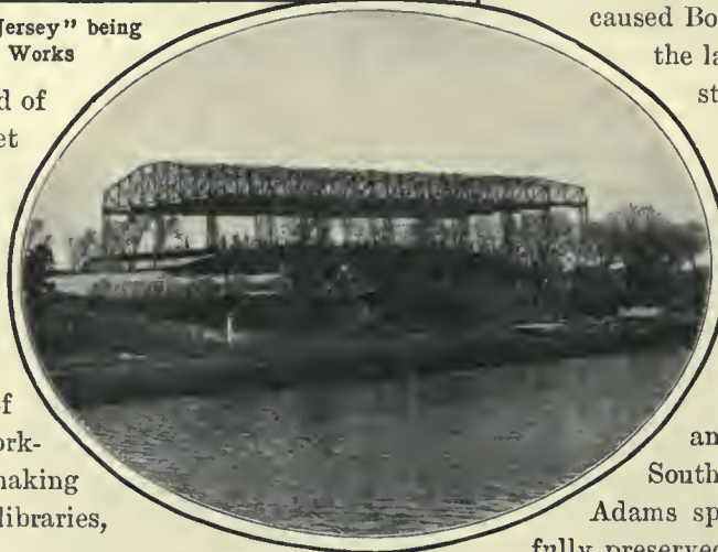
The Frame under which Large Ships are built
