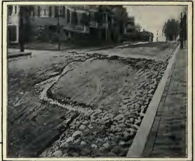
Water cutting a Channel in the Street
