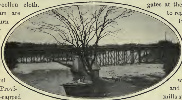
River and Canal Side by Side: Canal at Left, River at the Right
