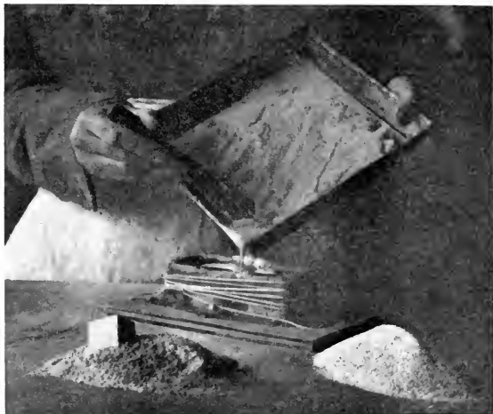
Pouring Cement Mortar into the Clay Form
