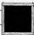
⑥ flowing a dark colored cement into the form, making the base of the tile
