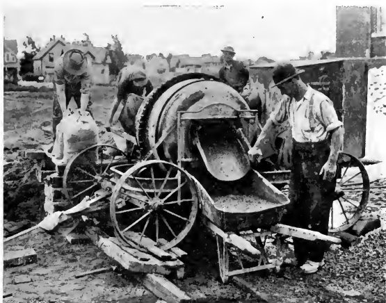
Mixing Concrete in a Rotary Batch Mixer
