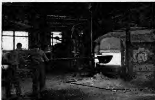
Removing a Crucible from the Furnace
