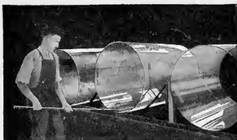
Cutting the Cylinders Lengthwise
