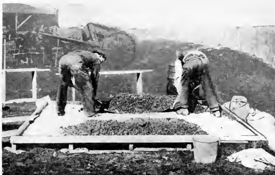
Mixing Concrete by Hand
