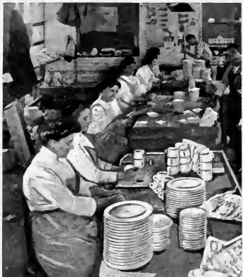
Decorators Applying Print Pattern (Transfers) in One Color
