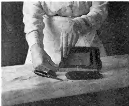
Building Outside Form Walls
