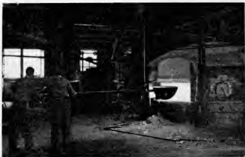
Removing a Crucible from the Furnace
