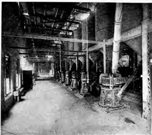
Ball Mills, Which Grind the Clinker into Portland Cement
