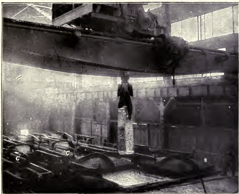
FIG. 39.—View over Tops of Soaking Pits.
