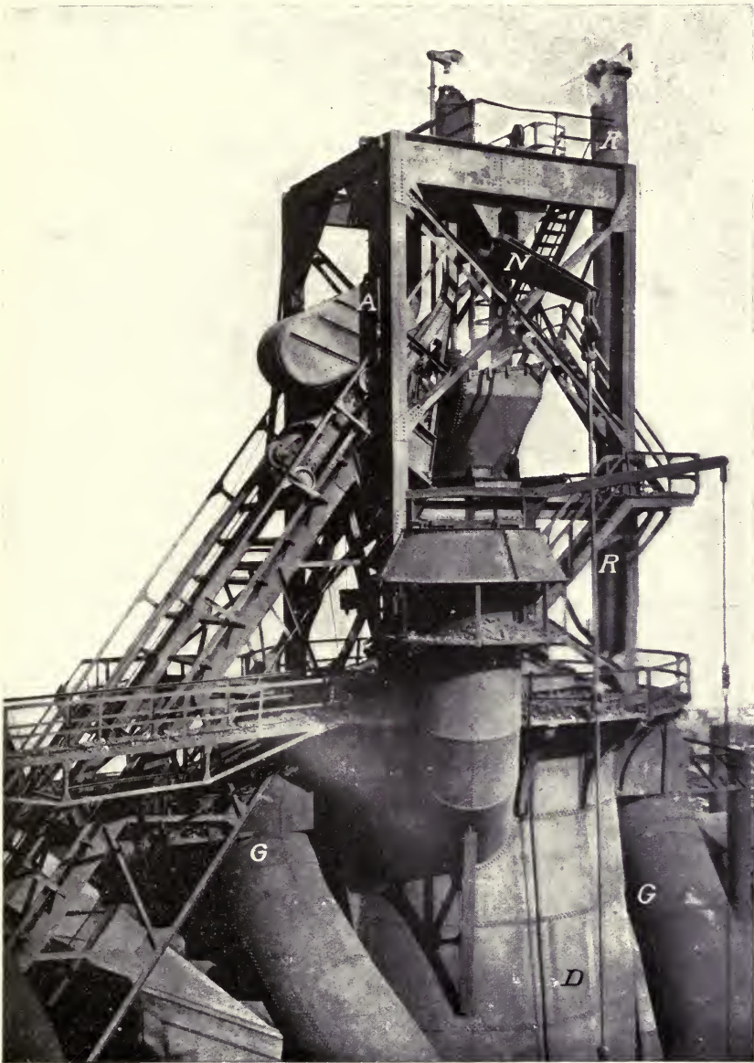
FIG. 6B.—Top of a Blast Furnace.
