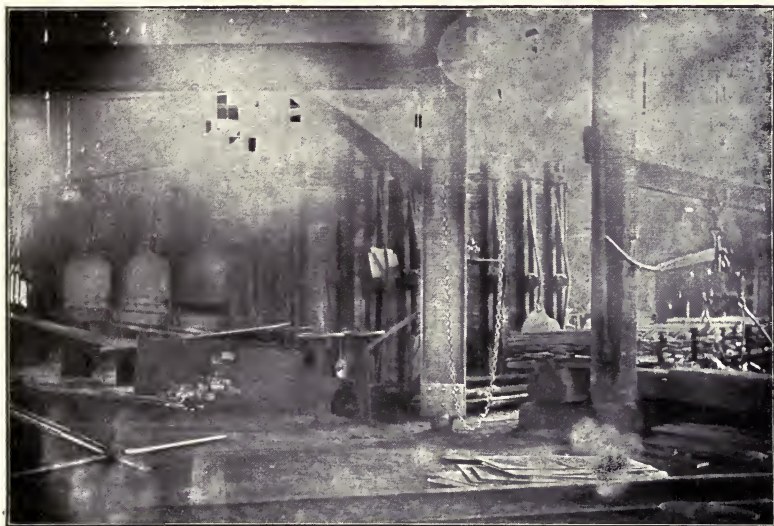
FIG. 22.—Re-heating Furnace used in Making Wrought Iron.
