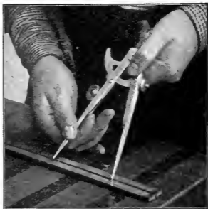
Fig. 99. Setting Compasses on a Rule.
