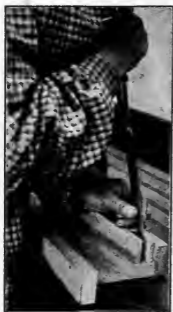
Fig. 74. Finishing the Mortise.
