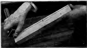
Fig. 16. Finishing a Gauge Line.
