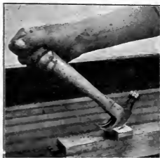
Fig. 29. Withdrawing a Long Nail.
