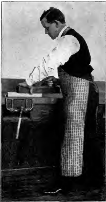
Fig. 168. Using the Wooden Jack Plane
