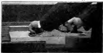
Fig. 30. Planing a Joint Flush.
