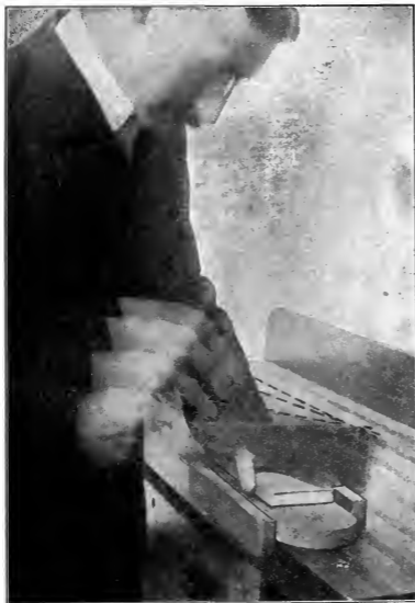
Fig. 38. Positions in Starting the Saw.
