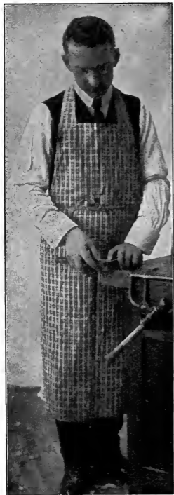
Fig. 51. Drawing Lines Across an End.
