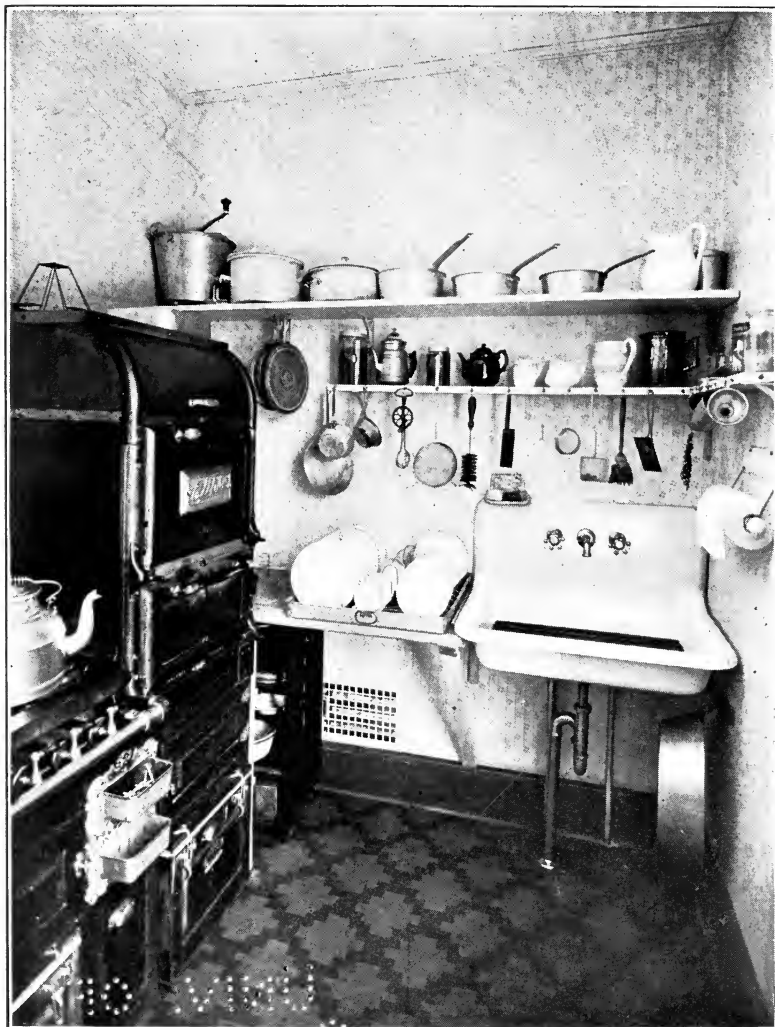
KITCHENETTE WITH GAS-RANGE.
