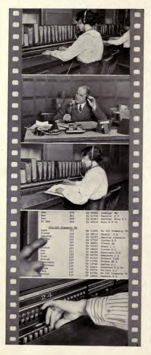
The information operator has records of telephone numbers by street address, records of listings against telephone numbers, and records showing changes in numbers or the disconnection of telephones.
