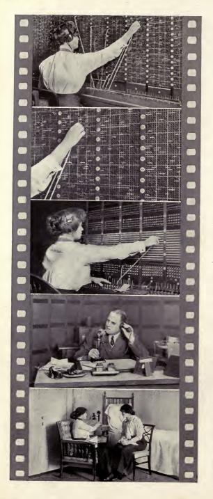
The "B" board has a long row of single cords, instead of pairs of cords, as on the "A" board. Each one of these cords is connected back through a "trunk" line to a numbered jack on the "A" board of some other central office. Each one is numbered, and each has a tiny signal lamp connected with it, which signals "B" to disconnect when "A" has disconnected.
