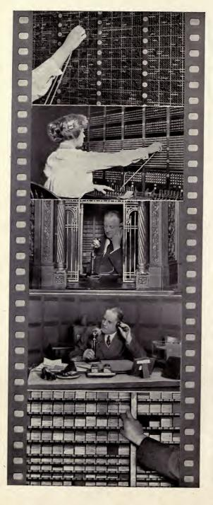
"PBX's" switchboard merely passes on outgoing calls to the "A" operator in the Spring Central Office.
