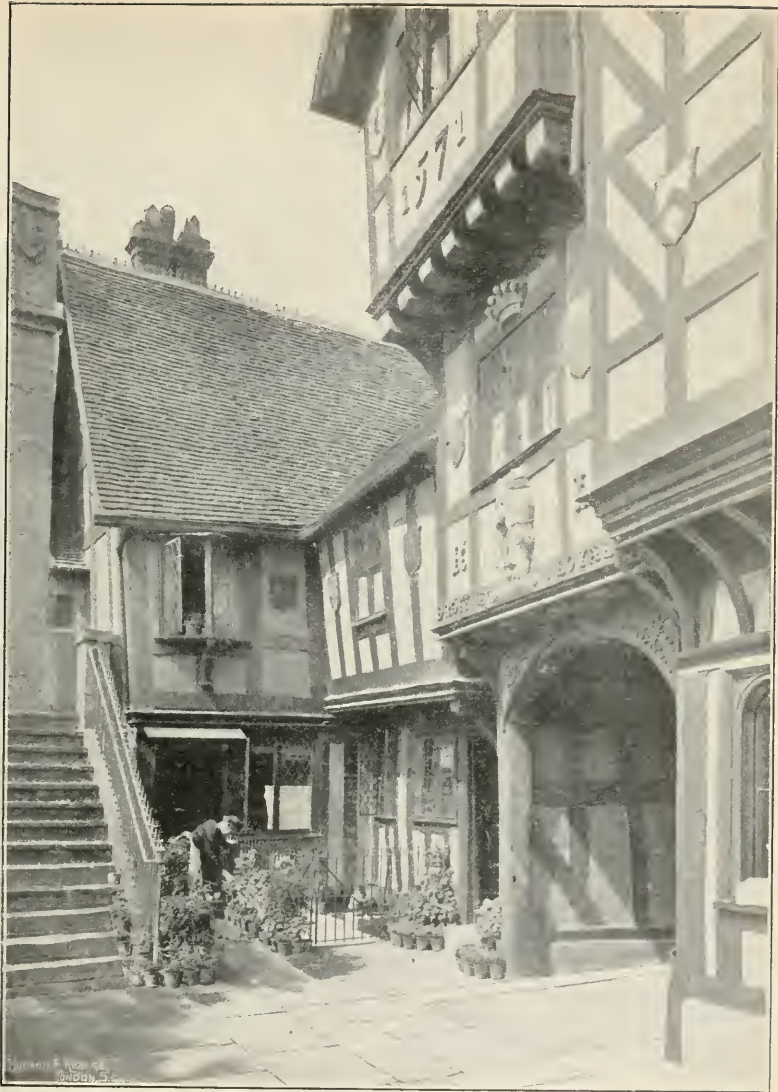
THE GATEWAY, LEICESTER'S HOSPITAL, WARWICK, ILLUSTRATING ORNAMENTAL WOODWORK AND PLASTER CONSTRUCTION.
