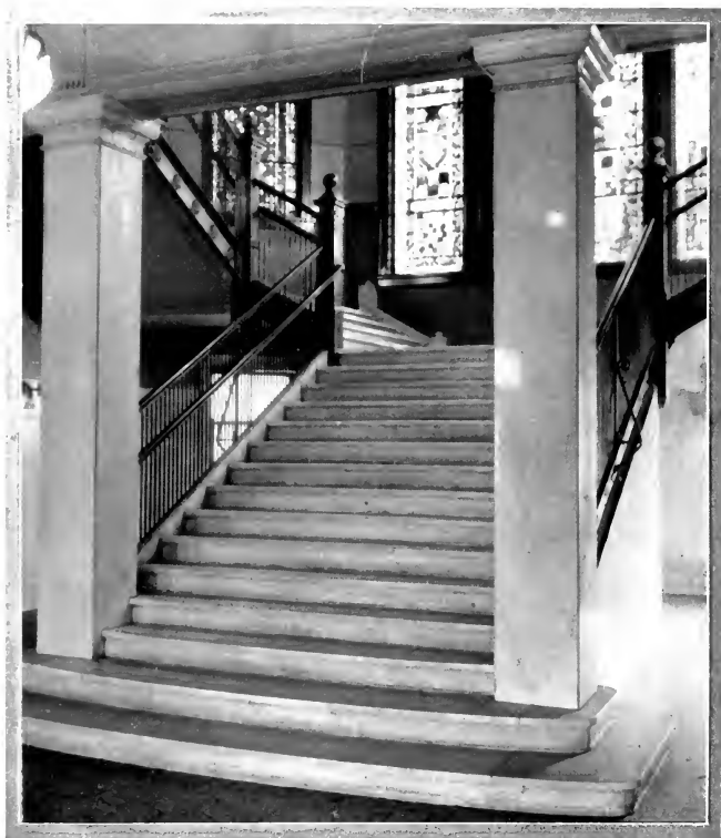
Stairway, Front Corridor
