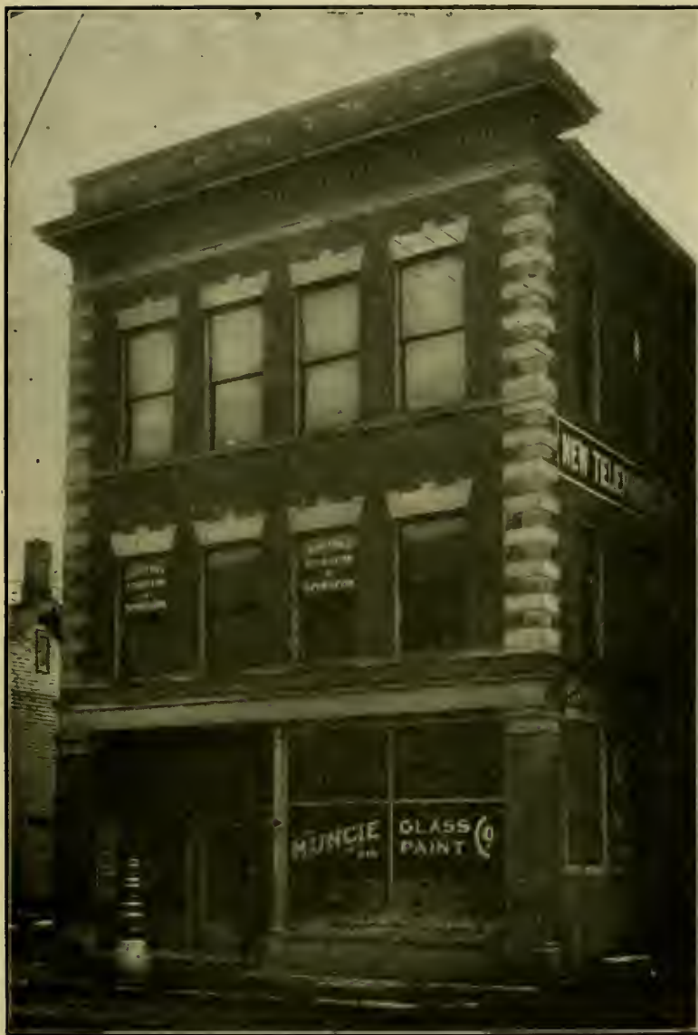
NEW D. & M. TELEPHONE BUILDING
