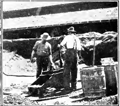
Washing old mine-filling in a rocker
