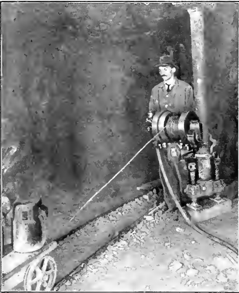
"LITTLE TUGGER" HOIST PULLING CAR IN TUNNEL
