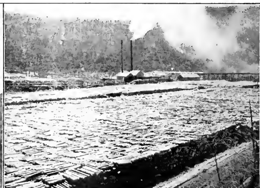
OVER 7,000 CORDS OF WOOD STORED ON THE ANDERSON LEASE FOR THAWING
