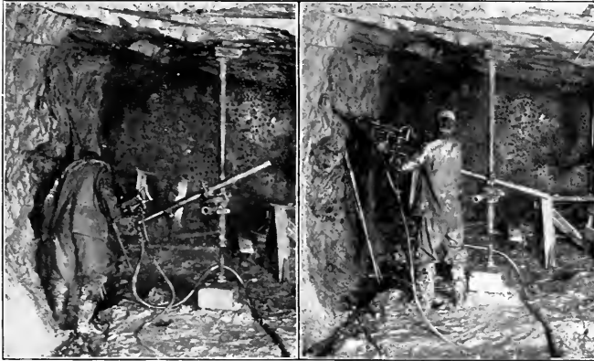
SULLIVAN AIR-FEED DRIFTER AT WORK
