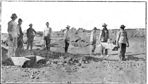
TRANSPORTING MOLTEN SLAG AND "CLEANUP" AT THE PANULCILLO PLANT
