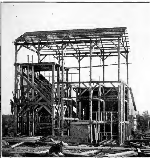
THE CRUSHER STATION IN CONSTRUCTION STAGE
