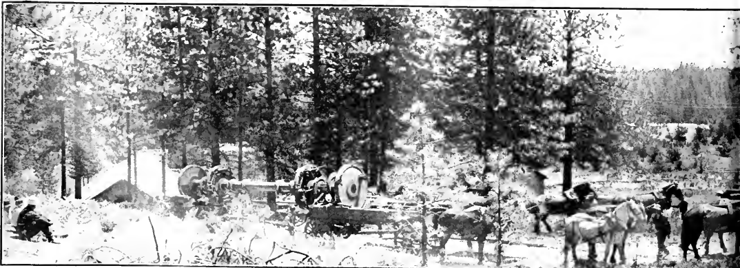
SHAFT FOR THE NEW NORDBERG HOIST AT THE CENTRAL The shaft had two disks and two clutches attached and weighed a total of 23 tons. It was 30 ft. long, drivers and six men required. The total cost
