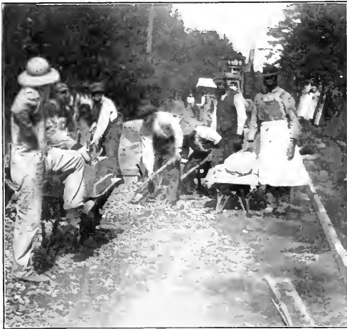
LOADING WHEELBARROW WITH CRUSHED STONE AND MEASURING LOAD AT SAME TIME
