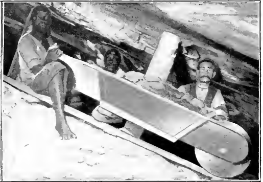
NEW SYSTEM OF CONVEYING ORE FROM FLAT STOPES OF THE RAND
