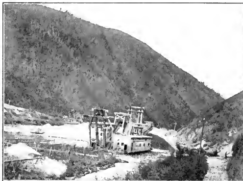
TWO DREDGES ON UPPER BONANZA CREEK; THAWING PLANT IN FOREGROUND
