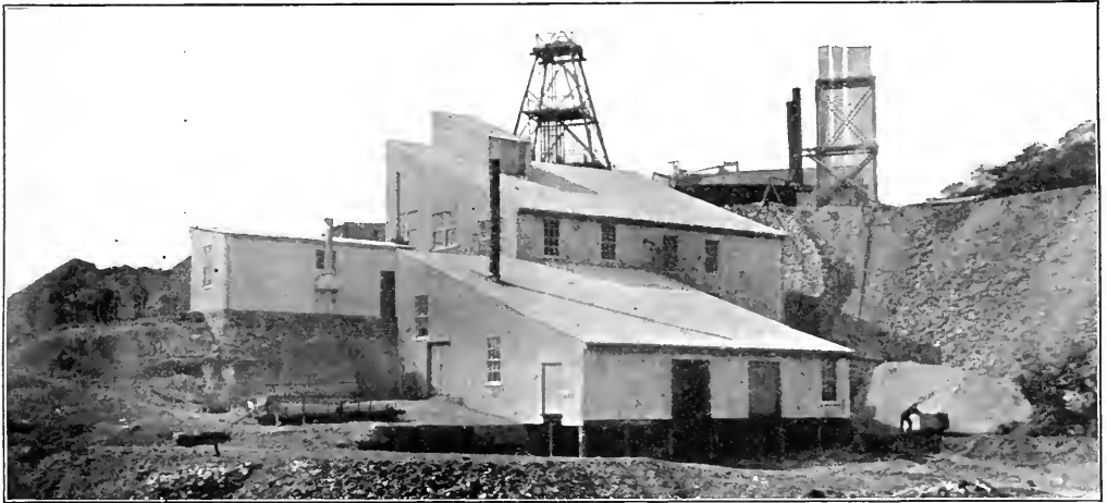
GENERAL VIEW OF THE SILVER PEAK FLOTATION MILL, VICTORIA, AUSTRALIA
