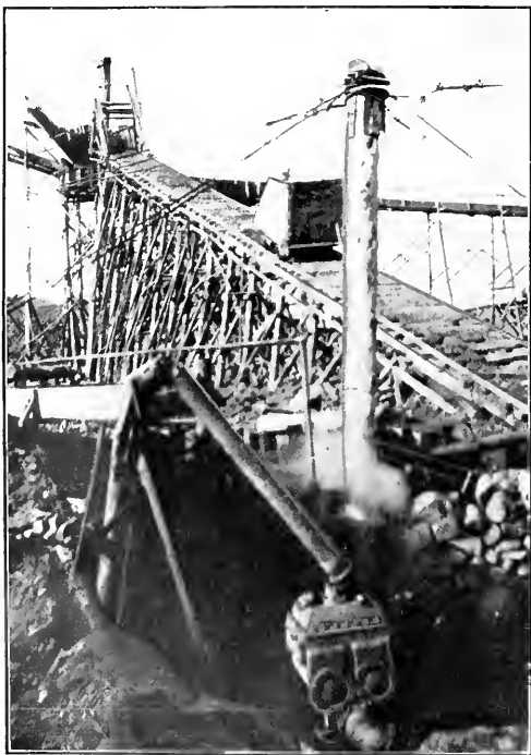
FIG. 3. INCLINED TRACK, LOADED CAR, LEAD MAST AND SEEPAGE PUMP
