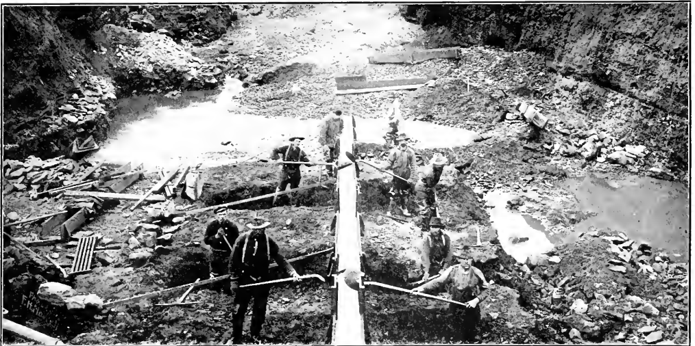
FIG. 1. SLUICING GRAVEL AT THE ALASKA FIELDS, HAND METHOD OF MOVING THE MATERIAL
