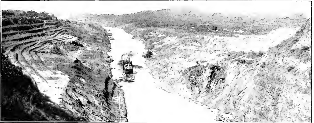
THE CULEBRA SLIDE IN AN EARLY STAGE; SLIDE FROM EAST SIDE ONLY, OCTOBER, 1914
