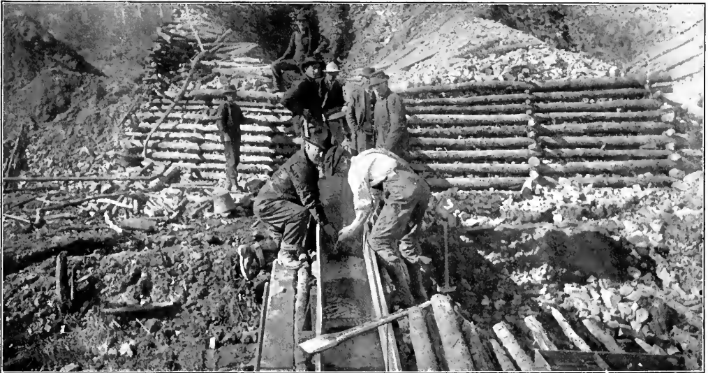
MAKING A CLEANUP AFTER SLUICING PART OF THE WINTER DUMP
