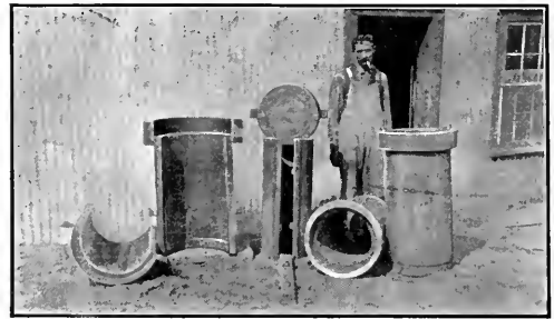
FORMS AND COMPLETED CONCRETE TILE
