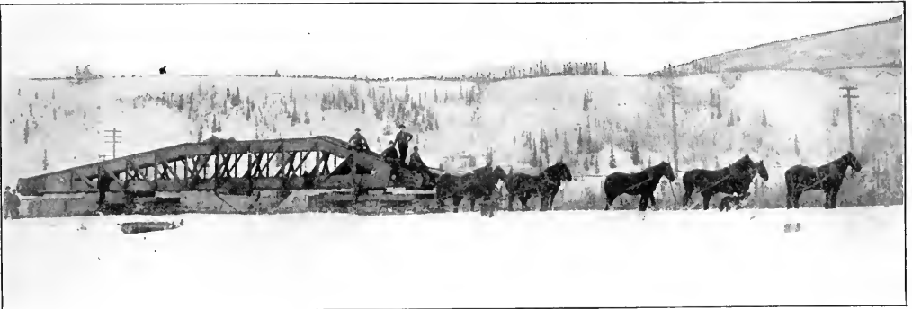
HAULING THE DIGGING LADDER OF DREDGE NO. 5 OVER A WINTER ROAD IN THE YUKON
