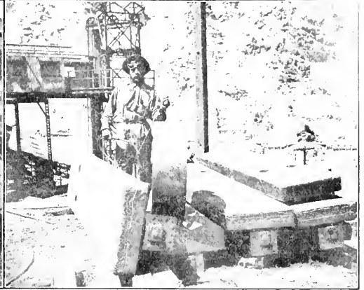
Fig. 2—Furnace jackets repaired by oxyacetylene welding
