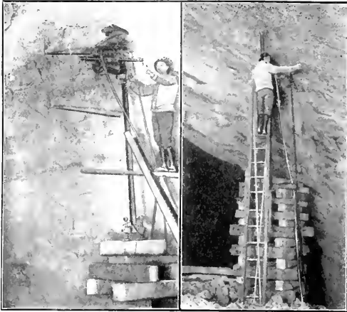
BACK STOPPING WHERE HIGH BACK REQUIRES MUCH BLOCKING AND LONG COLUMNS
