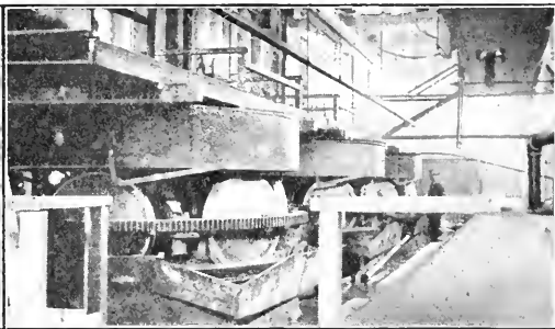
CRUSHING INSTALLATION OF LANE MILLS
