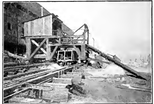
DRAG SCRAPER DIGGING AND LOADING MATTE AT ANYOX
