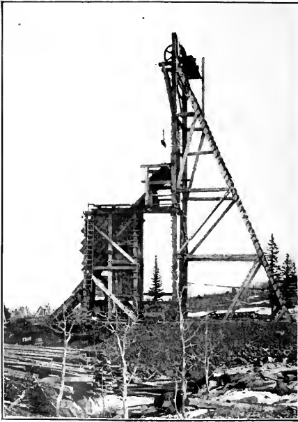
FIG. 1. SKIP IN DUMPING POSITION
