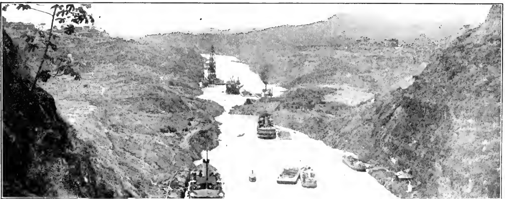
FULLY DEVELOPED CULEBRA SLIDE, AFTER AUGUST, 1915, WHEN BOTH BANKS SLID
