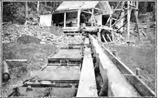
NUGGET MINE, BUTTE COUNTY, CALIF., SHOWING SLUICE AND UNDERCURRENTS
