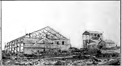
CONSTRUCTION OF TANK ROOM, CRUSHER STATION IN THE BACKGROUND
