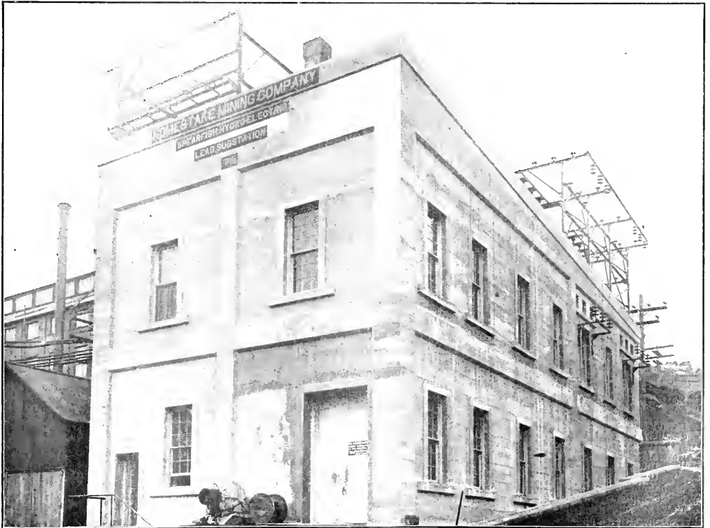
LEAD SUBSTATION OF THE HOMESTAKE MINING CO'S SPEARFISH HYDRO-ELECTRIC DEVELOPMENT
