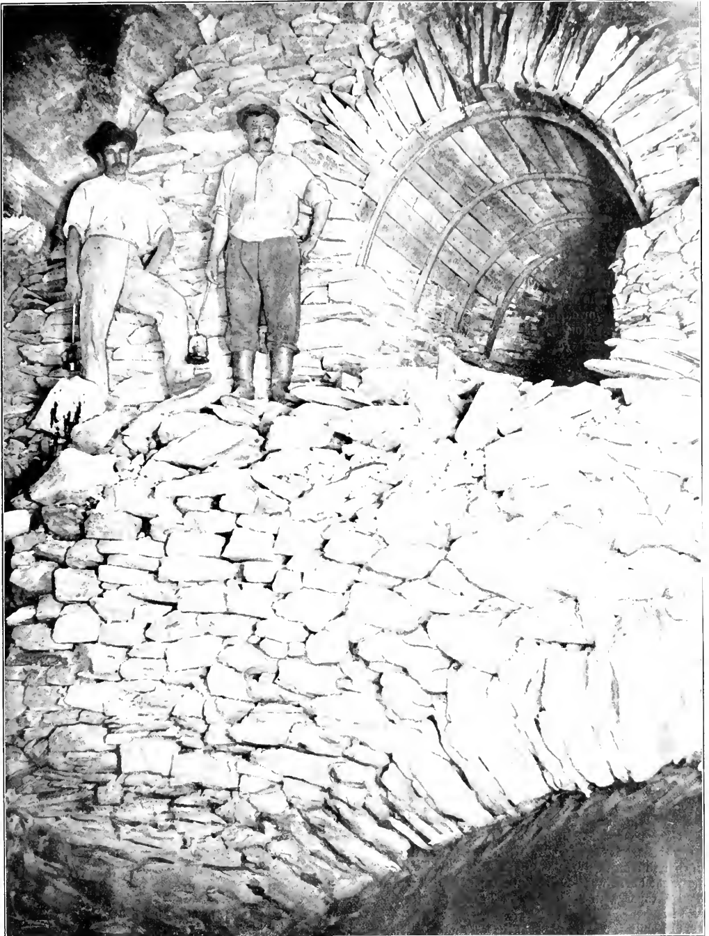
HAND FILLING OF STOPES AT THE PASSAGEM MINES OF THE OURO PRETO COMPANY, BRAZIL.
