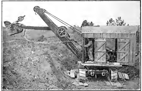
FIG. 1. REVOLVING SHOVEL WITH GASOLINE-ENGINE DRIVE
