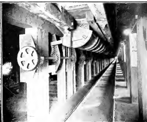
FIG. 3. BEDDED-ORE BINS WITH ARC GATES ALSO OPERATED BY THE CHARGING LARRY
