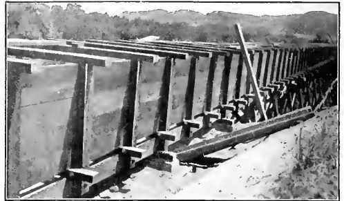
FIG. 2. VIEW OF FERNANDO FLUME, LOS ANGELES WATER-WORKS
