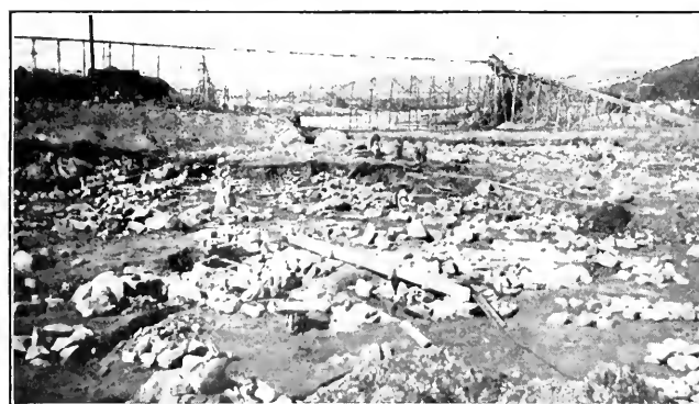
FIG. 1. CLEANED BEDROCK WITH THE SET-UP IN THE BACKGROUND
