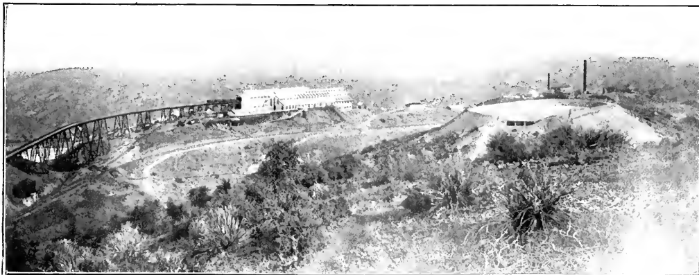
INSPIRATION CONSOLIDATED COPPER CO.'S MILLING PLANT AND RESERVOIR AT MIAMI, ARIZ.
