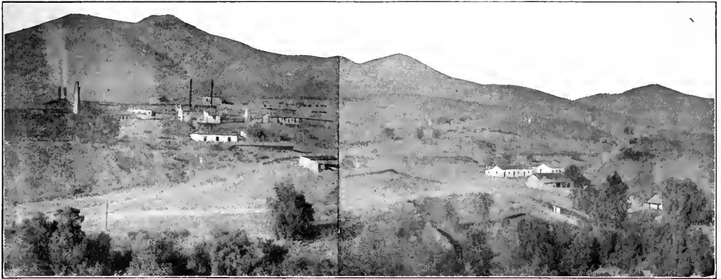
GENERAL VIEW OF CENTRAL CHILI COPPER CO. AT PANULCILLO
