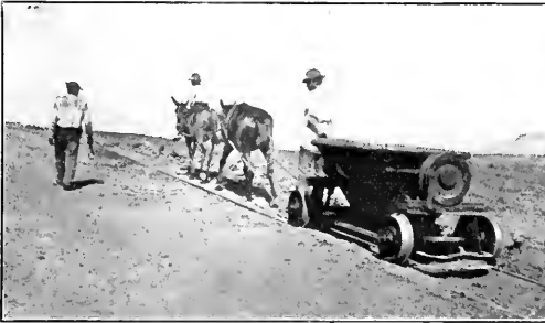
TRANSPORTING MOLTEN SLAG AND "CLEANUP" AT THE PANULCILLO PLANT
