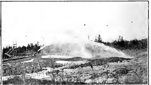
GIANTS DISTRIBUTING TAILINGS AT THE END OF THE LOGAN FLUME
