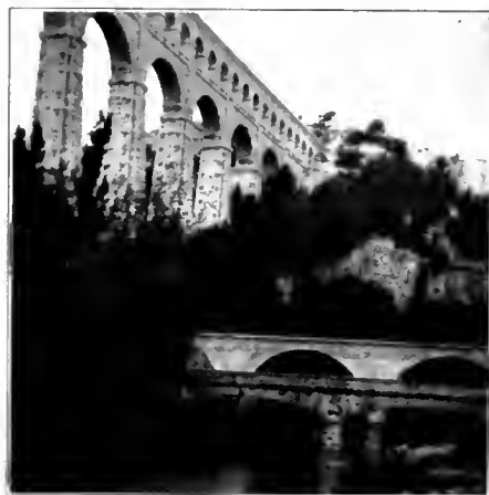
AQUEDUCT OF ROQUEFAVOUR, MARSEILLES. Early nineteenth century.
