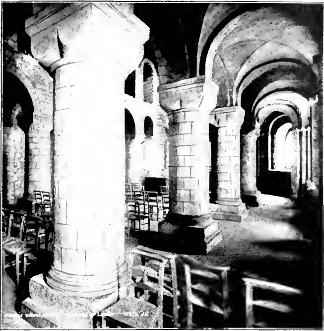
Photo, Valentine & Sons. FIG. 13.—INTERSECTING GROINED VAULTING. Early example. St John's Chapel, Tower of London.
