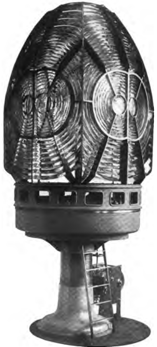
Fig. 55.—Pachena Point Lighthouse, B.C.—First Order Double-Flashing Apparatus.
