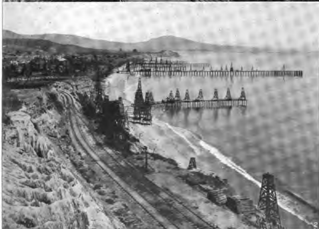
1 The Arroyo Seco ("Dry Wash"), a typical ravine between Los Angeles and Pasadena and its concrete bridge 1,460 feet long, 160 feet high 2 Oil wells in the Pacific Ocean at Summerland
