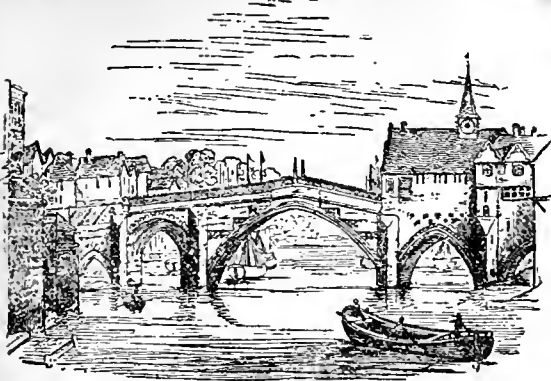
FIG. 115.—Old Bridge at York.
