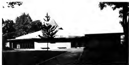
JOHN M. REEVES BUILDING, CENTENARY COLLEGE FOR WOMEN
