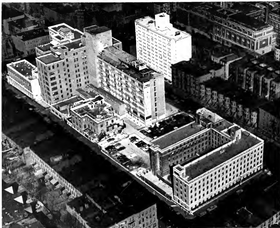
AERIAL VIEW OF METHODIST HOSPITAL, BROOKLYN, NEW YORK
