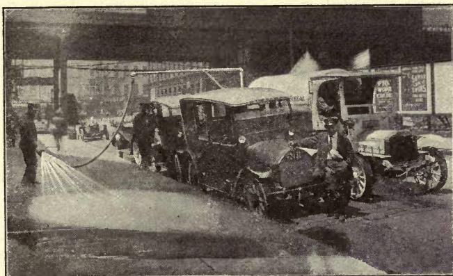
Parked Automobiles Are Not Disturbed by Sidewalk Flusher
