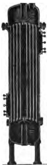
Fig. 19. The Goubert feed-water heater.
