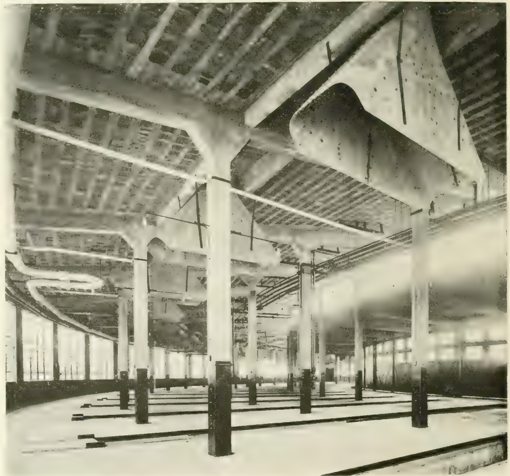
Fig. 4. Interior View of 100-ft. Roundhouse of Locomotive Terminal. Note Asbestos Smoke Jacks.
