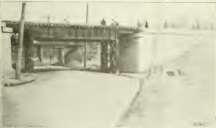
Fig. 5. Finished Roadway and a Grade Crossing Elimination.
