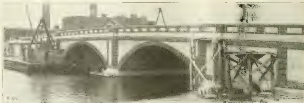
Fig. 13. View of Larz Anderson Bridge Practically Completed—Note Effective Architectural Treatment.
