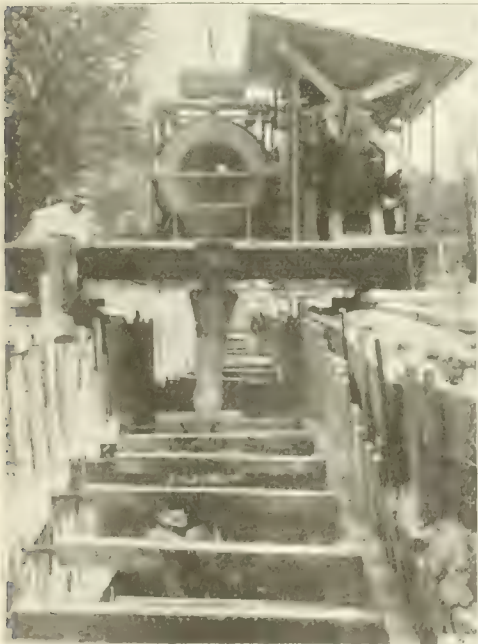
Fig. 1. View Showing Mixer Mounted on Rollers, and Flexible Concreting Chute, North Shore Intercepting Sewer Construction, Chicago.
