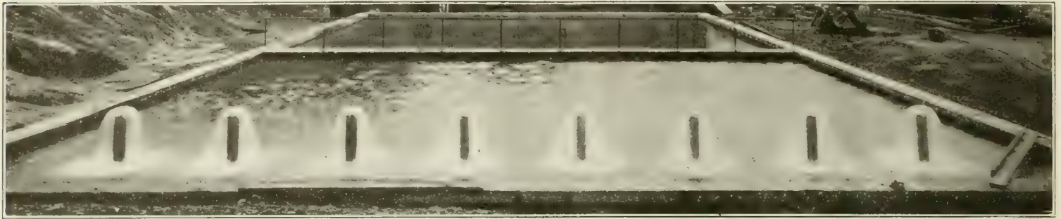
Fig. 5. Close View of New Kensington Settling Basin Showing Aerating Inlets in Operation.
