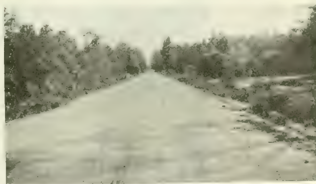
Fig. 5. Sand-Clay Roads Surfaced with Natural Sand-Clay. (Sand-Clay Mixtures Derived from Sedimentary Deposits or the Weathering of Rock in Place).
