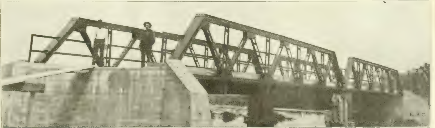
Fig. 15. Typical Riveted Low Truss Steel Bridge.
