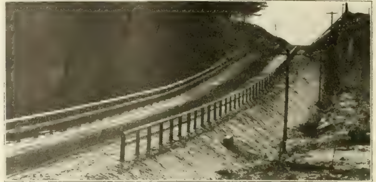
Fig. 10. Fill, Culvert and Guard Rail on a Road in Pittsfield County.
