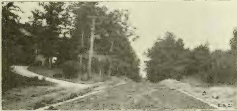
Fig. 6. Completed Pavement Covered with Earth for Protection to Concrete While Curing.
