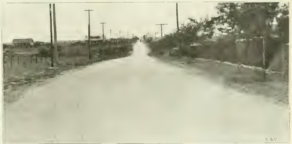
Fig. 2. An Asphalt Macadam Road Near Dallas, Texas. Surface 18 Ft. in Width.
