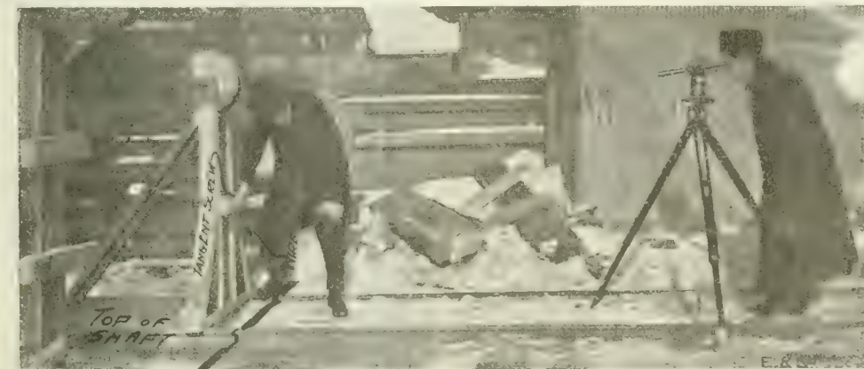
Fig. 8. Method of Alining Shaft Plumbing Wires, C. N. Ry. Tunnel at Montreal.
