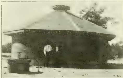
Fig. 1. Completed Superstructure of Pump Well at Atlantic City. Ten-inch Tubular Well on the Left. Edge of Old Pump Well on Extreme Right.
