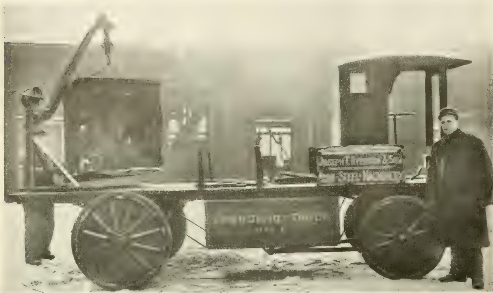
Hand Operated Derrick Mounted on Motor Truck.
