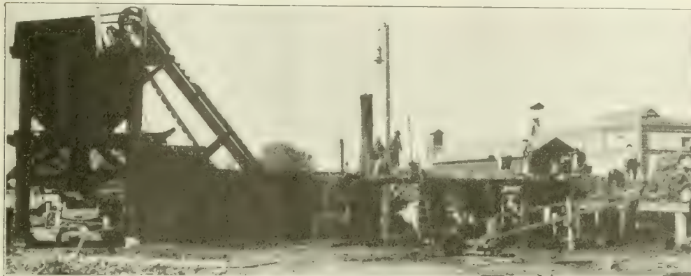
Fig. 3. Rock Asphalt Crushing Plant in Operation in Salt Lake, Utah.
