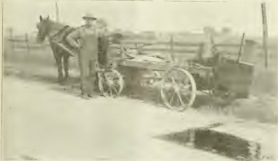
Fig. 2. Patrolman's Equipment and Method of Patching.
