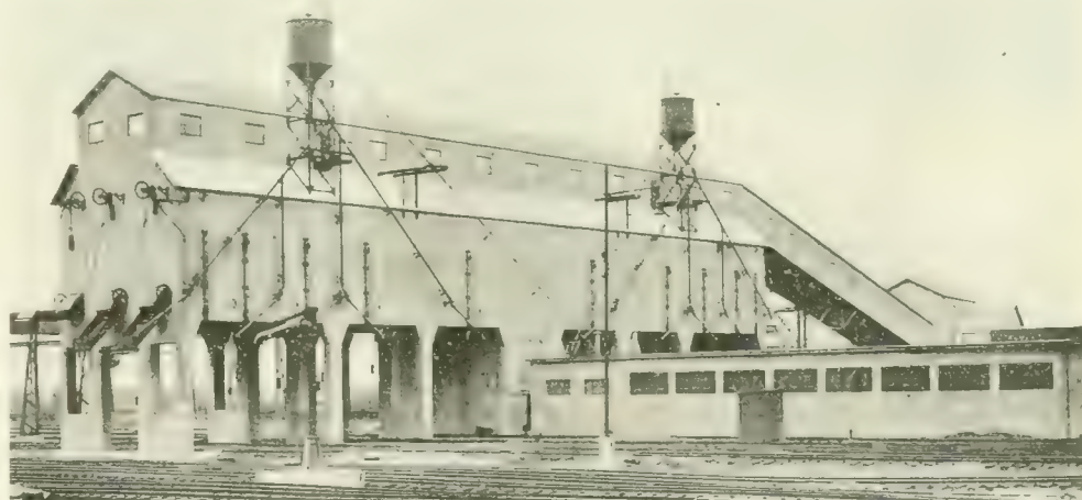
Fig. 6. View of Coaling Plant (Looking North) of Locomotive Terminal. Note Sand Storage Tanks at Top of Building.
