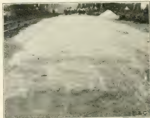
Fig. 2. View Showing the Condition of Old Surface Prior to Resurfacing.
