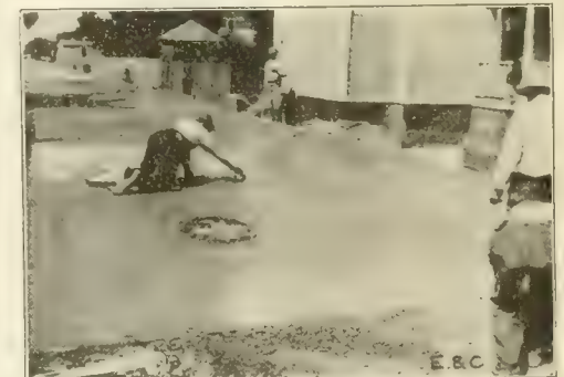
Fig. 6. Method of Floating the Surface at Intersection.
