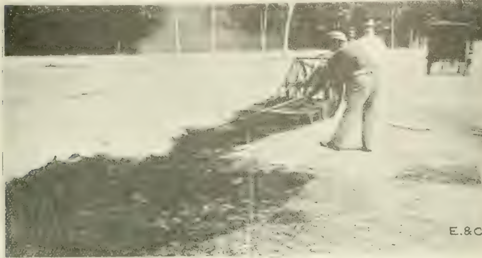
Fig. 1. View Showing Method of Operating a Hand Burner.
