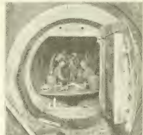
Fig. 5. View of Air Lock, Chelsea Creek Water Tunnel, Boston, Mass.
