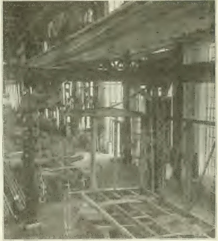
Fig. 6. View of Portion of Erecting Section of Steel Freight Car Shop of Canadian Pacific Ry.
