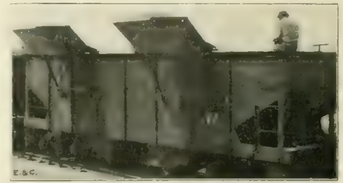
Rapid Loaders in Filling Position.
