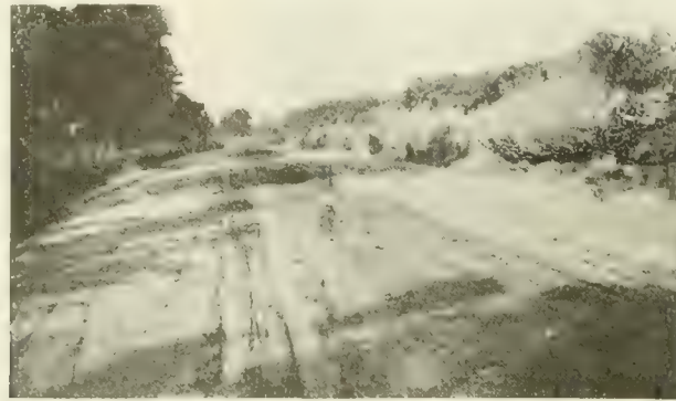
Fig. 6. Sand-Clay Roads Surfaced with Artificial Sand-Clay. (Sand-Clay Mixtures Produced by the Mechanical Mixing of Sand and Clay During Construction).
