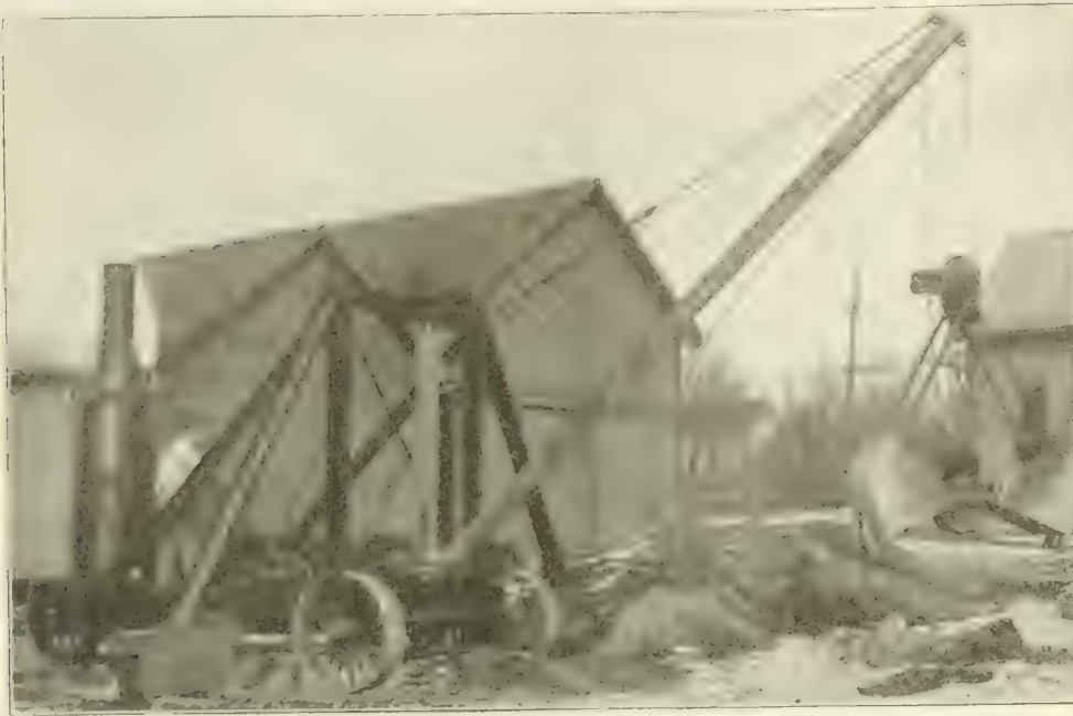
Portable Excavator for Light Excavation and Sand and Gravel Handling.
