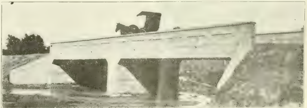
Fig. 8. Typical Concrete Girder Bridge.
