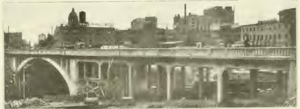
Fig. 9. View of Completed San Jacinto St. Bridge, Houston, Tex., Showing Types of Construction.
