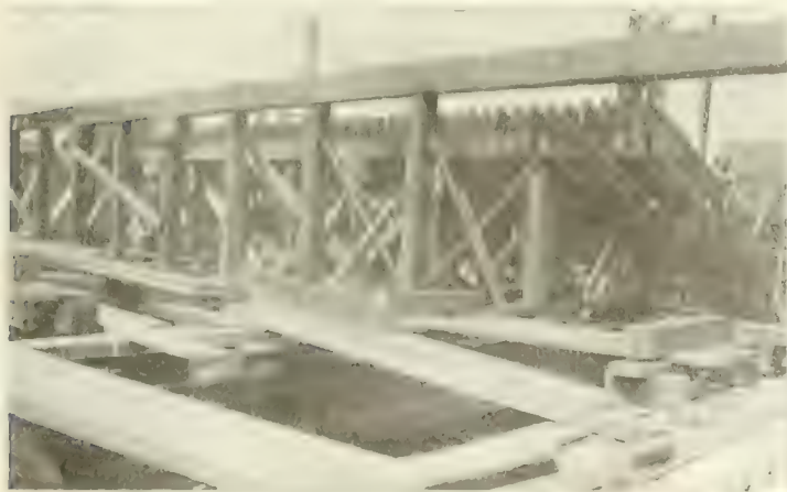
Fig. 6. View of Partially Completed Centering for 110-ft. Span of San Jacinto St. Bridge.
