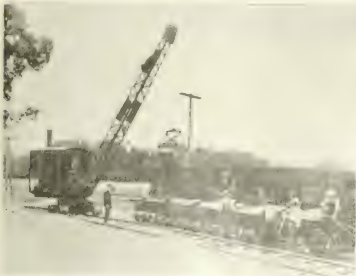
Fig. 2. Transferring Road Material from Railroad to Industrial Railway Camp.
