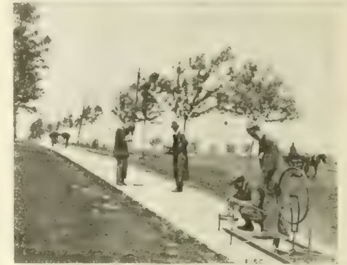
Fig. 4. Method of Measuring Base Line Showing Use of "Spiders," Bicycle Wheel, Tension Outfit and Intermediate Supports for Tape.
