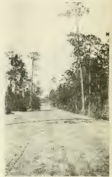
Fig. 6. Sand-Clay Roads Surfaced with Artificial Sand-Clay. (Sand-Clay Mixtures Produced by the Mechanical Mixing of Sand and Clay During Construction).
