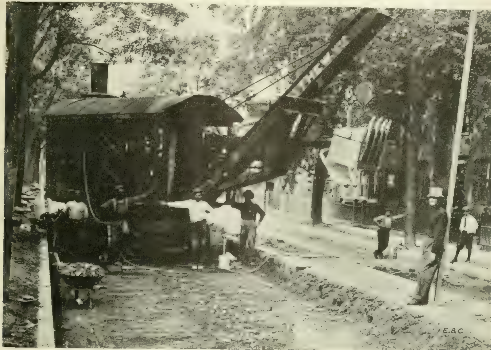
Fig 2. Steam Shovel Excavating Old Gravel Macadam.
