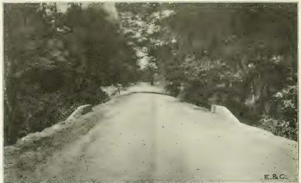
Fig. 2. View Showing Finished Surface. Note Culvert Headwalls the Full Width of the Road Apart.
