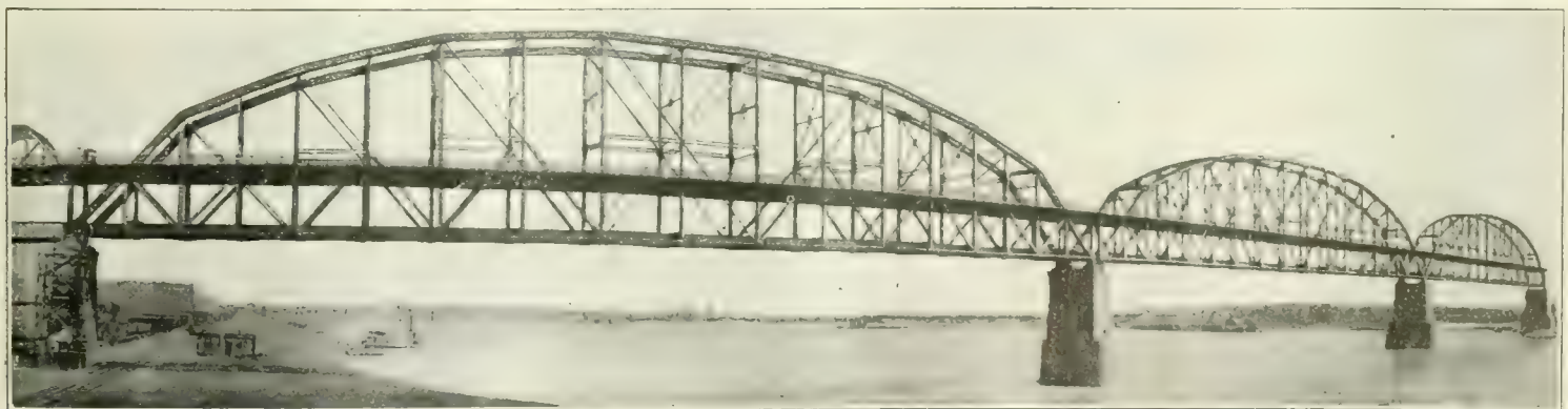
Fig. 1. View of Three 668-ft. River Spans of St. Louis Municipal Bridge Showing Type of Construction.
