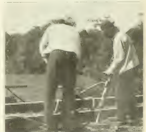
Fig. 2. View of Pair of Pneumatic Tie Tampers in Operation.
