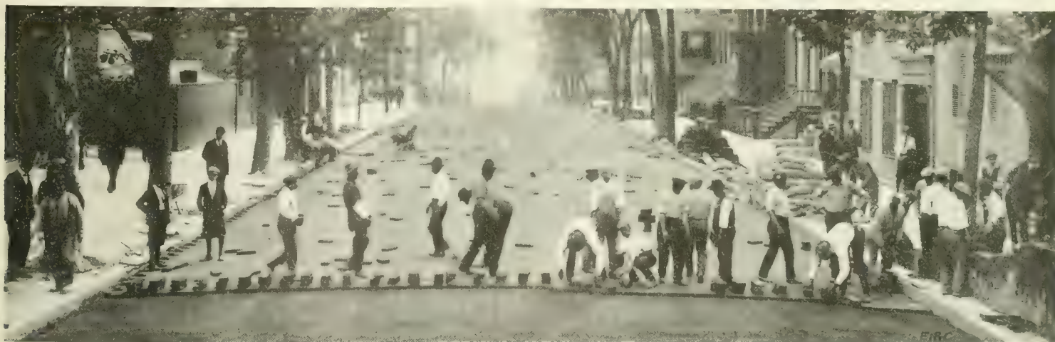
Fig. 3. Laying Asphalt Blocks at Newburgh, N. Y.
