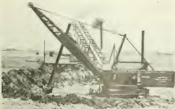
View of 3\frac{1}{2} Cu. Yd. Revolving Steam Shovel. Excavating Canal.
