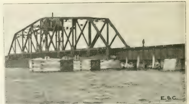
Fig. 10. View of Swing Span, Protection Works and Adjacent Girder Spans of Completed Richelieu River Bridge.
