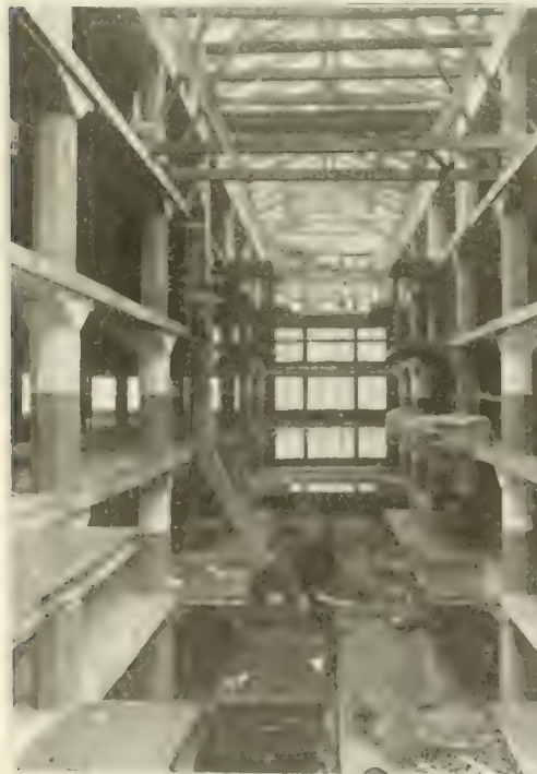
Fig. 7. View of Center Bay of Ford Motor Co. Building, Showing Floor Cantilevers, Roof Construction and Track.
