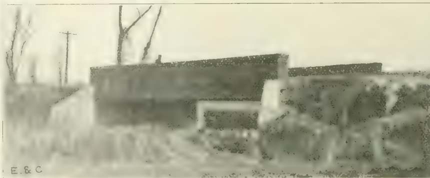
Fig. 1. Type of Concrete Girder Bridge.
