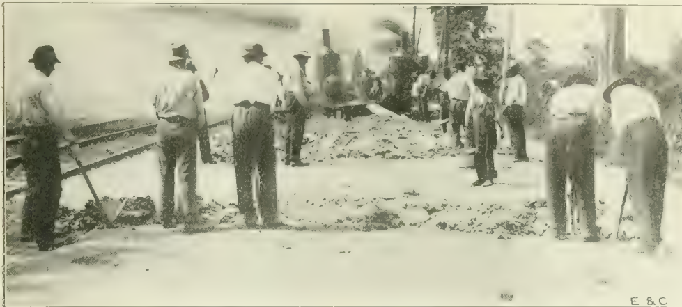
Fig. 3. Tearing Up Old Surface and Wheeling to the Mixer.
