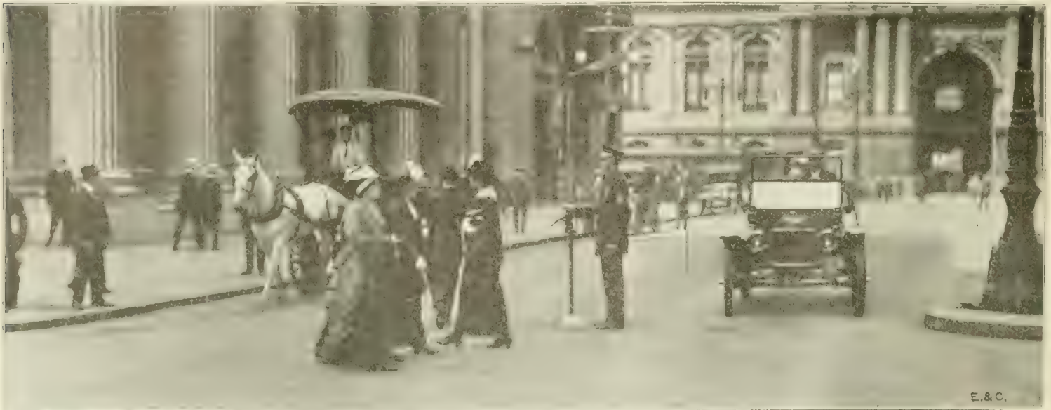
Fig. 3. Traffic Semaphore. Vehicular Traffic Closed, Pedestrian Traffic Open.
