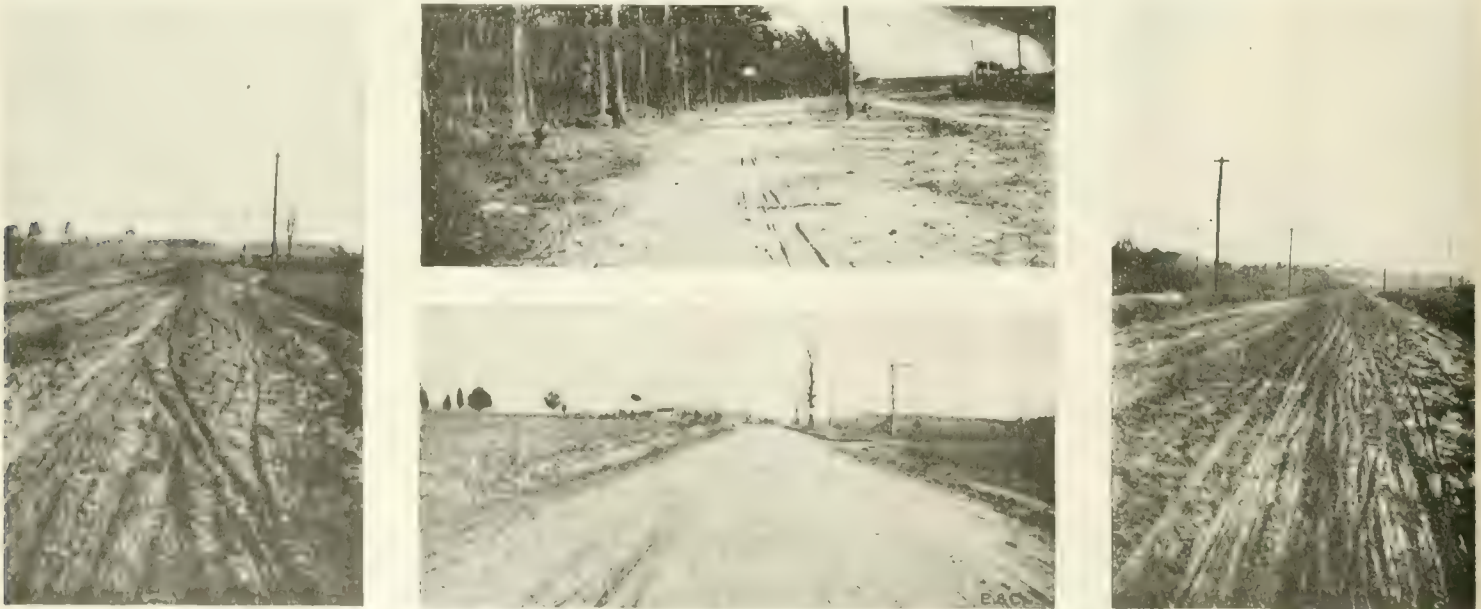
Fig. 3. Sand-Clay Roads Surfaced with Top-Soil. (Sand-Clay Mixtures Produced by the Weathering of Surface Soils).
