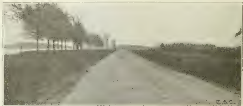
Fig. 1. Bituminous Carpet Treatment of a Road in Queen Victoria Park.
