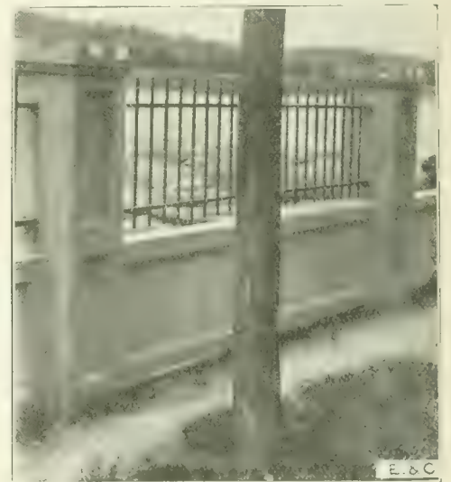
Fig. 2. View of Typical Panel of Georgetown Reservoir Fence.
