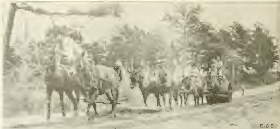
Fig. 5. Maintaining a Newly Surfaced Sand-Clay Road.
