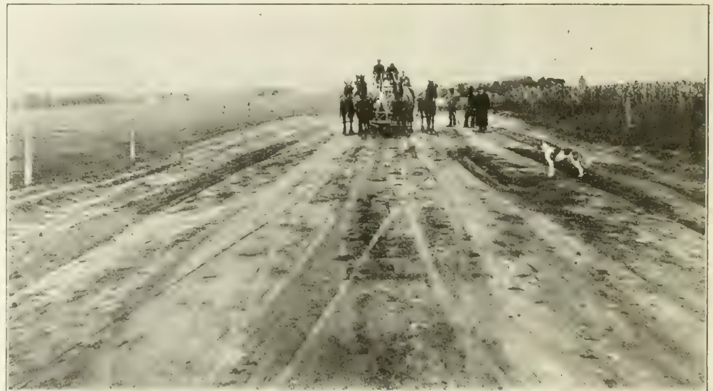
Fig. 5. Rolling Gravel Road Built to Standard Cross Section.
