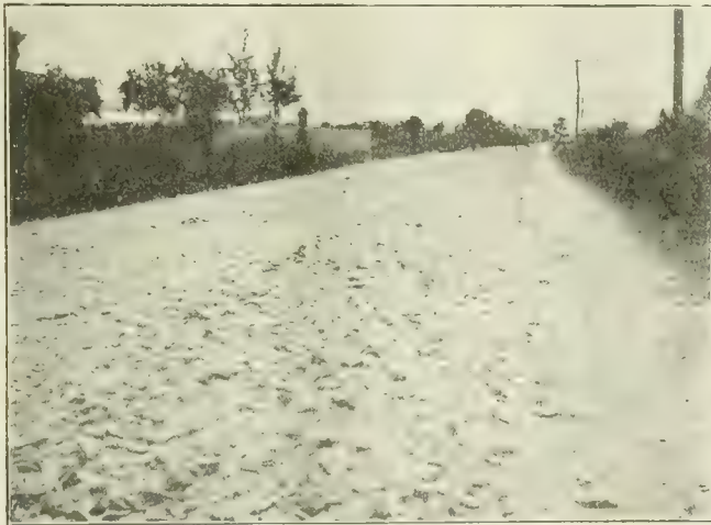
Fig. 1. Shell Surface Prepared for Surfacing.
