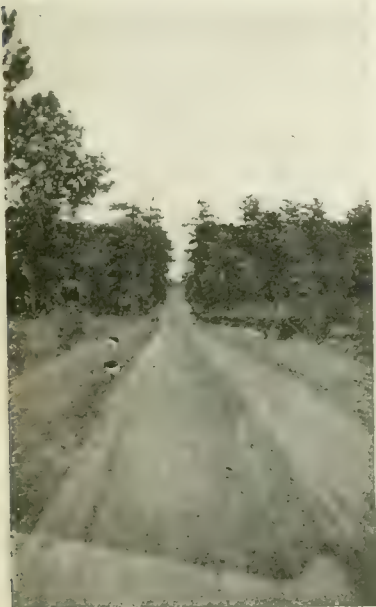
Fig. 5. Sand-Clay Roads Surfaced with Natural Sand-Clay. (Sand-Clay Mixtures Derived from Sedimentary Deposits or the Weathering of Rock in Place).
