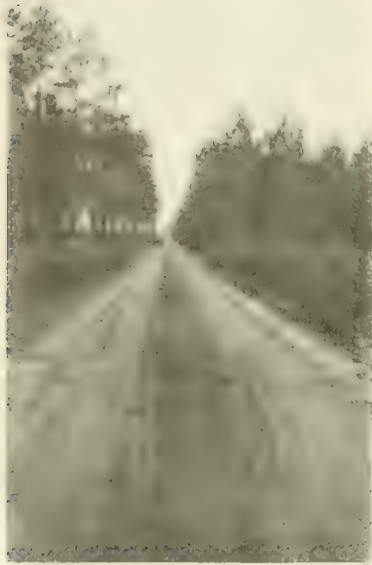
Fig. 6. Sand-Clay Roads Surfaced with Artificial Sand-Clay. (Sand-Clay Mixtures Produced by the Mechanical Mixing of Sand and Clay During Construction).
