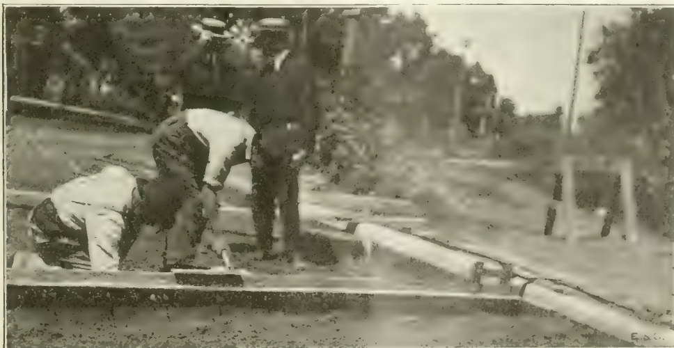
Fig. 4. Method of Setting Transverse Expansion Joint.
