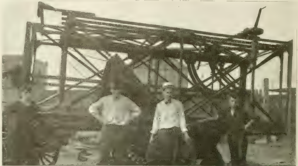
Concrete Hoisting Tower With Telescopic Sections, for Easy Transportation.
