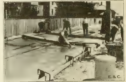
Fig. 4. Method of Constructing Curb.
