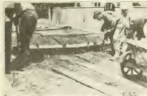
Fig. 5. Method of Placing Expansion Joint.
