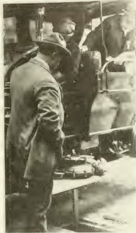
View of Motor Truck Attachment for Rapid Closing of Large Gate Valves.
