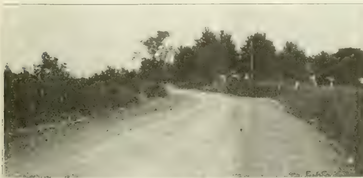
Fig. 7. Typical Limestone Macadam Road 9 Ft. Wide in Argyle County.
