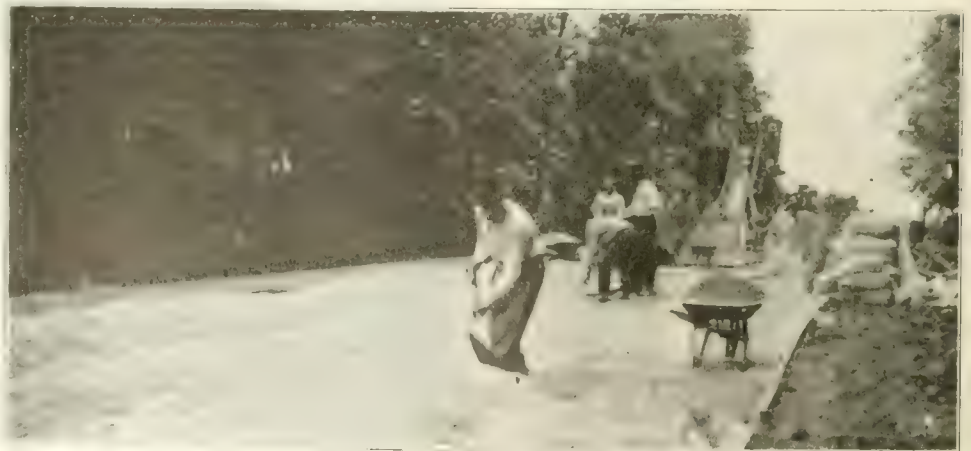
Fig. 5. Distribution of Sand and Gravel on Subgrade Ahead of the Mixer.
