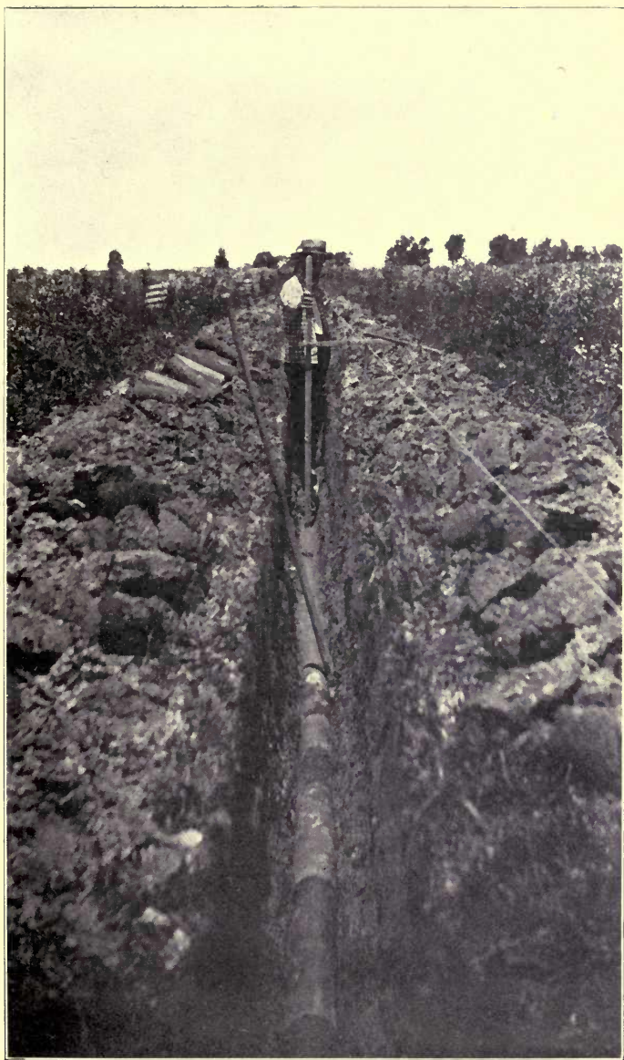
A FOUR-INCH LATERAL DRAIN.
