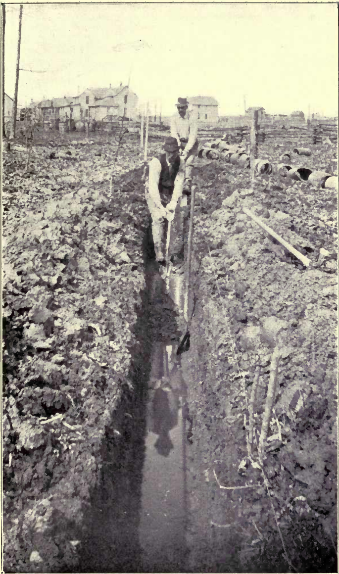
DIGGING A DITCH FOR TWELVE-INCH DRAIN-TILE.
