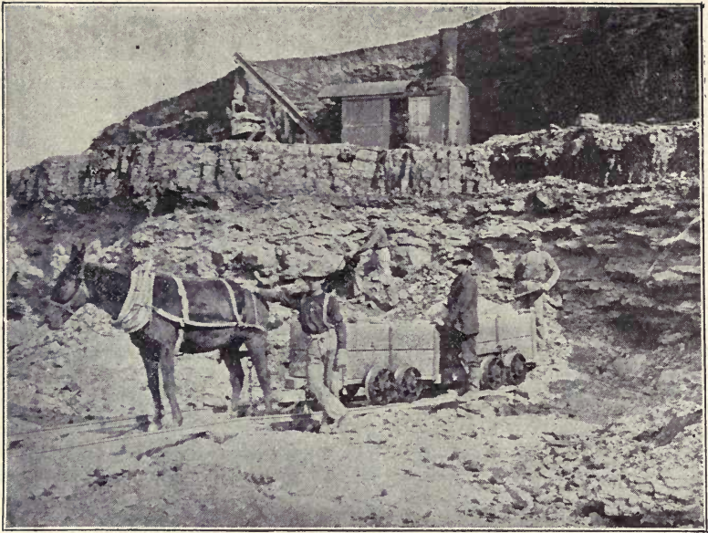
PLATE LXXXVIII, FIG. 1. — Section showing fire clay underlying coal seam. The upper clay above coal is of impure character.
