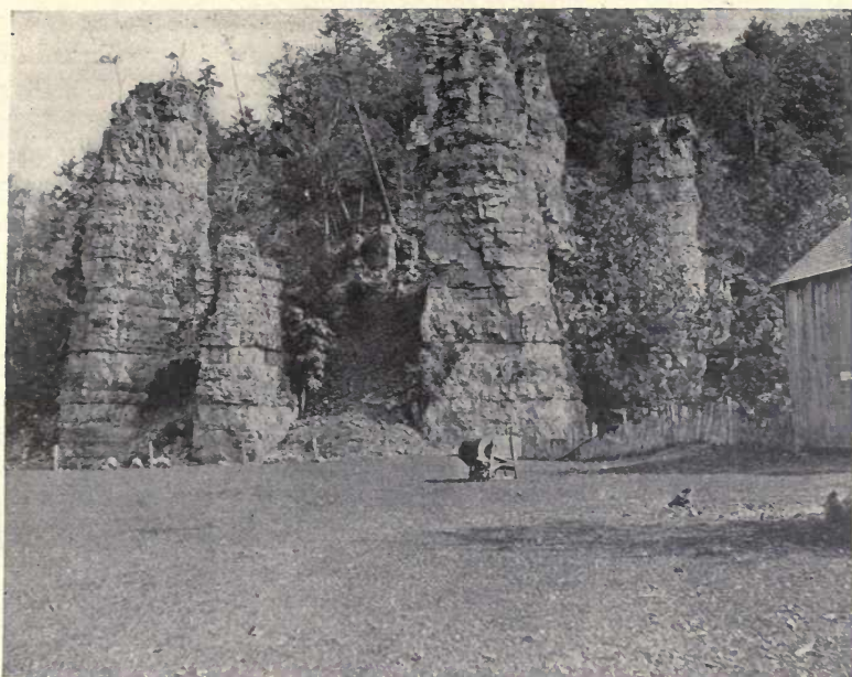
PLATE XXXVII, FIG. 1. — Limestone "chimneys," separated by hollows caused by solution along vertical joint planes. (T. L. Watson, photo.)
