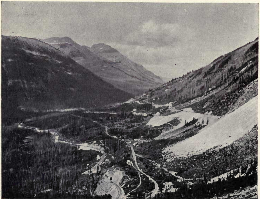
FIG. 2. — View from Mount Stephen, near Field, B. C., looking towards pass at Hector. On right slope are seen the two ends of the upper tunnel crossing fault zone in mountain on right. On extreme left, slope of Mt. Ogden, where the lower spiral tunnel is in massive limestone.
