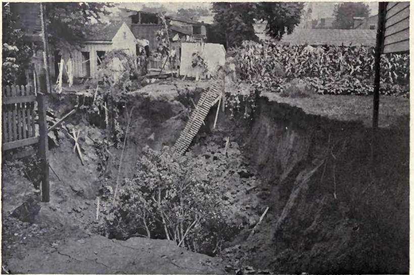
FIG. 2. — Large hole formed along line of caving, Staunton, Va.
