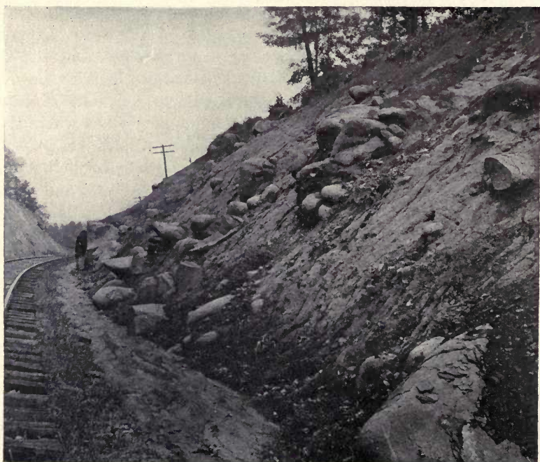
FIG. 2. — Diabase dike, Virginia. The weathering has broken the rock down to a mass of boulders. (T. L. Watson, photo.)
