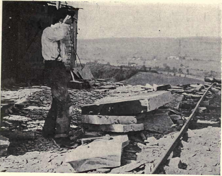
PLATE LXXXII, FIG. 1. — Sculpting slate. The slab has been broken along the grain, and as the one piece dropped, it broke along the cleavage. (H. Ries, photo.)
