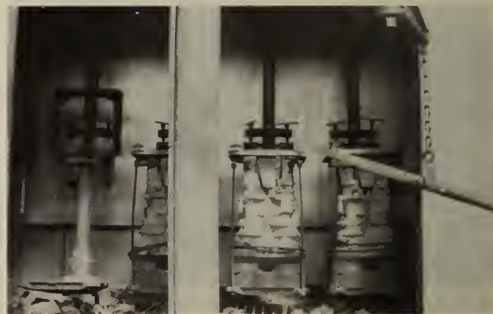
Fig. 7—Casting coming from smoke hood and vibrator ready to be removed for breakup
