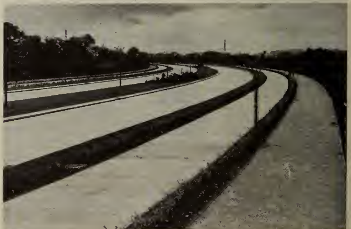
Fig. 4—Highway in the Borough of Derby, England. Note the division to provide for cyclists and pedestrian pathways
