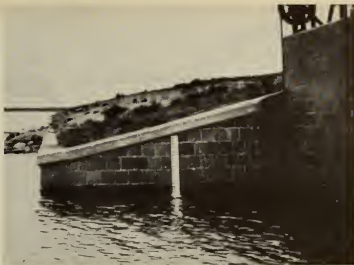
Fig. 5—Closer view of the tile facing on the reservoir outlet structure.
