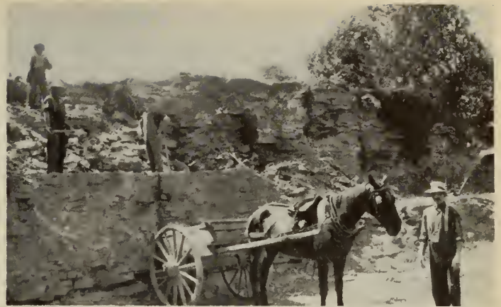
Fig. 5—Highway Work in Ontario, 1918. Operation of Quarry, Hamilton-Dundas Road
