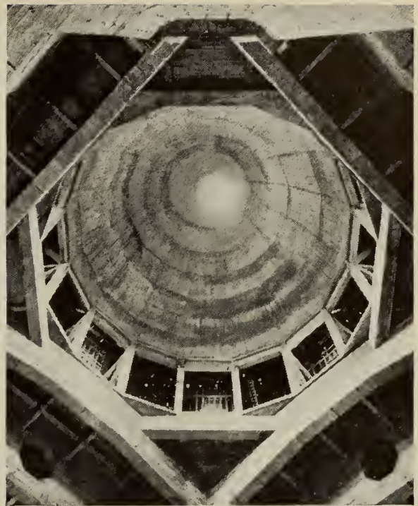
Fig. 9—Upper View from the Nave Floor Showing the Small Dome and Its Supports
