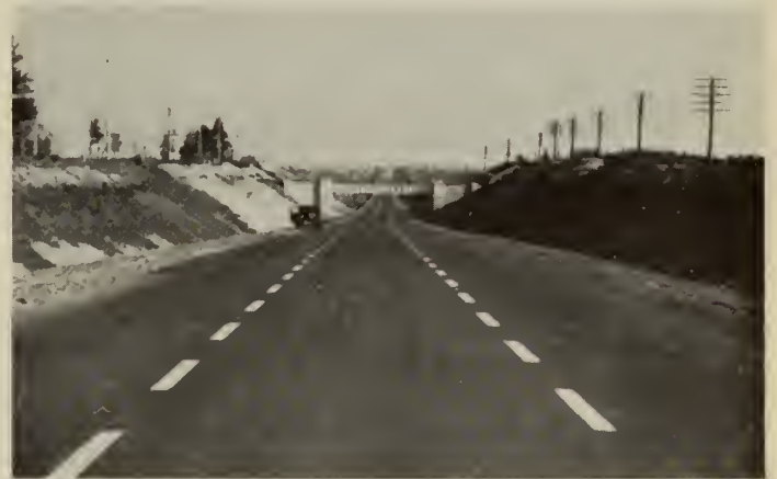
Fig. 2—Highway No. 11, between Pont Béclair and St. Jérôme, Que., showing well marked traffic lanes making for increased safety
