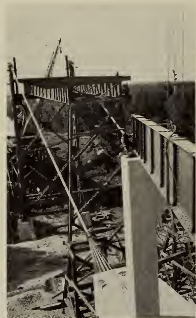
Fig. 6—Erection of North Approach Viaduct Suspension Span
