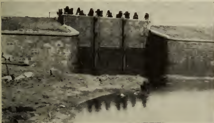
Fig. 4—Concrete outlet structure from a large reservoir repaired and faced with glazed tile in the fall of 1927.
