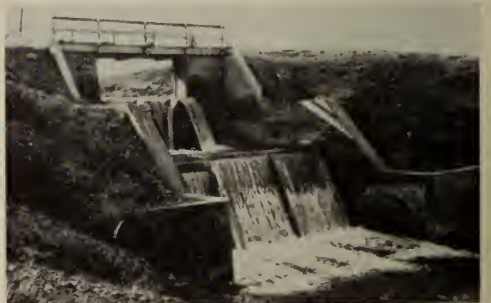
Fig. 3—View of the same drop taken about six years later. Discoloration caused by dried algae.
