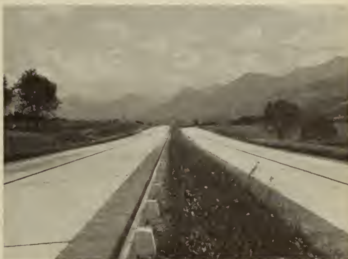
Fig. 5—Reichsautobahn, Munich-Salzburg, Germany. Limited highways not necessarily built at the same elevation
