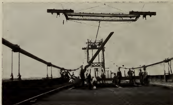
Fig. 10—Erecting I-Beam-Lok Flooring, Suspension Bridge
