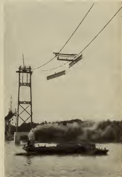
Fig. 9—Erection Second Girder, First Girder Connected, Suspension Bridge
