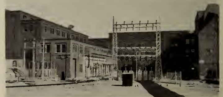
Fig. 6—General View of Substation at Baie Comeau
