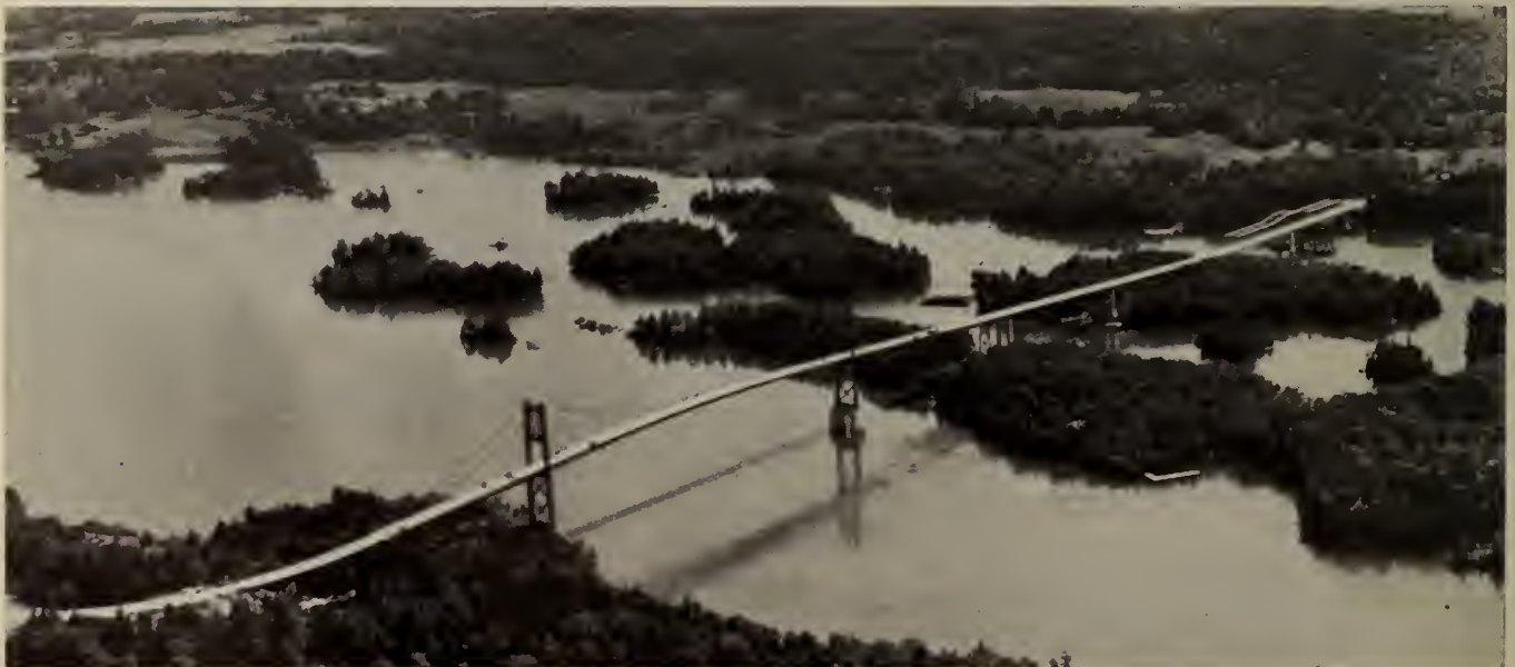
Fig. 1—Canadian Section of Thousand Islands Bridge (looking South), showing Canadian mainland in Foreground
