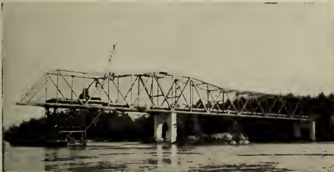
Fig. 3—Erection of North Span, Continuous Truss Bridge
