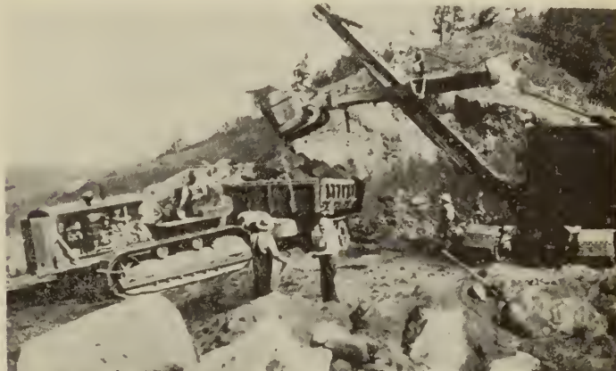
Fig. 9—Highway Work in Quebec, 1938. Caterpillar Tractors with 12-Yard Track Type Waggon Disposing of Boulders and Clay from 1\frac{1}{2} -Yard Shovel
