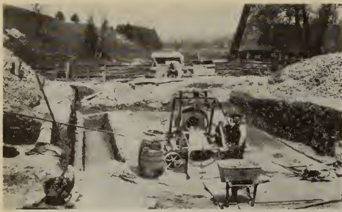
Fig. 7—Highway Work in Ontario, 1918. Concreting Bridge Abutment
