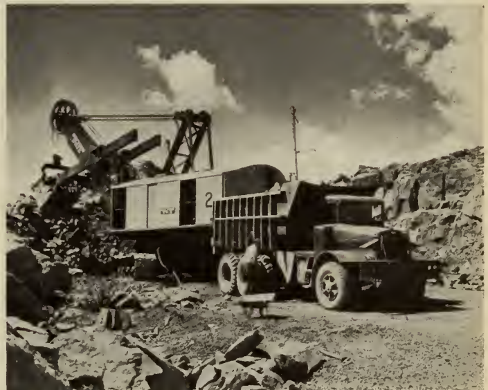
Fig. 1—Truck and shovel operating at Frood mine where surface, or open pit, mining obtains average grade of ore by combining surface and underground ore
