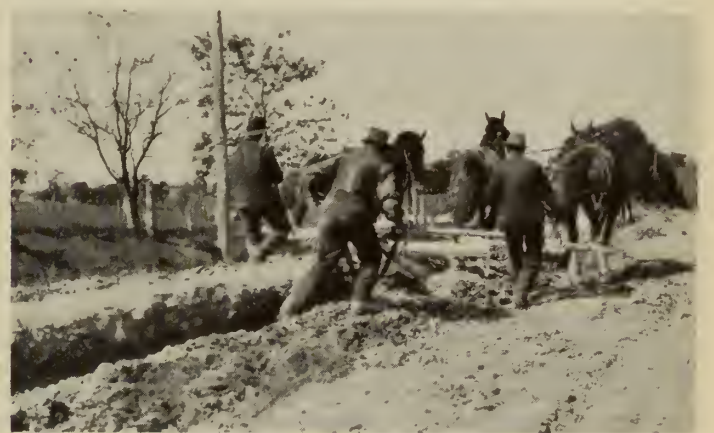
Fig. 6—Highway Work in Ontario, 1918. Ditching Operations
