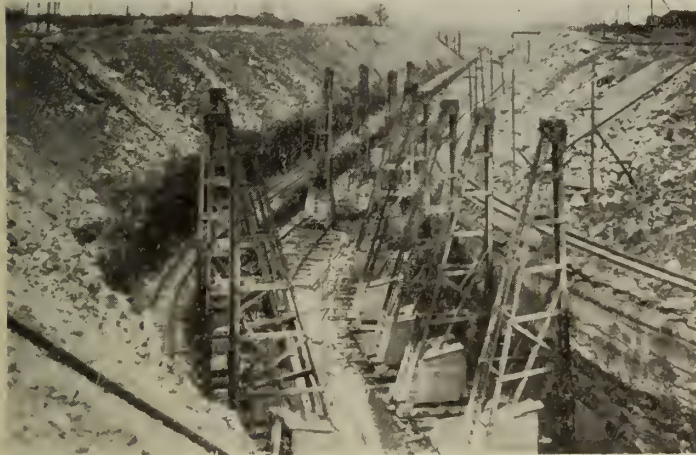
Fig. 1—Queenston-Chippewa development, 1918 to 1922. Battery of Drills working in Rock Cut
