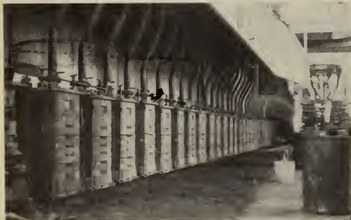
Fig. 6—Completed mould mounted on pouring reel
