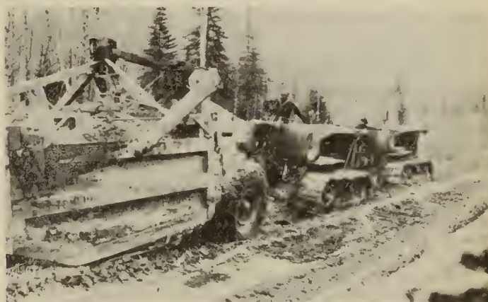
Fig. 10—Highway Work in Ontario, 1938. Grading with Carryall
