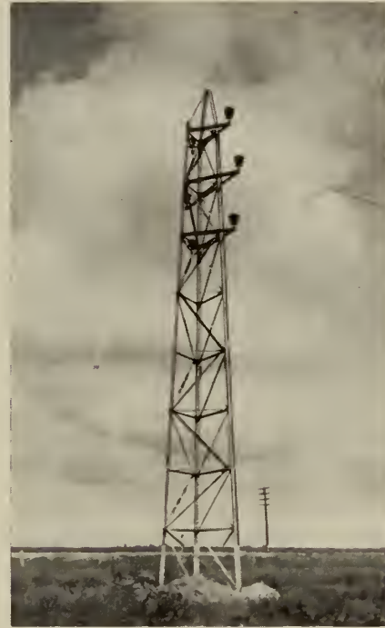
Fig. 5—Double circuit 66 kv. three legged tower
