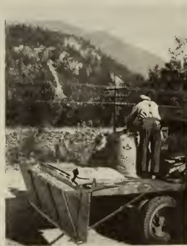
Fig. 6—Method used for spreading calcium chloride.
