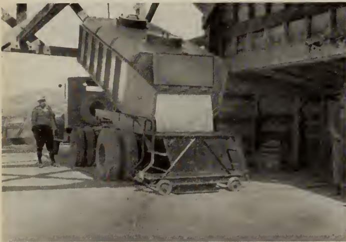
Fig. 3—Rapide Blanc Development, 1931 to 1934. Unloading cement from special semi-trailer truck into bin at mixer plant
