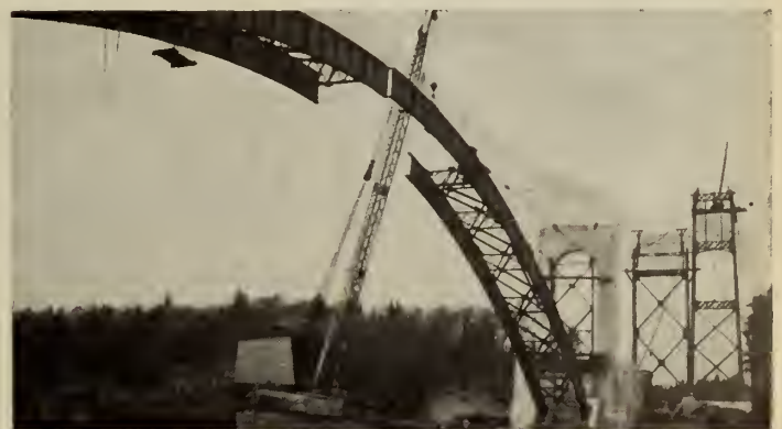
Fig. 4—Erection of Arch Ribs
