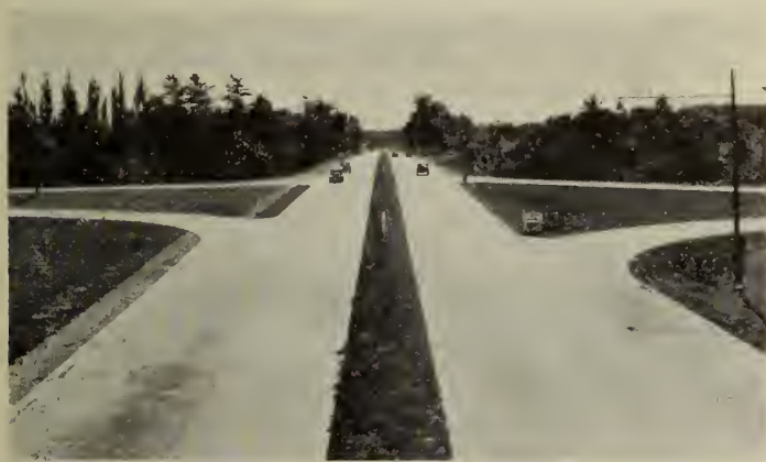
Fig. 1—The Queen Elizabeth Way between Toronto and Fort Erie, Ontario. Note widened traffic way to permit of traffic leaving the highway
