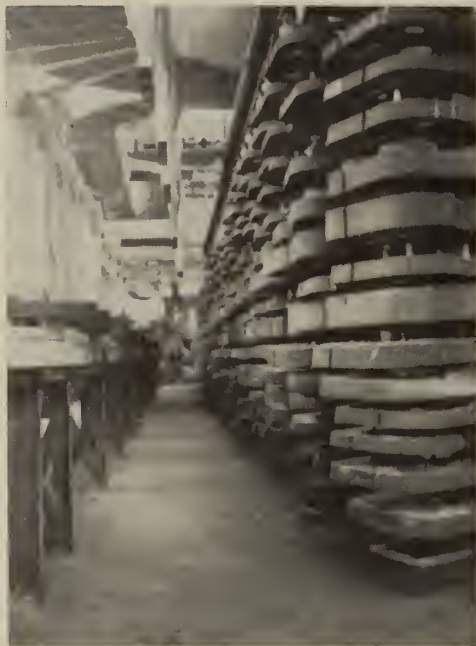
Fig. 5—Finishing conveyor (left), storage reel (right)
