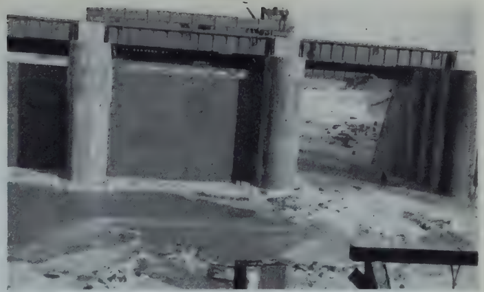
Piers and gates of South dam at Ile Juliet.
