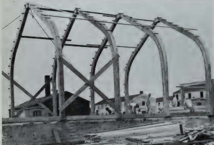
Fig. 2—Laminated arches provide a simple but sturdy frame for an army camp chapel.
