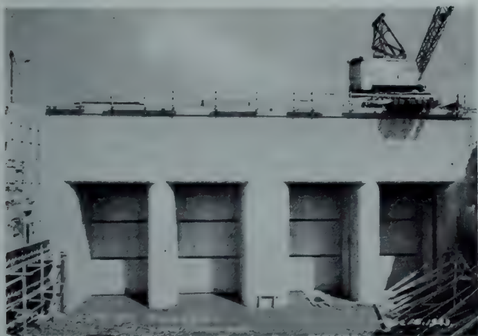
Fig. 6—Photograph of headworks nearing completion.
