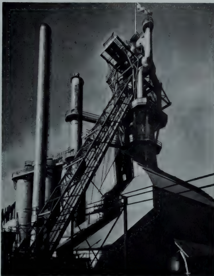
Canada's largest blast furnace. This stack has a daily capacity of 980 net tons of pig iron.
