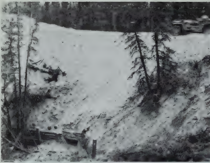
A heavy fill over a deep culvert.
