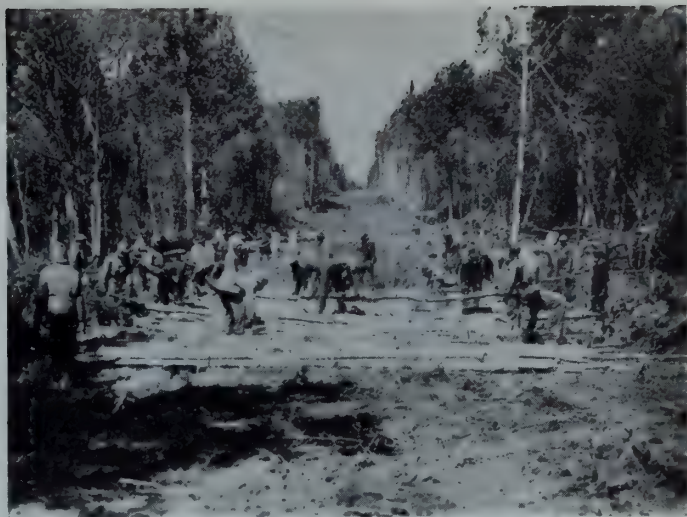
Crew engaged in ditching and corduroying.
