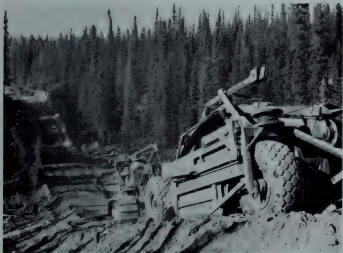
Carry-all moving earth to a fill.
