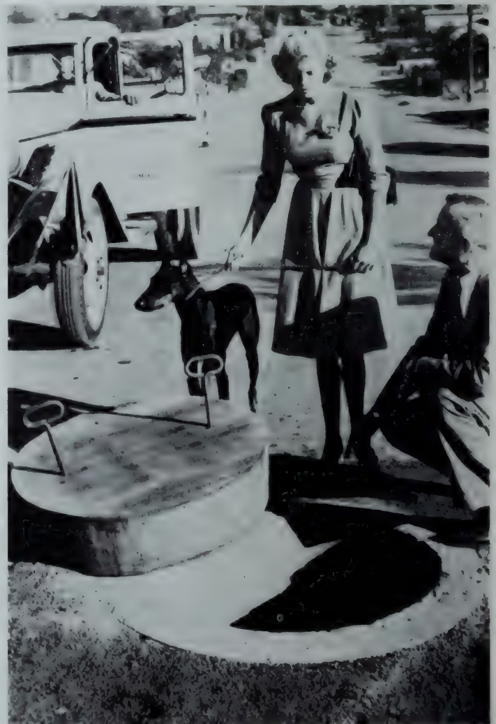
Alfred Jones, Los Angeles County Surveyor, explains the wooden manhole installation to Miss Beverly Hoyt.
