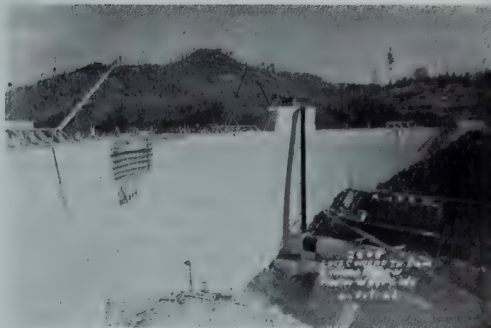
Fig. 6—General view looking east, showing connection to penstock. October, 1941, completed.
