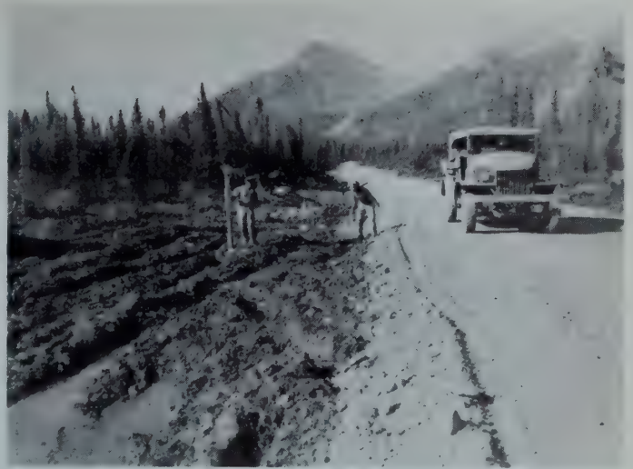
Completed road 40 miles east of Teslin.
