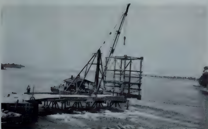
Placing steel crib in the south channel at Ile Juliet.
