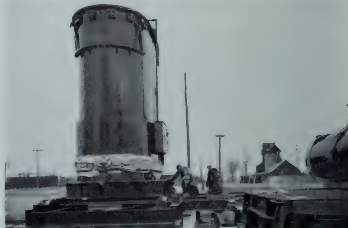
Fig. 3—Transformer on transfer truck.
