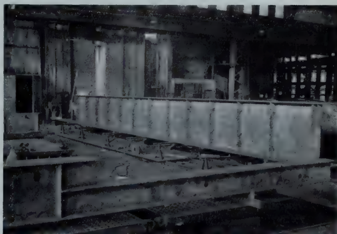
Fig. 1—Girders and columns for mill buildings fabricated by welding rolled plates.
