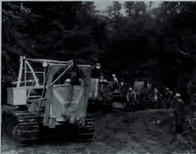
The latest method of providing storm-proof long distance telephone facilities is by burying cable directly in the ground by means of special plough drawn by powerful tractors. This type of cable is being laid in 1943 to link Ottawa, Montreal and Toronto.
