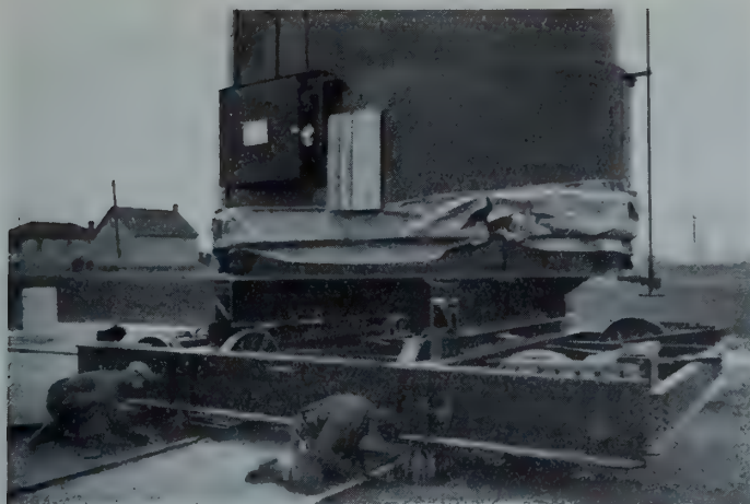
Fig. 4—Changing wheels on transformer truck.
