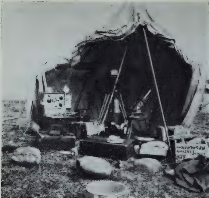
Equipment for obtaining astronomic observations; radio set on the left; prismatic astrolabe at right centre on stool.
