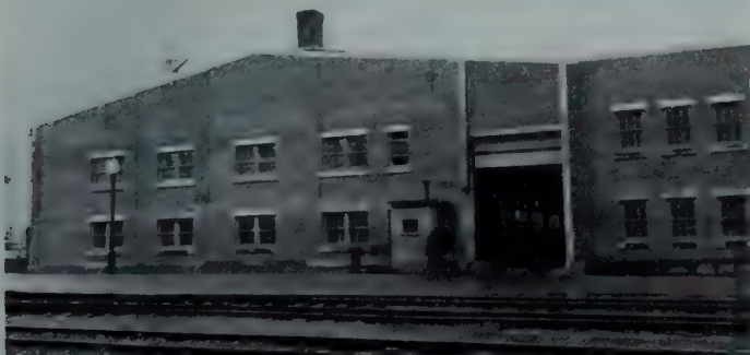
Fig. 5—West end of shed 8 showing vertically sliding door at entrance from Union St.
