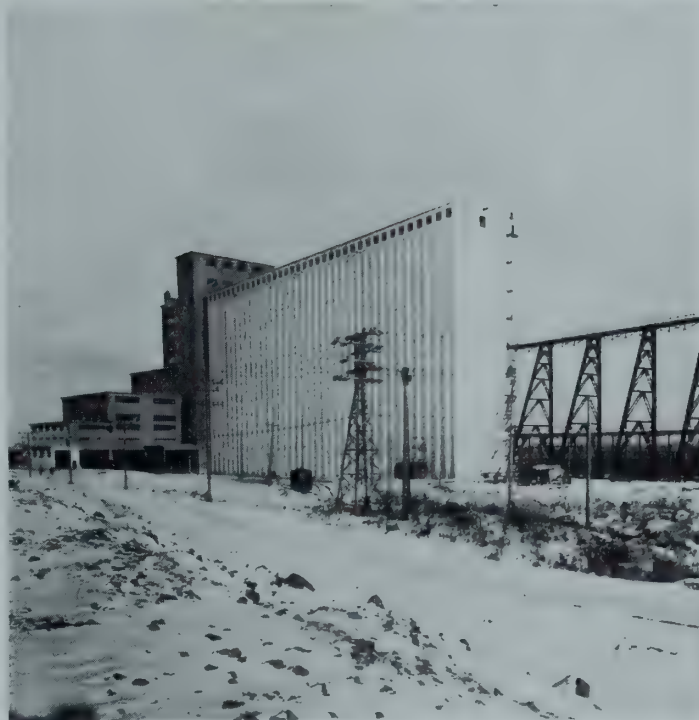
Grain storage elevators and flour mill on the Welland Canal, near Port Colborne, Ont.
