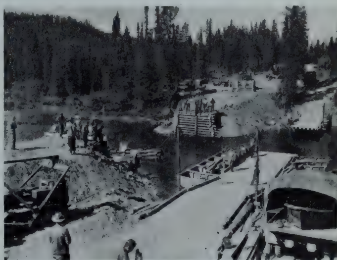
Building a bridge over Morley River.
