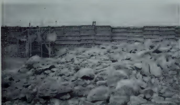
Steel crib cofferdam unwatered, showing typical river bottom.
