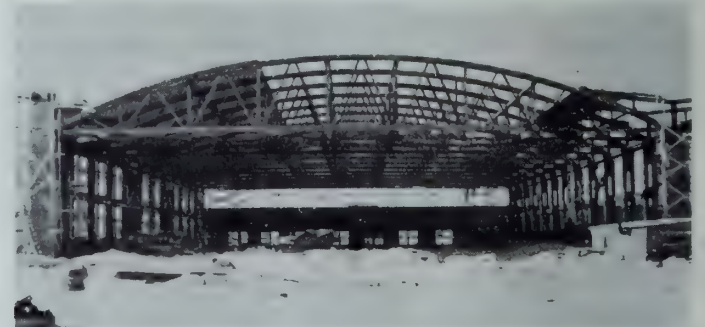
Fig. 18—View of 134 ft. clear span hangars at an airport in Eastern Canada. These have the longest span timber roof trusses in Canada.
