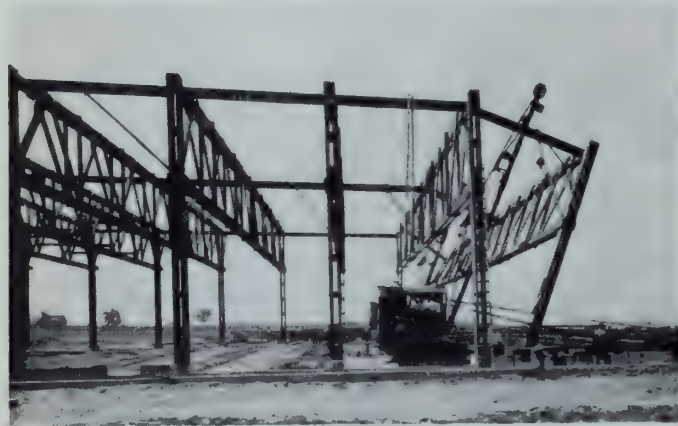
Fig. 18—View of 134 ft. clear span hangars at an airport in Eastern Canada. These have the longest span timber roof trusses in Canada.
