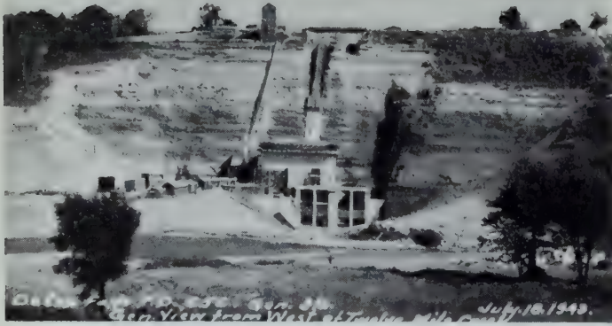
Fig. 8—Photograph of penstock and power house.
