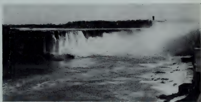
Goat Island flank of Horseshoe falls from Canadian side. (Above) November 26, 1925, discharge over Horseshoe, 106,000 cu. ft. per sec. (Below) April 30, 1913, discharge 198,000 cu. ft. per sec.
