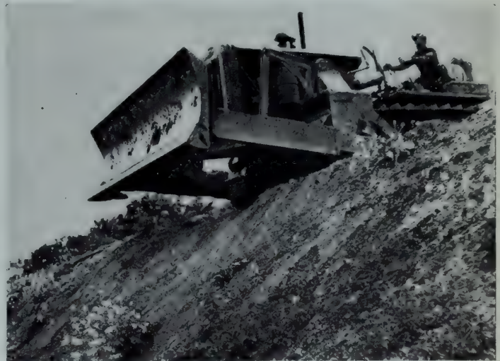
A bull-dozer tractor, levelling out rough ground.
