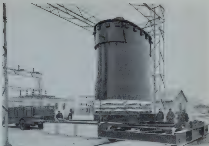
Fig. 5—Pulling transformer onto its foundation.
