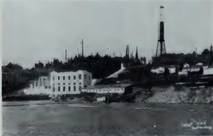
Fig. 1—Power house and surge tank at Scow Bay.
