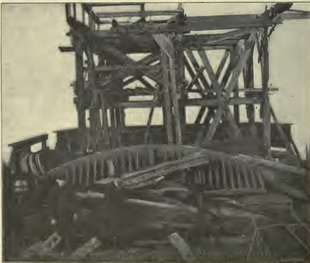
SADDLES AND WRECKED FALSEWORK ON NORTH SIDE OF TOWER.
