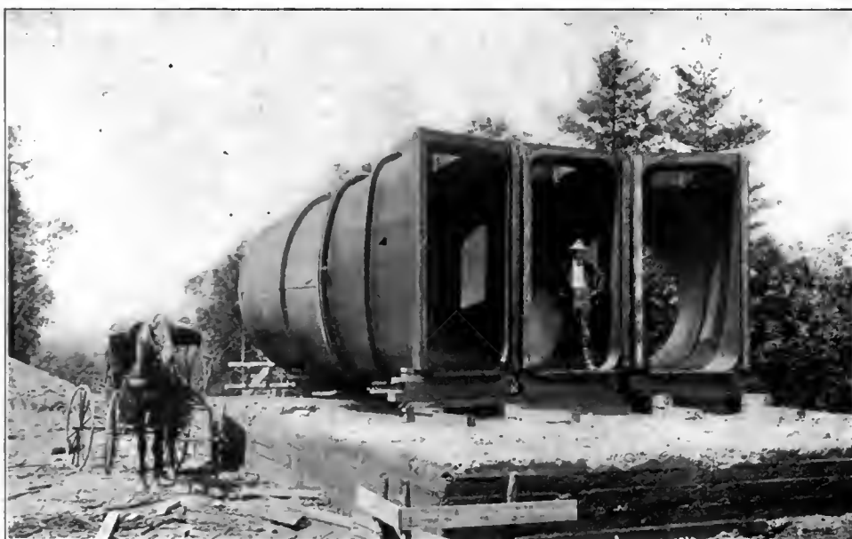
CASTINGS AT SIPHON CHAMBER FOR CONNECTING WITH STEEL PIPES.
