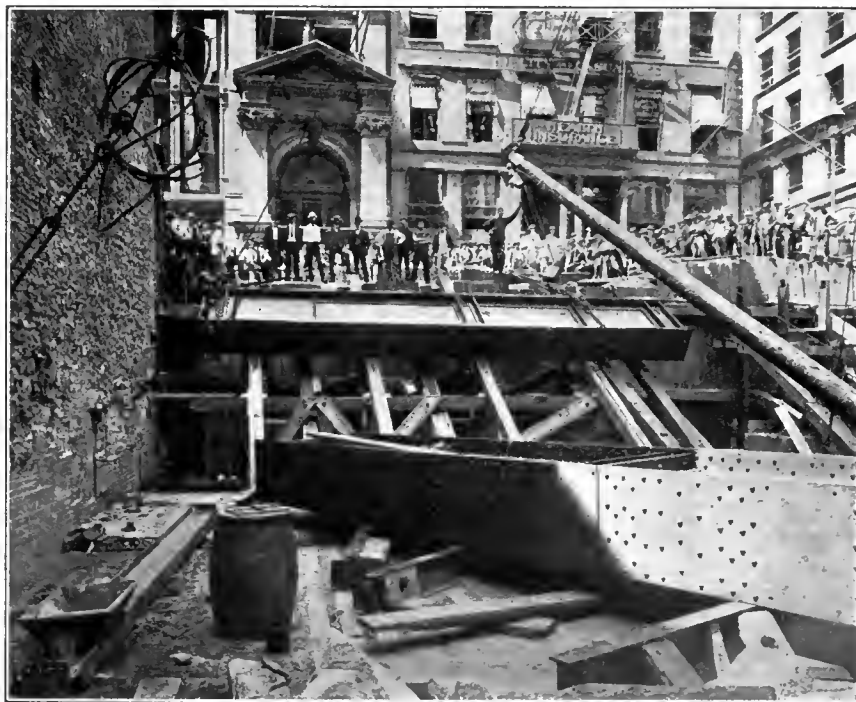
METHOD OF LOWERING A HEAVY FOUNDATION GIRDER.
