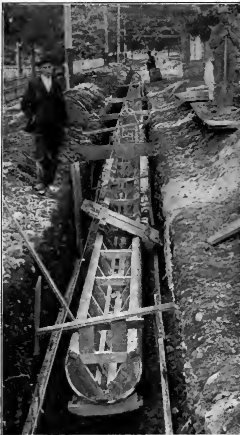
THE CENTERING IN PLACE.
