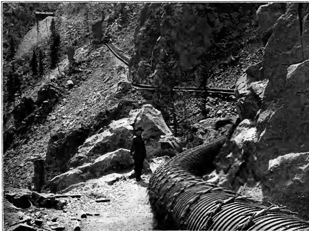
THIRTY-INCH WOOD STAVE PIPE, 23,000 FEET LONG.
