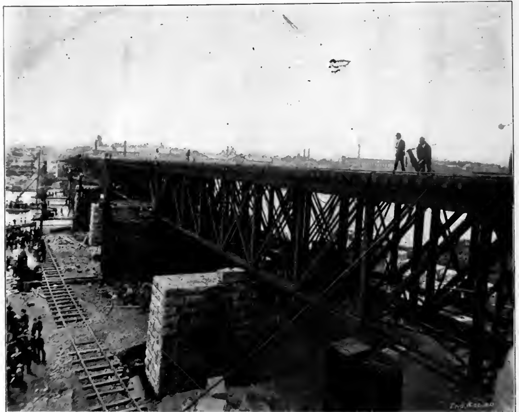
MOVING THE PENNSYLVANIA RAILROAD BRIDGE AT NEW BRUNSWICK.
