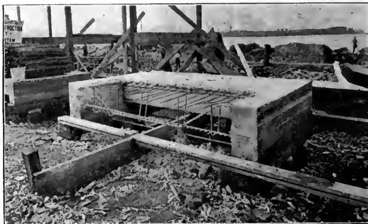
CONSTRUCTION OF TEST SLAB.
