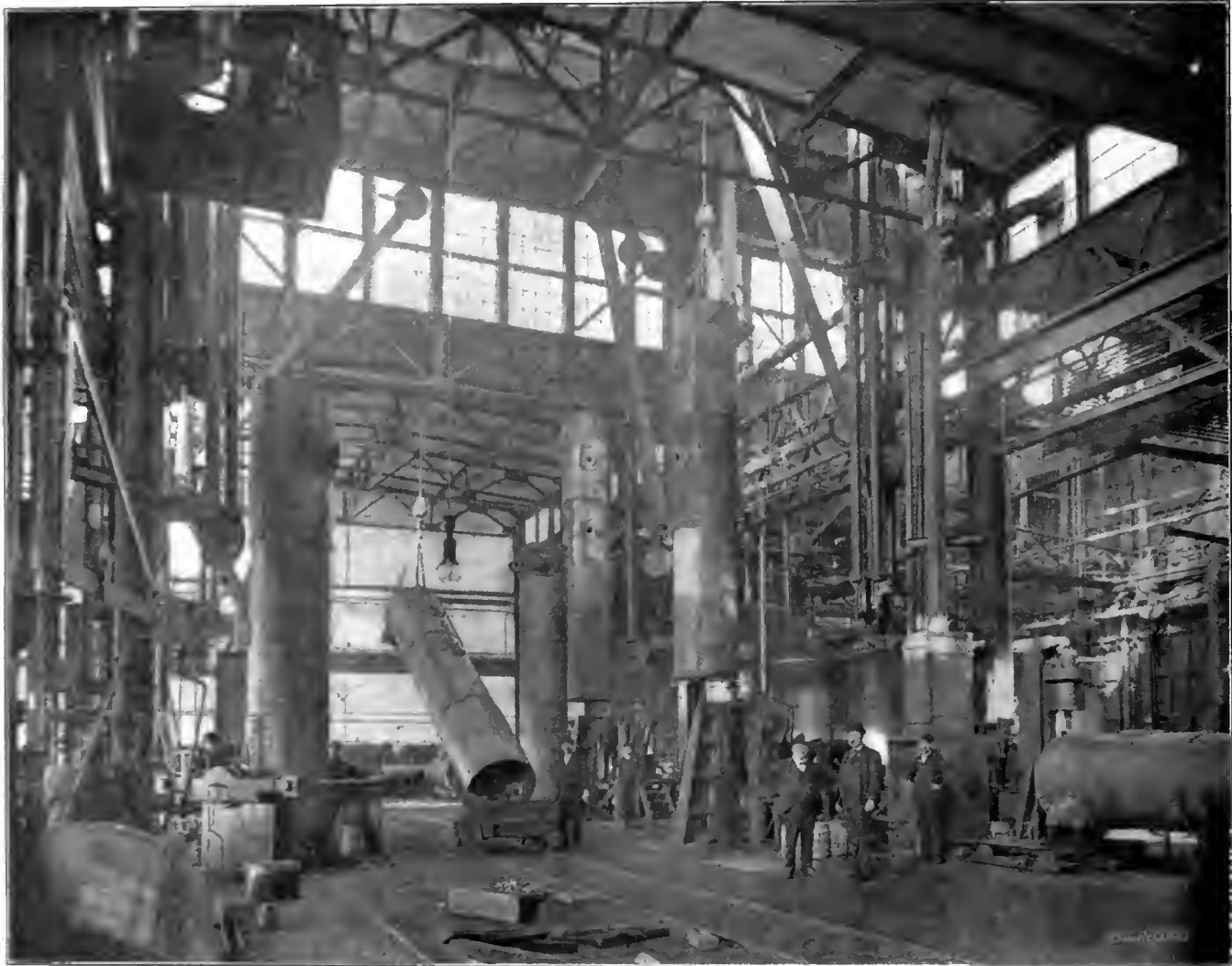
VIEW OF RIVETING TOWER.
