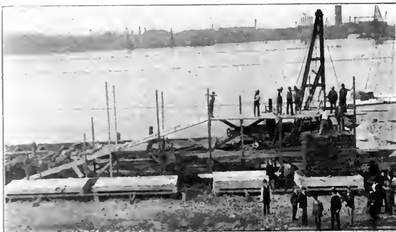
LOADING TEST SLAB.
