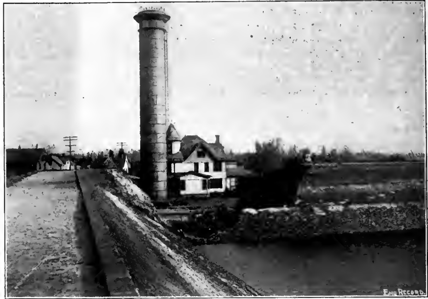
VIEW OF BREAK FROM INSIDE THE RESERVOIR.
