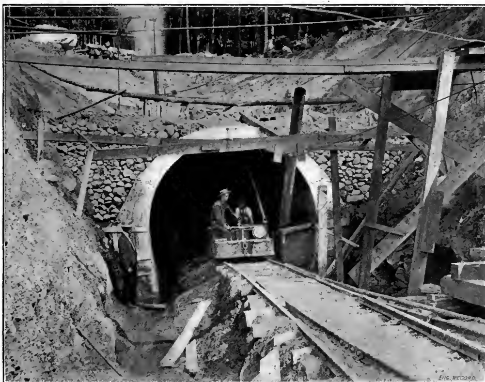
WEST PORTAL OF TUNNEL NO. 4 SHOWING CROSS-SECTION OF CONCRETE LINING.
