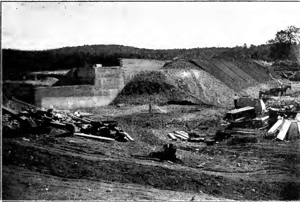
DOWN-STREAM FACE OF DAM AT EFFLUENT CHAMBER.
