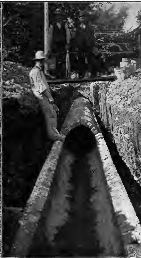
THE COMPLETED INVERT.
