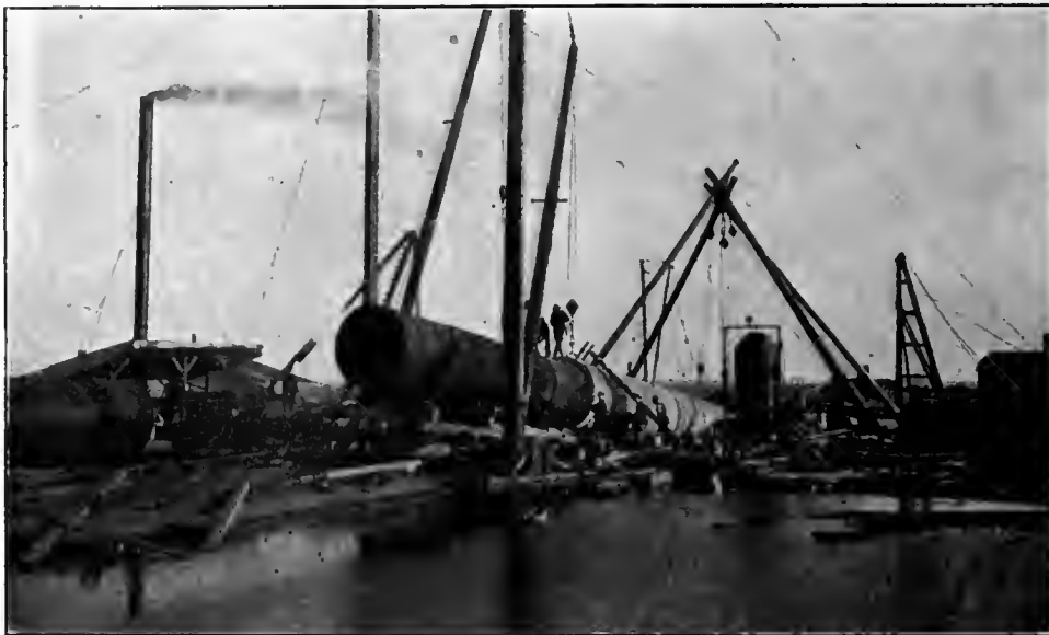
ASSEMBLING AND LAUNCHING PIPE.
