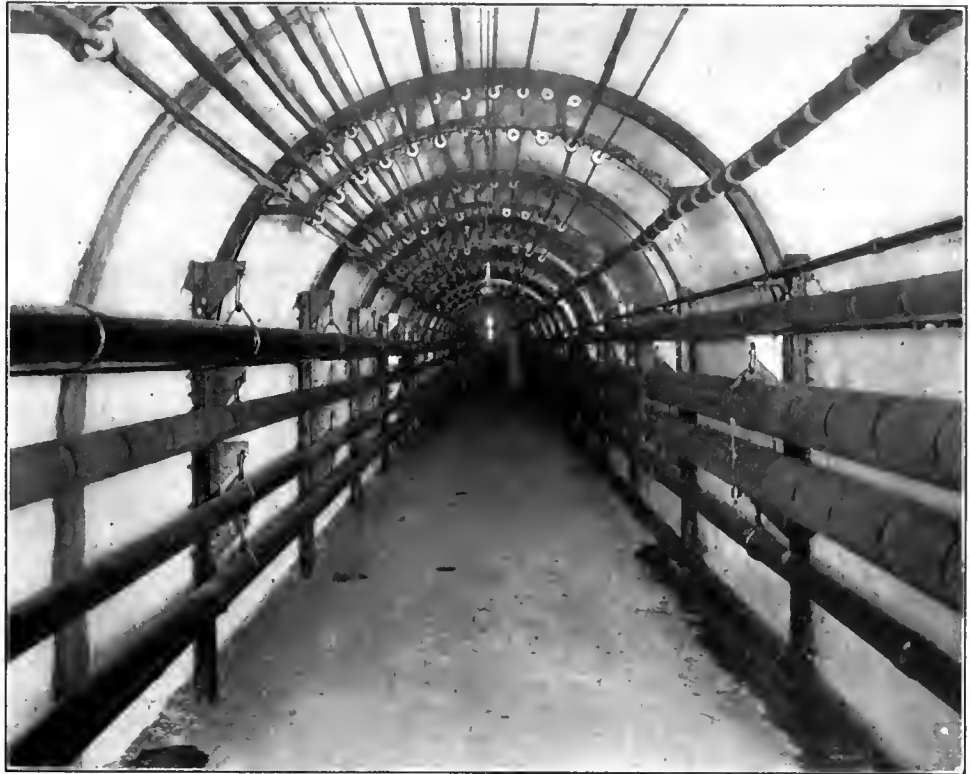
TUNNEL CONNECTING POWER STATION AND HEADHOUSE.
