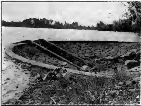
CIRCULAR DAM, LAKE COCHITUATE.
