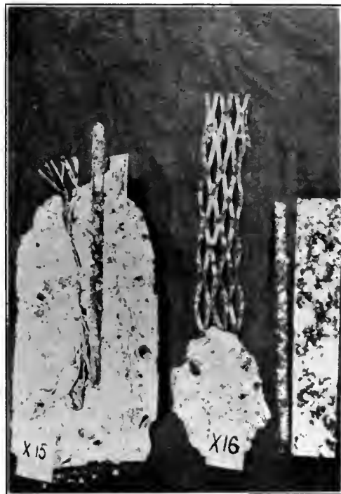
STEEL RUSTED BY CONTACT WITH CINDERS.
