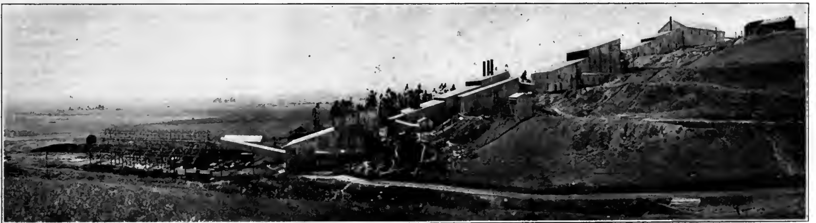
THE WORKS OF THE PACIFIC PORTLAND CEMENT CO., SUISUN, CAL.
