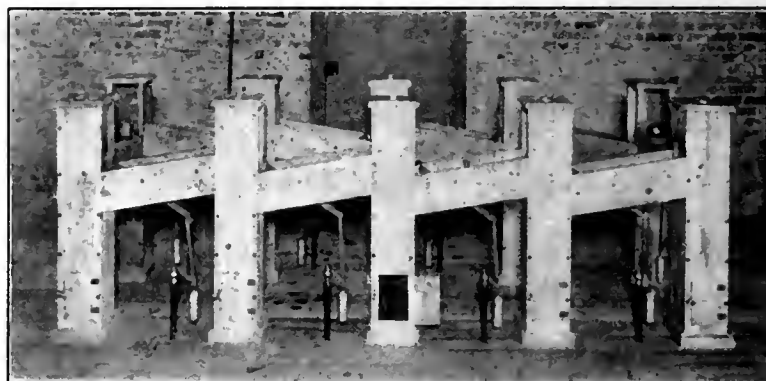
AUTOMATIC CONTROLLING DEVICE, SEWAGE PURIFICATION PLANT, LAKE FOREST, ILL.
