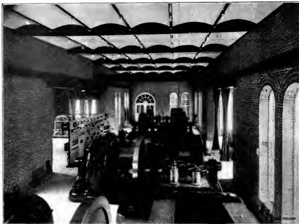
INTERIOR VIEW OF STATION A.
