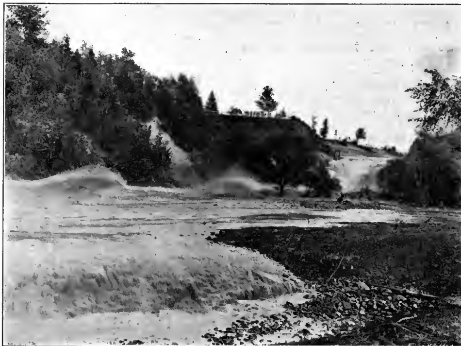
BREAK IN RESERVOIR BEFORE COMPLETION OF WASHOUT.
