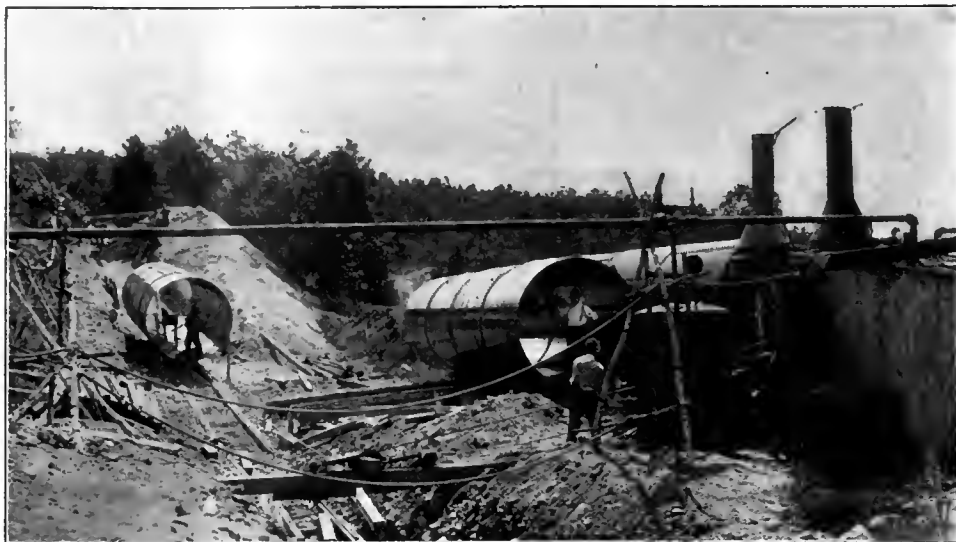
PLANT FOR LAYING STEEL PIPES, HAPPY HOLLOW SIPHON.
