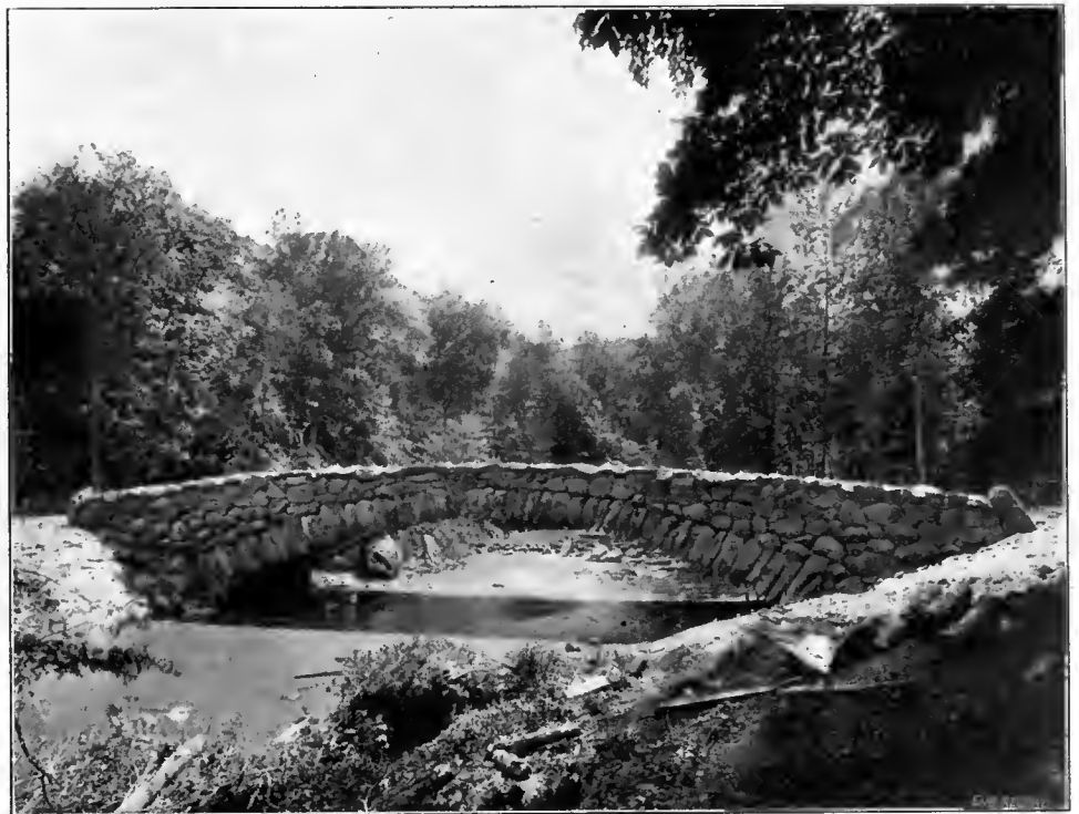
A CONCRETE-STEEL BRIDGE OVER ROCK CREEK, WASHINGTON, D. C.
