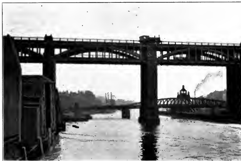
THE HIGH-LEVEL BRIDGE, NEWCASTLE.
