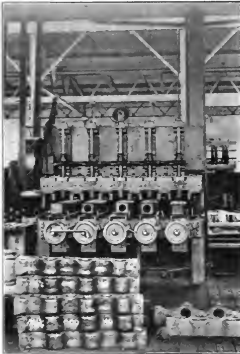
MULTIPLE TOOL FOR BORING HEADERS.
