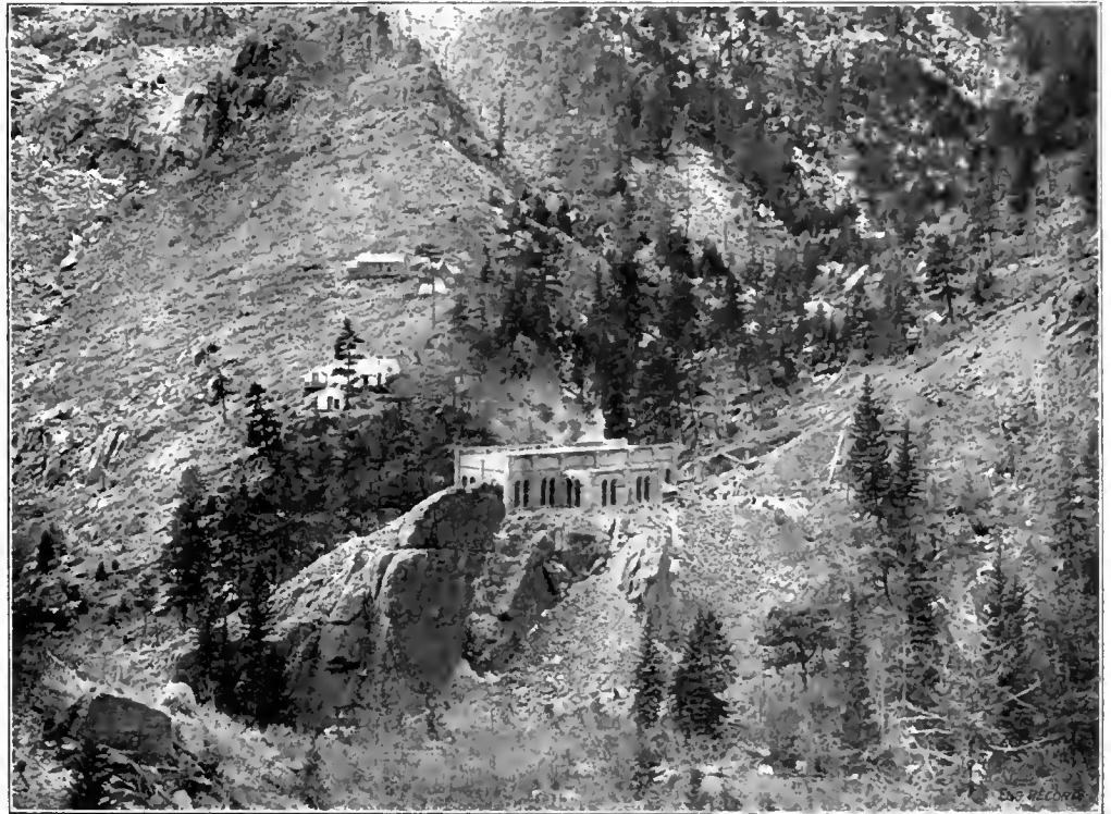
POWER STATION A, PIKE'S PEAK POWER COMPANY.
