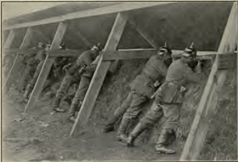
FIG. 35.—Rifle trench with overhead cover of steel plates supported on frame-work.
