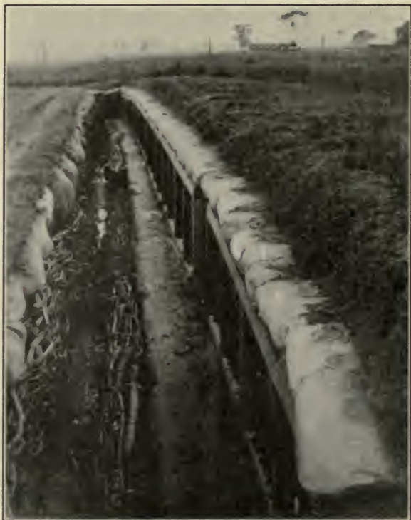
FIG. 30.—Simple rifle trench with sand-bag and hurdle revetment and splinter-proof shelters under parapet.
