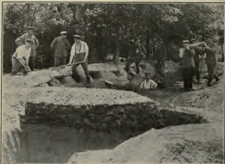
FIG. 32.—Rifle trench with head cover (loopholes) and traverses.
