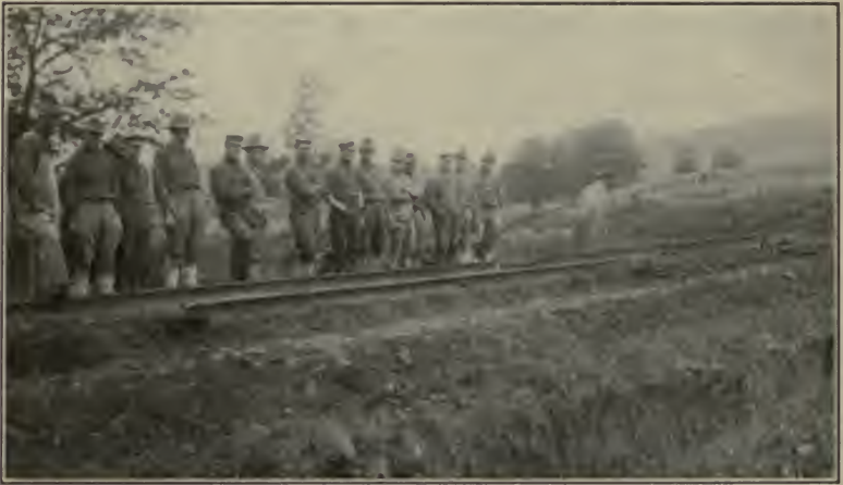
FIG. 54.—Railroad track cut by dynamite.
