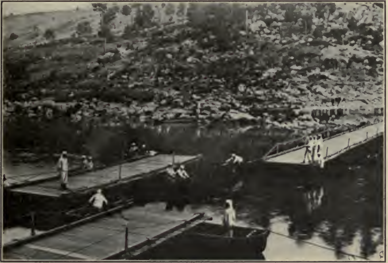
FIG. 13.—Draw span in ponton bridge. (Spanish ponton equipage.)
