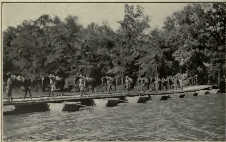
FIG. 12.—Completed bridge of light (canvas) equipage.
