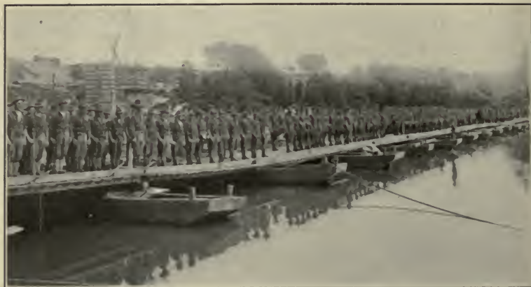
FIG. 11.—Completed bridge of heavy equipage. Note saddle in first boat.
