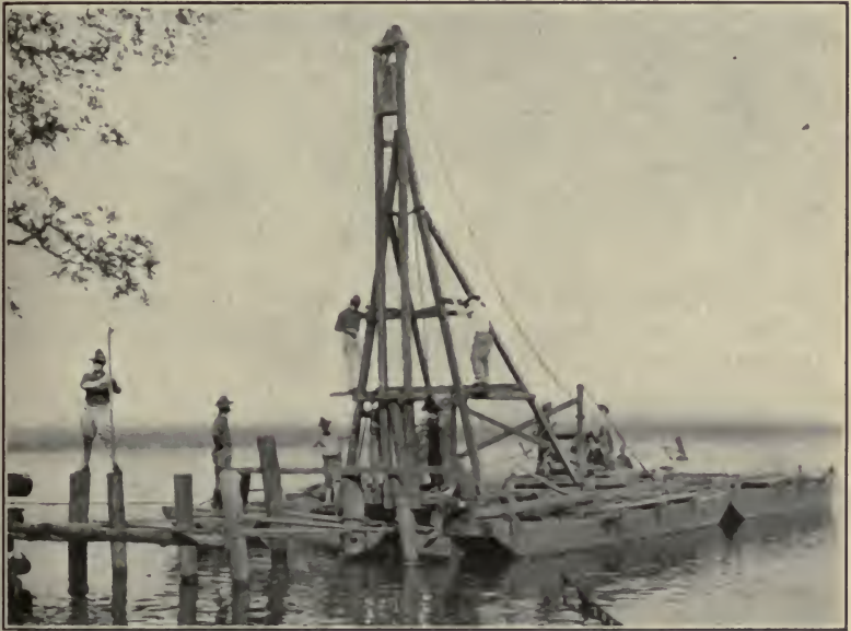
FIG. 15.—Driving piles with portable driver. The float is of ponton equipment, and the hoist is operated by a gasoline engine.
