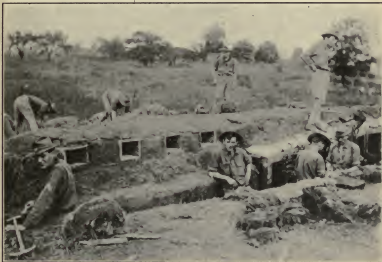
FIG. 33.—Rifle trench with plank loopholes and shelters under parapet. The latter is being covered with sod for concealment.
