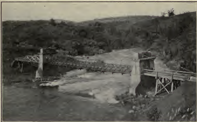
FIG. 23.—A Spanish suspension bridge in the Philippine Islands rebuilt for military use. Only the towers of the old bridge remained.
