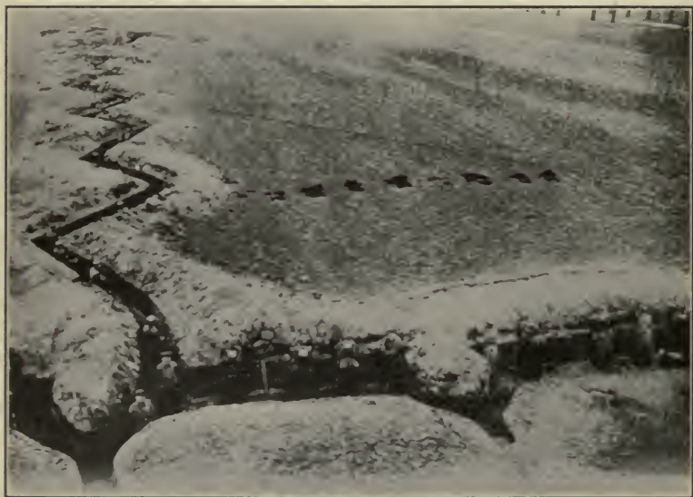
FIG. 40.—Second line of defense showing simple traversed trench and communicating trench zig-zag to front.
