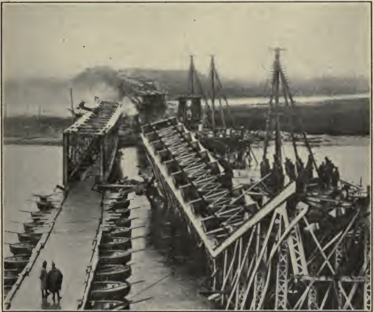
FIG. 53.—Ponton equipage used to replace ruined bridge span. (German ponton equipage.)
