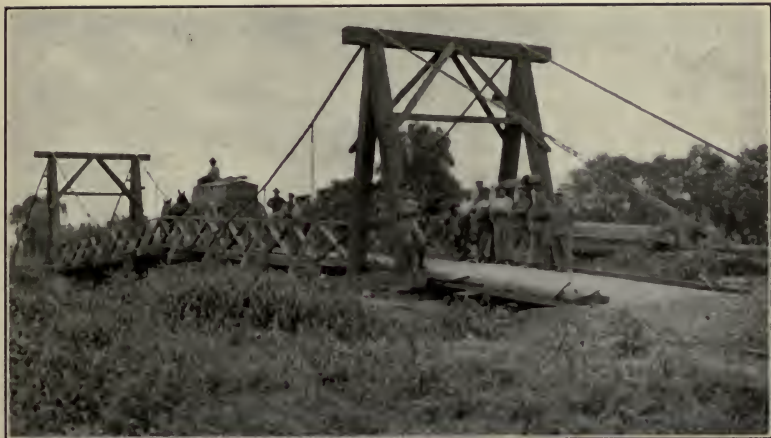
FIG. 22.—Field suspension bridge, roadway of ponton material. The wagon is the standard engineer tool wagon.
