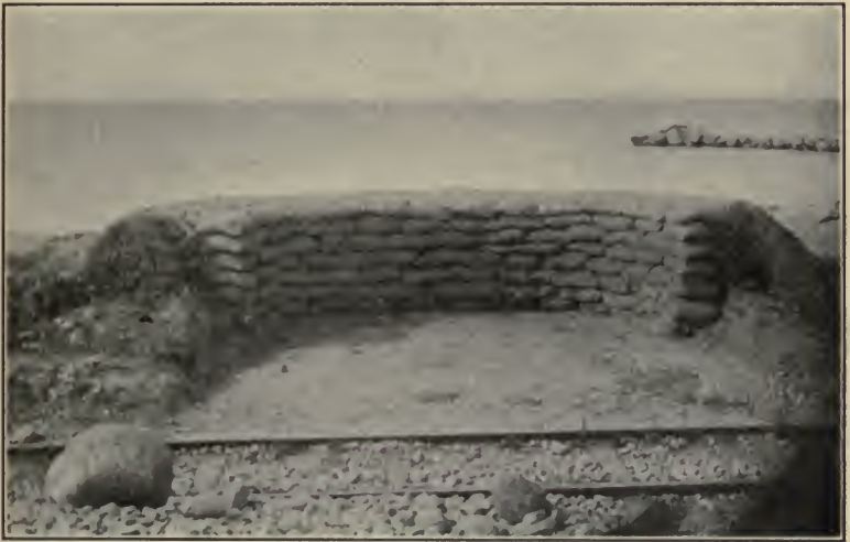
FIG. 49.—Emplacement for machine or field gun.
