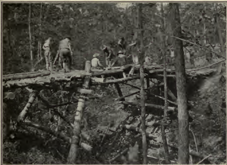
FIG. 20.—Double lock spar bridge.
