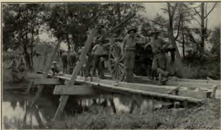
FIG. 5.—Portable trestle bridge of regular equipage. Note abutment sill, balk and side-rail lashings. This bridge can be constructed in a few minutes. It will carry the heaviest loads which accompany the army.
