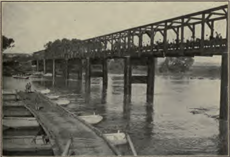
FIG. 17.—Truss bridge constructed in field by engineer troops. The spans are 90 ft. and the roadway 16 ft.
