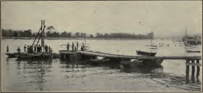
FIG. 24.—Landing wharf and pile driver of ponton material.
