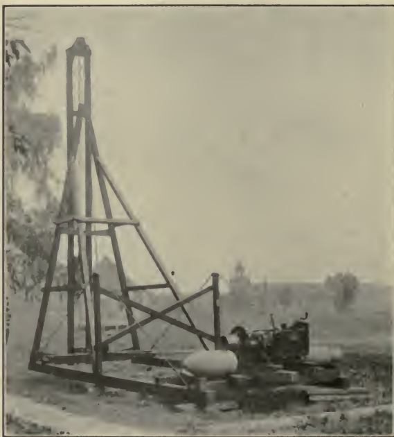
FIG. 16.—Portable pile driver with swinging leads and gasoline hoist.
