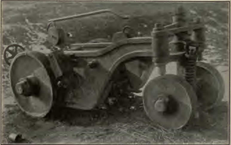
FIG. 56.—Machine employed by the Russians for tearing up roads.
