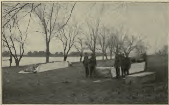
FIG. 8.—Assembling the canvas ponton.
