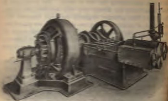
110 Horse-power Cross Compound Engine Directly Connected to 75 Kilowatt Dynamo.
