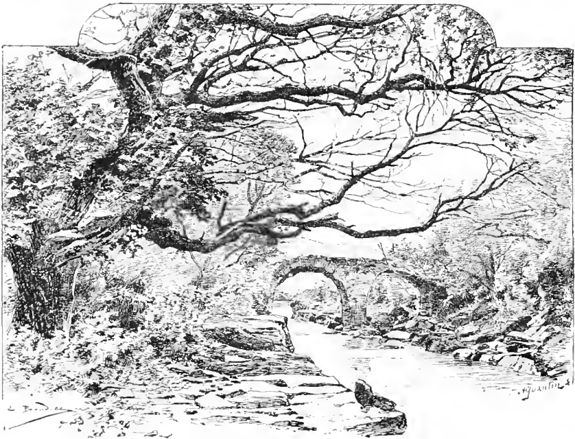
OLD BRIDGE AT KILLARNEY.
