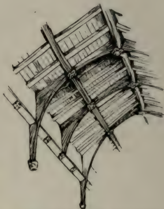
FIG. 71. ROOF WITH ARCHED PRINCIPALS, NORTH ELMHAM
