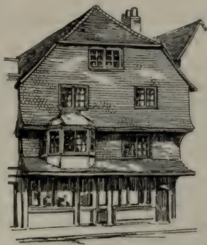
FIG. 176. WEATHER-TILING, HOUSE IN SALISBURY
